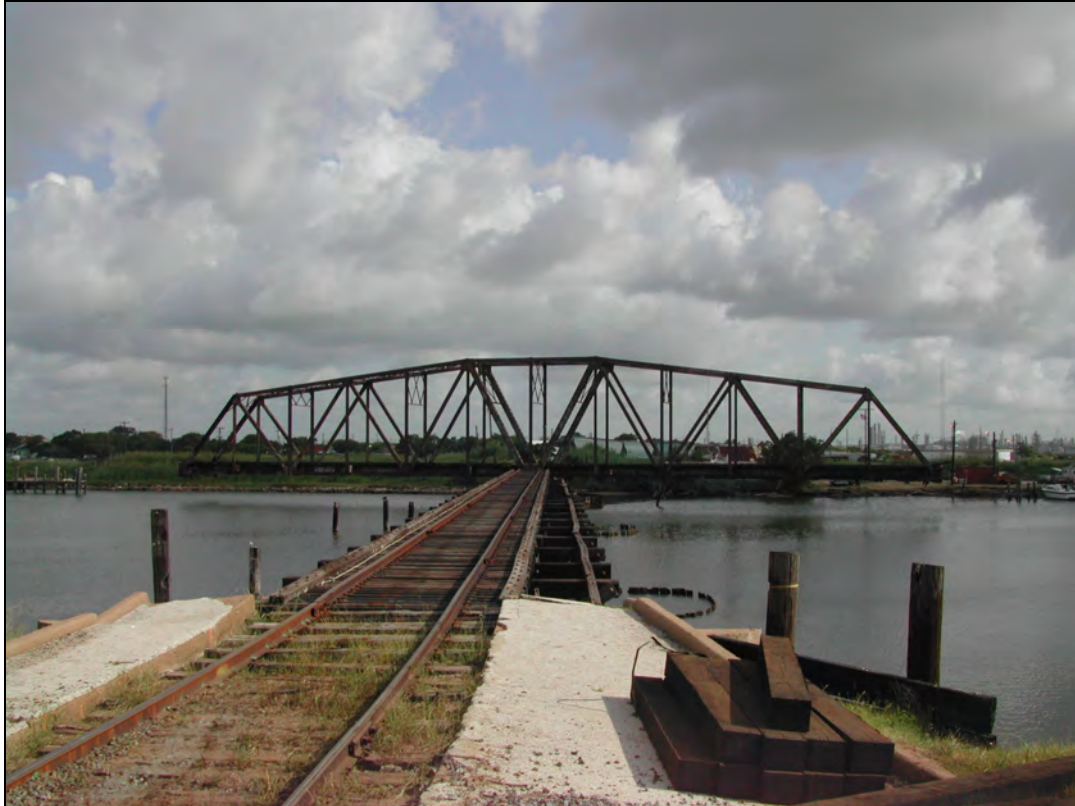
Figure 4.2 Swing Bridge on Rail Line Serving the Port of Freeport
