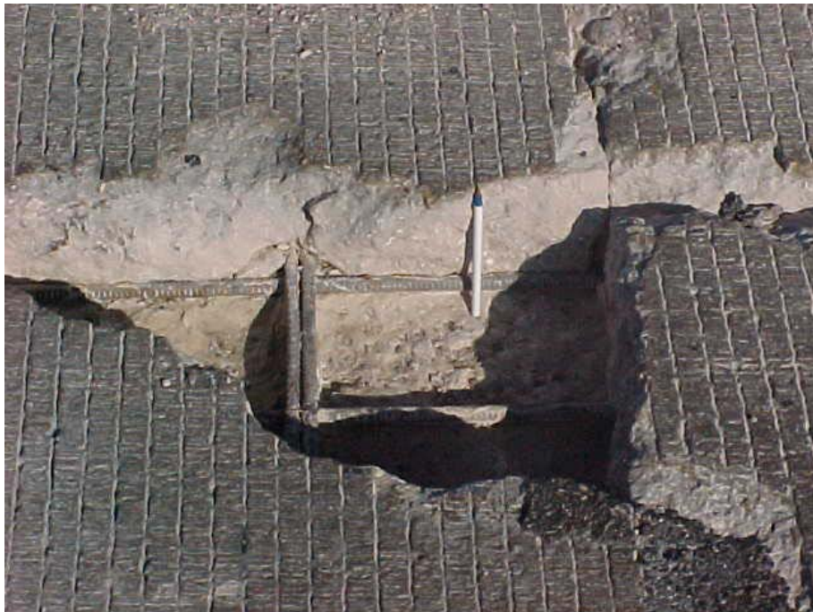
Figure 10.3 BCO deterioration
