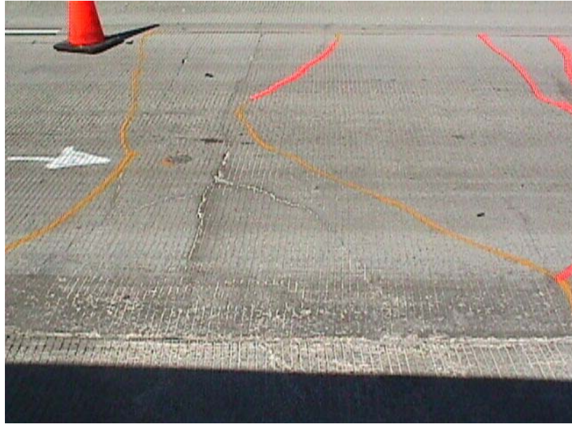
Figure 8.23 Delamination across the lane, where a core sample was extracted
