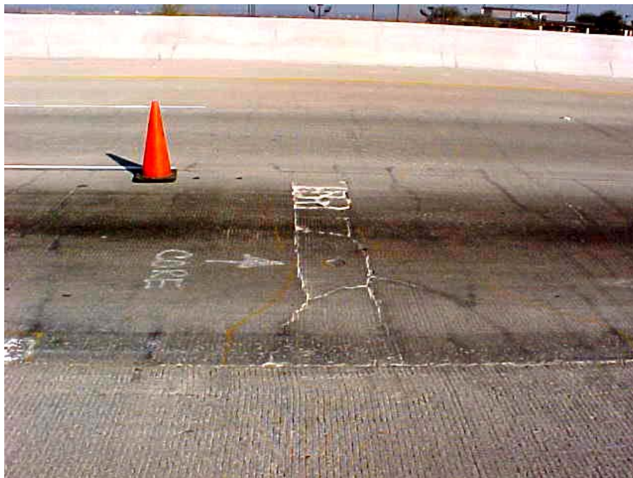
Figure 10.1 BCO delaminations on February 23, 1999
