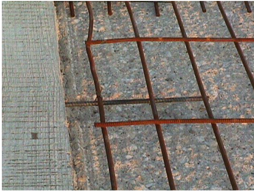
Figure 6.6 Tie-bar, from hardened pavement to new pavement
