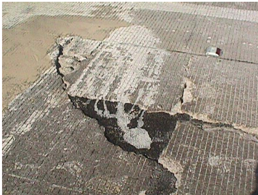
Figure 10.4 BCO deterioration
