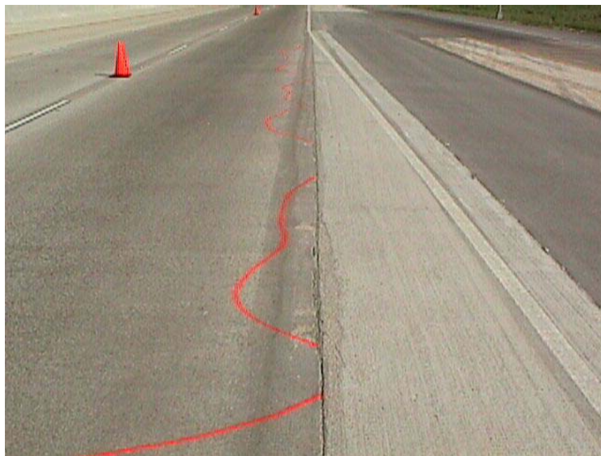
Figure 7.12 Common delamination pattern delineated with spray paint
