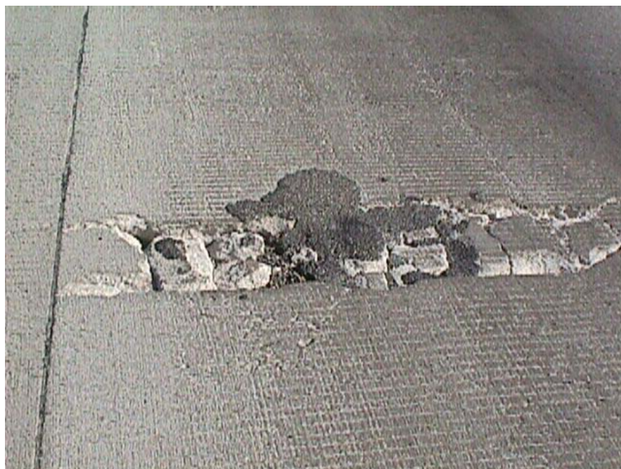
Figure 10.5 BCO deterioration
