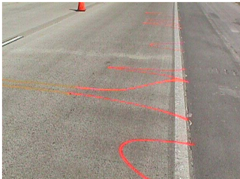
Figure 8.24 Extensive delamination starting at the edges and spreading toward the center of the lane
