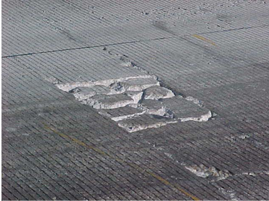
Figure 10.2 BCO deterioration
