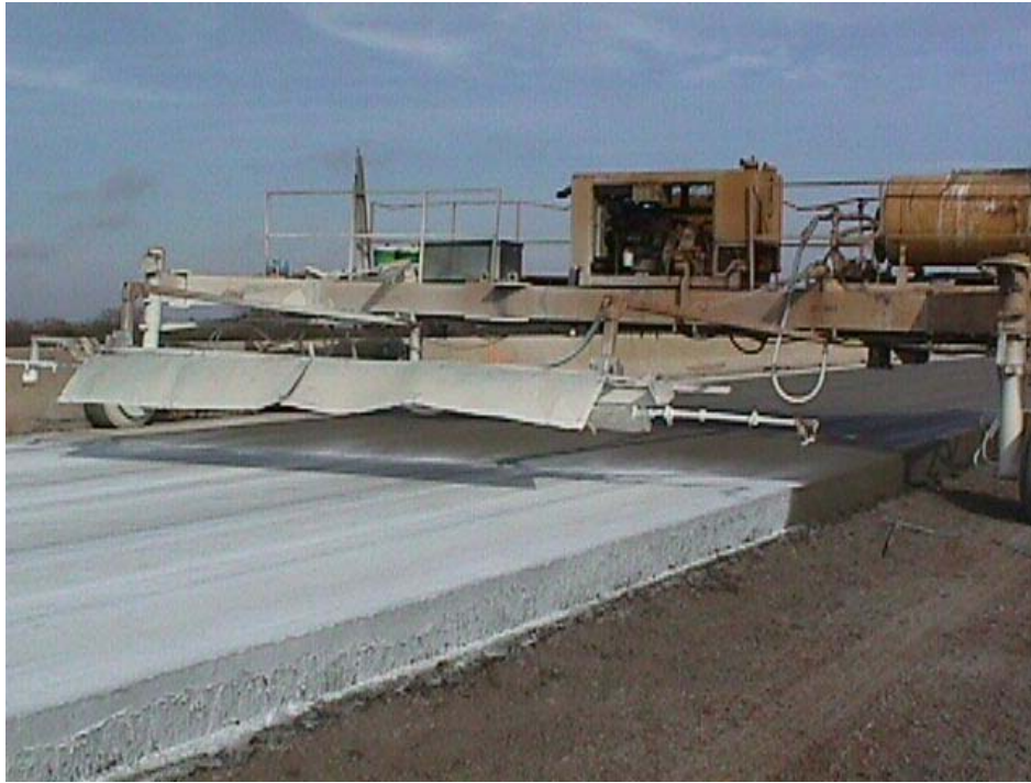
Figure 6.12 Application of curing compound
