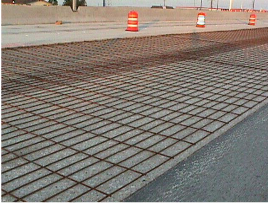
Figure 6.9 Steel placed directly on top of substrate
