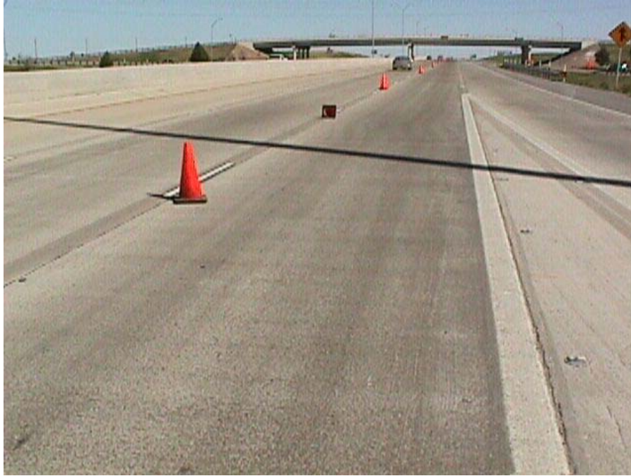
Figure 8.20 Eastbound BCO segment with no delaminations
