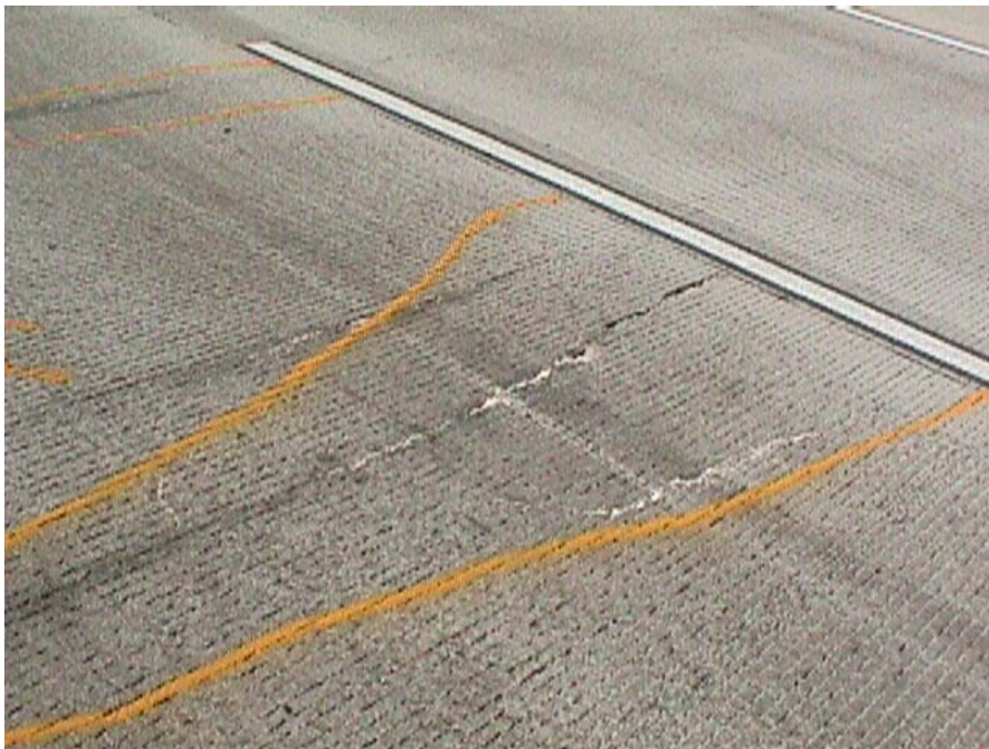
Figure 8.22 Delamination of the outside lane with extensive transverse cracking
