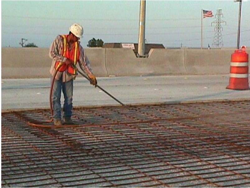
Figure 6.5 Final cleaning of the substrate, just prior to placement
