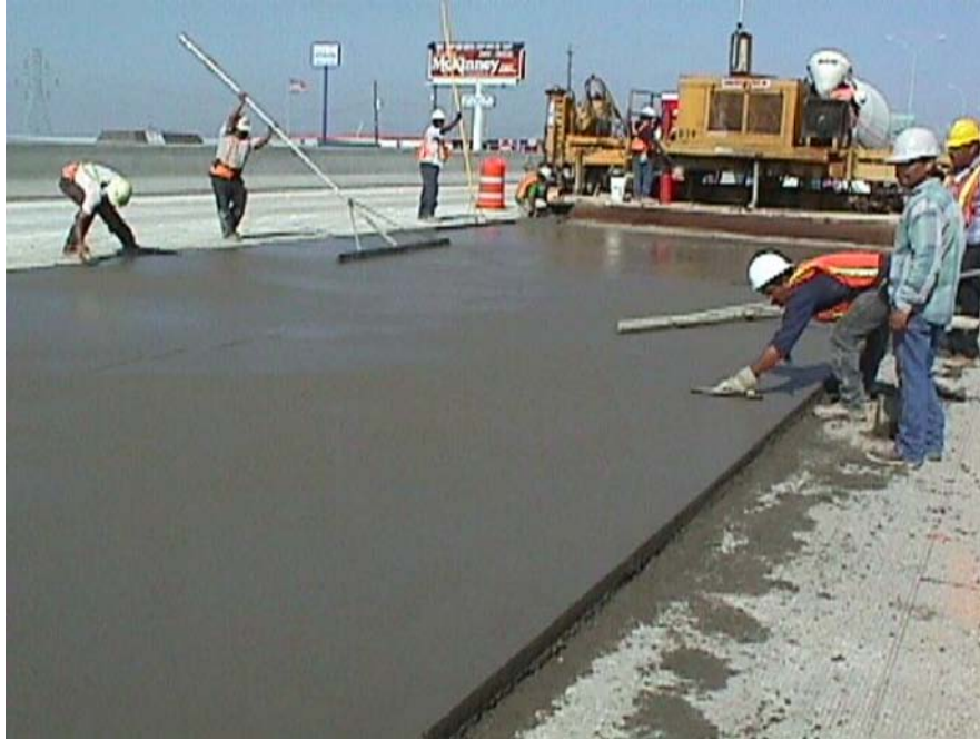
Figure 8.18 Finishing operations
