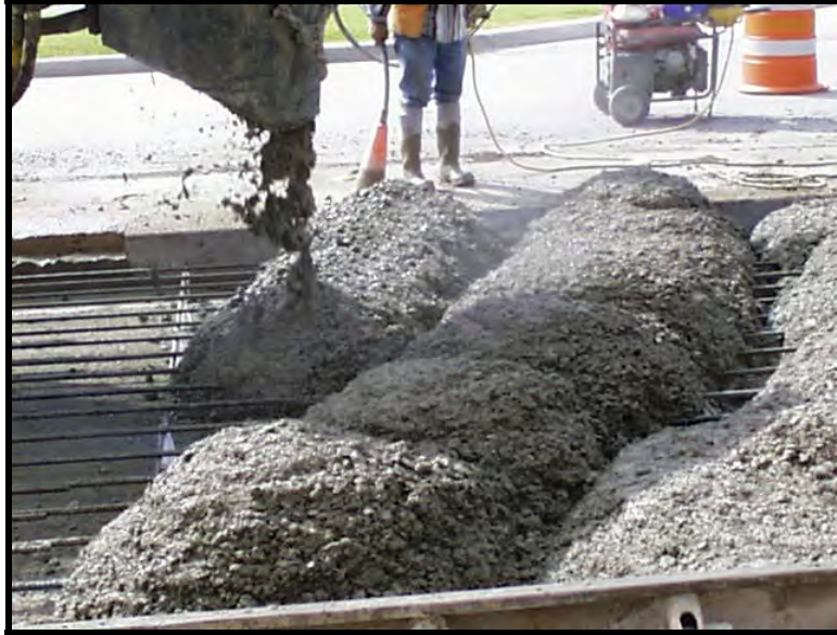
Figure 4.8: Placement of Concrete Using Spreader
