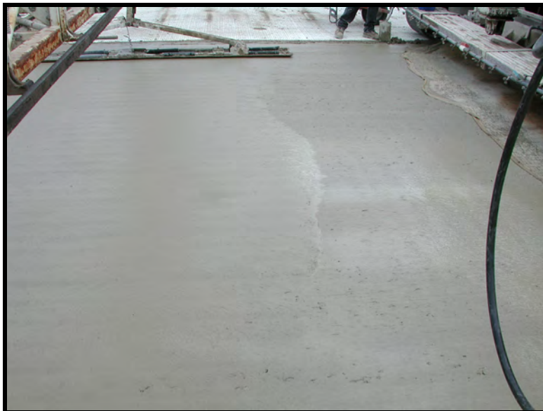
Figure 5.29: Smooth Surface during Initial Finishing (Section 7—SnF2-1.5)
