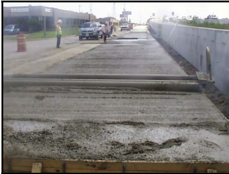
Figure 4.9: Roller Screed Operation
