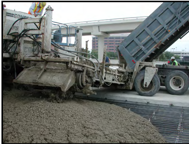
Figure 5.6: Placement of Concrete Using Slipform Paver
