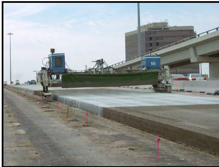
Figure 5.10: Application of Curing Compound
