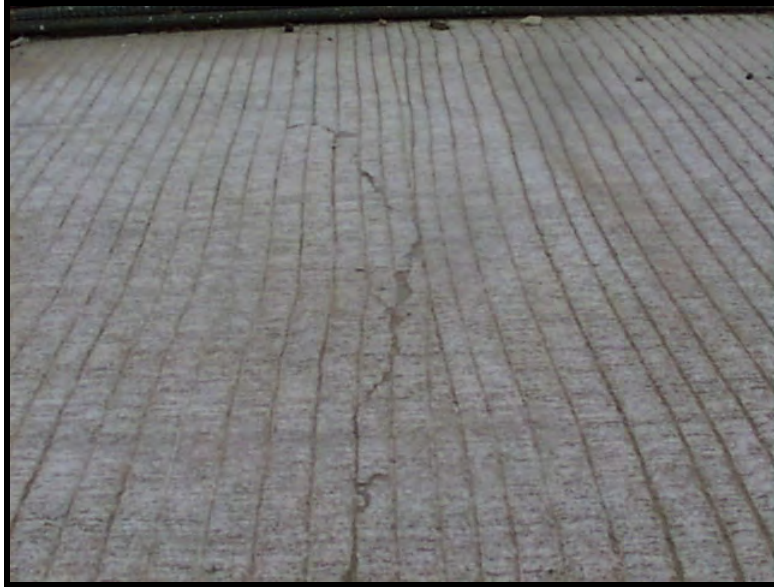
Figure 5.34: Evidence of Spalling in Existing Northbound Lane
