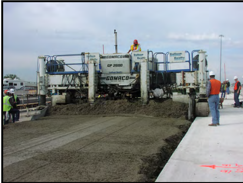
Figure 5.23: Smooth Flow during Placement (Section 1—SnF1-4)
