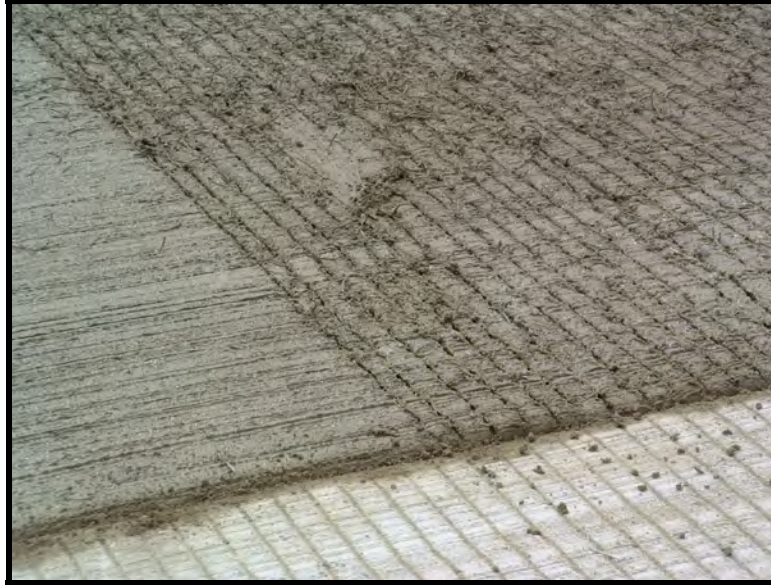
Figure 5.26: Fibers Disturbed during Tining (Section 1—SnF1-4)
