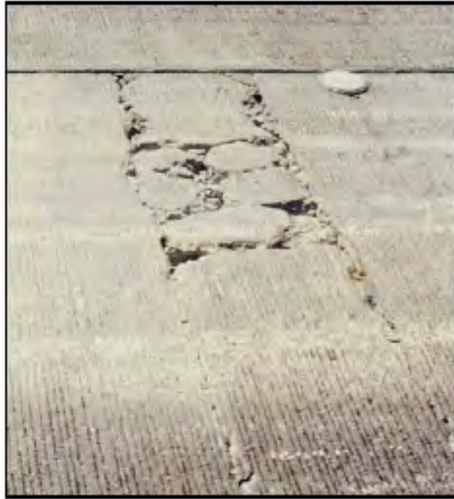
Figure 2.2: Edge Punchout (Miller 1993)
