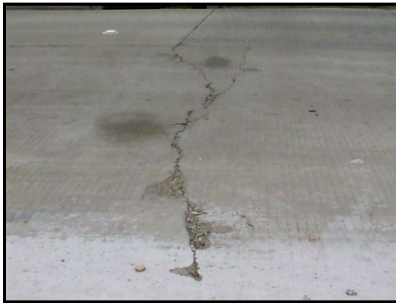
Figure 4.17: Evidence of Spalling in Existing Lane
