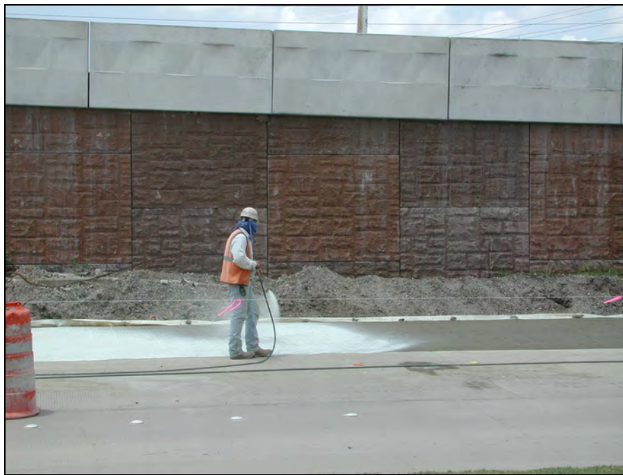
Figure 2.8: Curing Application
