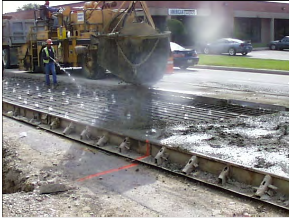
Figure 2.6: Concrete Spreader
