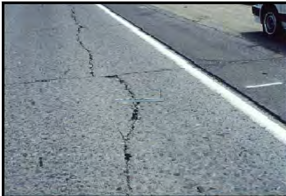
Figure 2.4: Longitudinal Cracking (Miller 1993)
