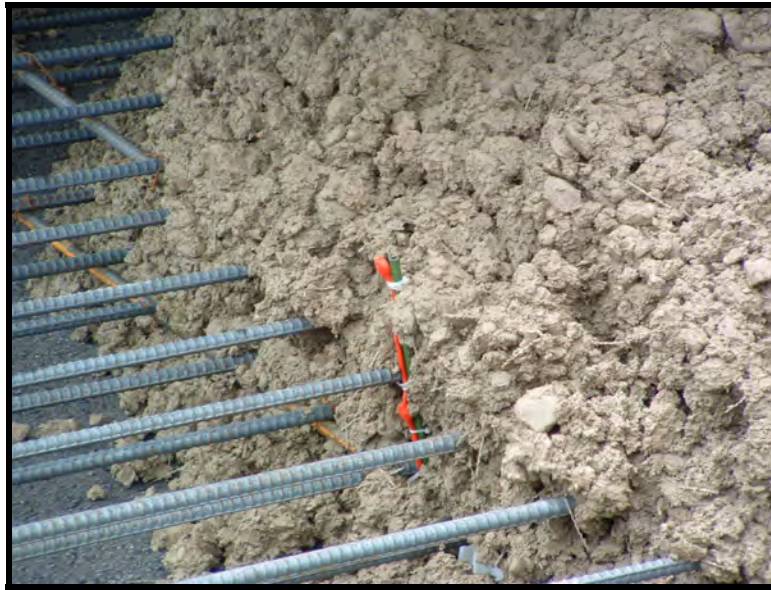
Figure 5.40: iButton during Construction
