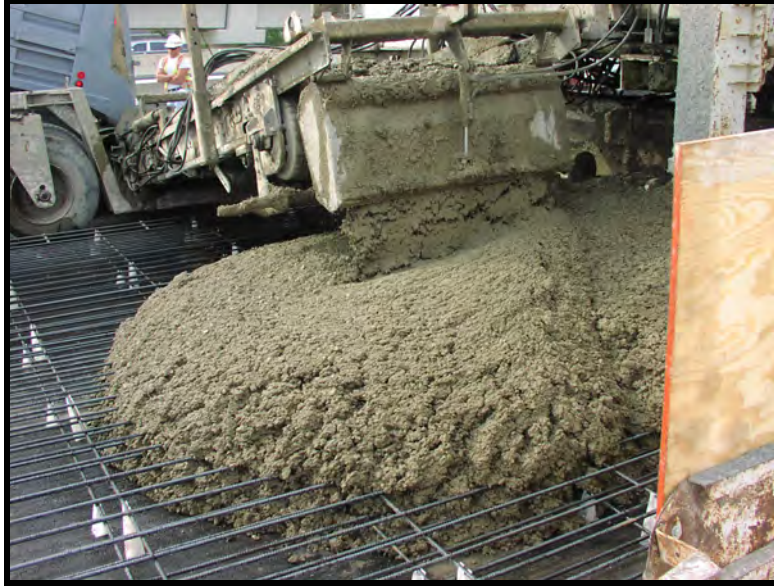
Figure 5.22: Nice Uniformity during Placement (Section 1—SnF1-4)
