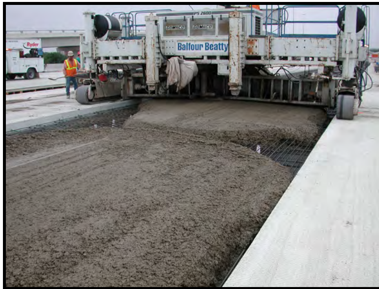
Figure 5.15: Discontinuity in Concrete during Placement (Section 5—SF1-40)
