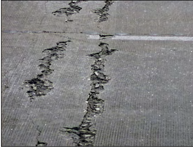
Figure 2.1: Severe Spalling (Won 2001)
