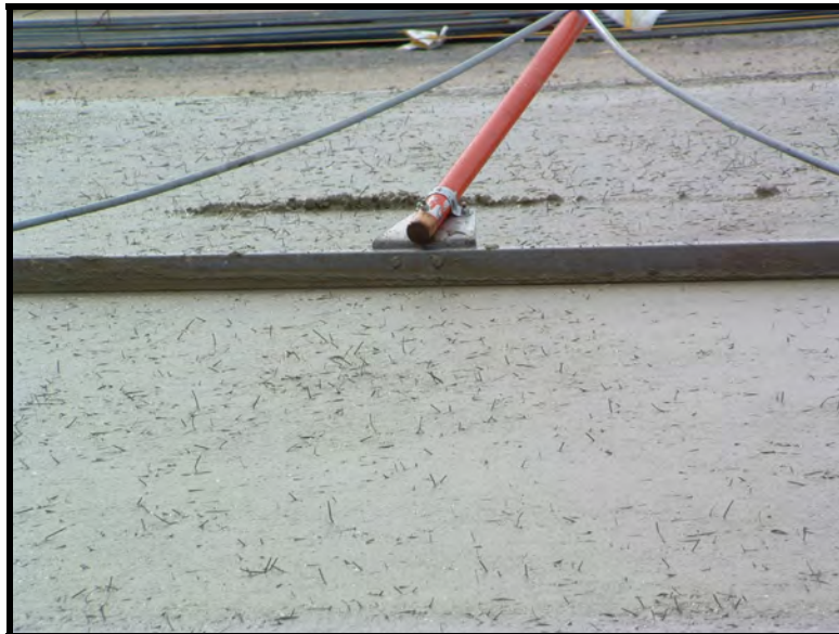
Figure 5.25: Fibers Disturbed by Bull Float (Section 1—SnF1-4)
