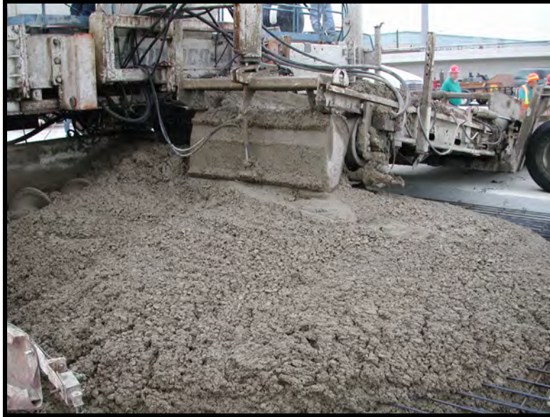
Figure 5.13: Nice Uniformity during Placement (Section 1—Control)
