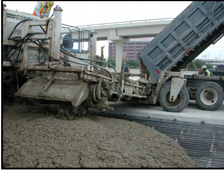
Figure 5.31: Segregation of Coarse Aggregate (Section 8—SnF3-0.5)
