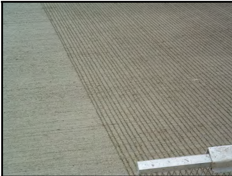
Figure 5.20: Fibers Undisturbed during Tining (Section 3—SF2-27.5)
