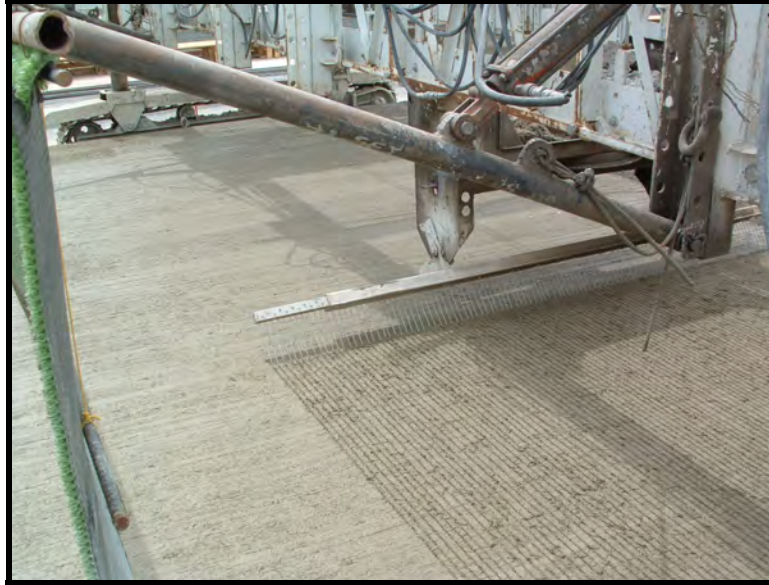
Figure 5.9: Mechanical Application of Tining
