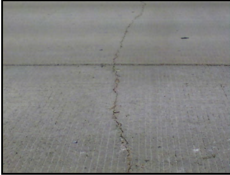
Figure 4.18: Horizontal Reflection Cracking in Existing Lane
