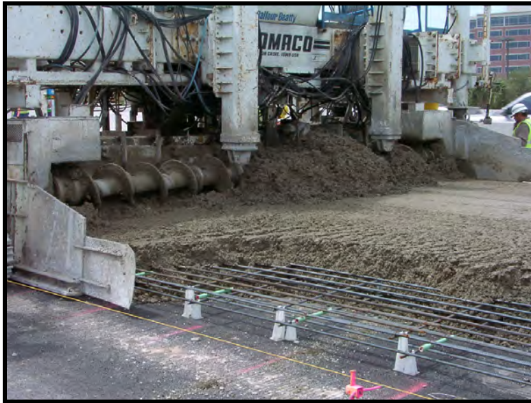
Figure 5.7: Vibrating and Placement of Concrete
