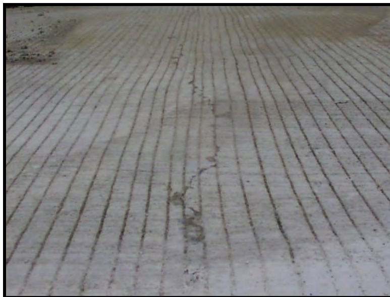
Figure 5.33: Evidence of Spalling in Existing Northbound Lane
