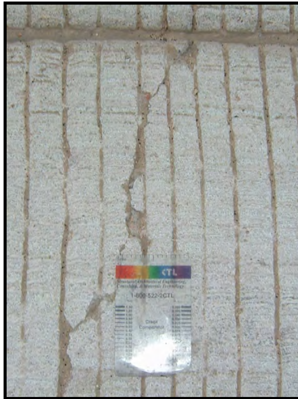
Figure 4.36: Evidence of Spalling in Control Sections
