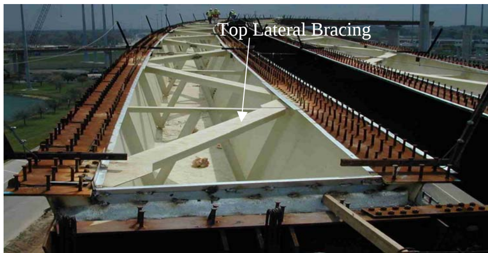
Figure 3.1 Top Flange Lateral Truss
