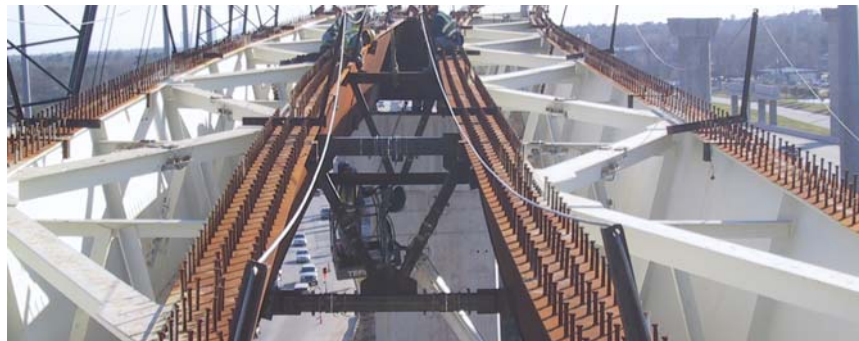
Figure 1.4 External box girder bracing
