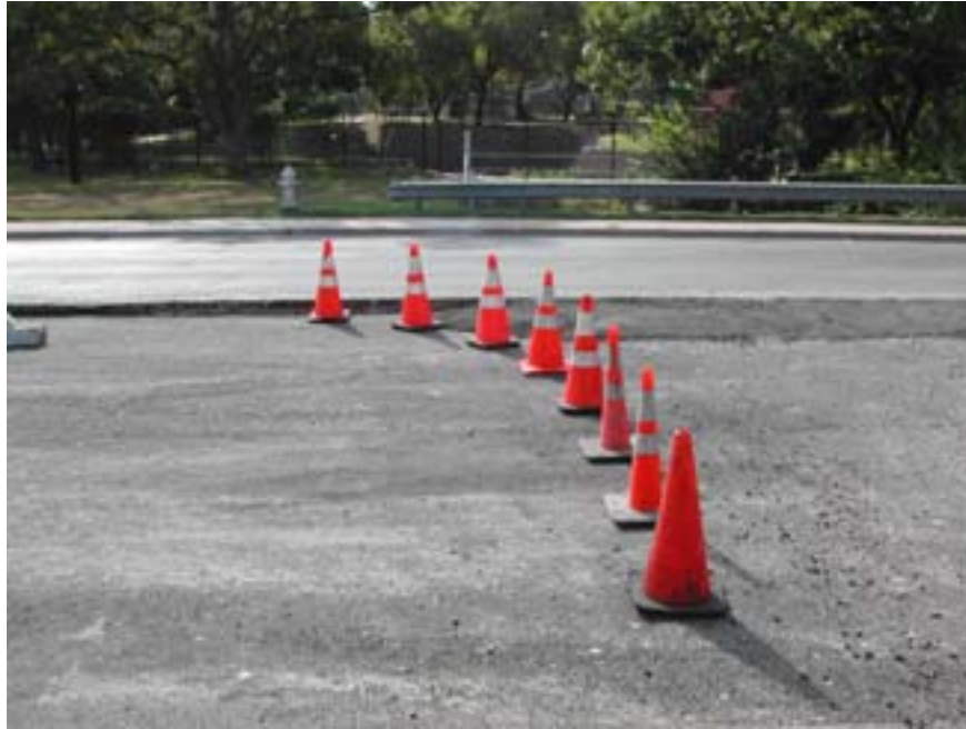
Figure 2.9 Recommended placement of cones on adjacent road
