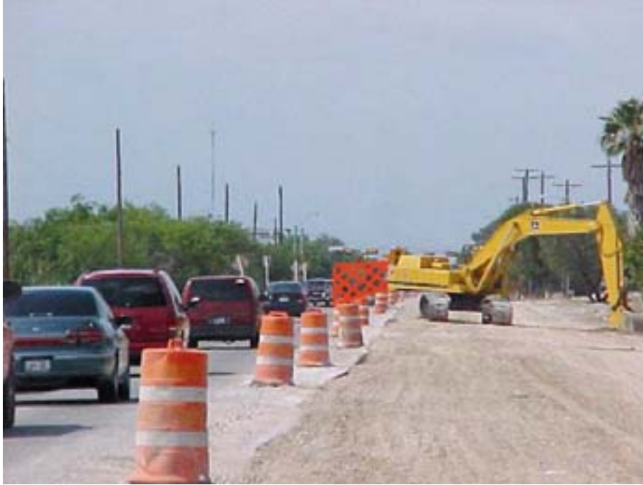
Figure 1.12 Recommended protection of traffic in close proximity to construction equipment
