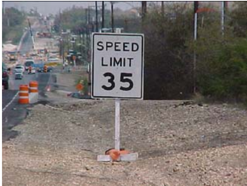
Photo C.19 Sign support did not meet the minimum mounting height
