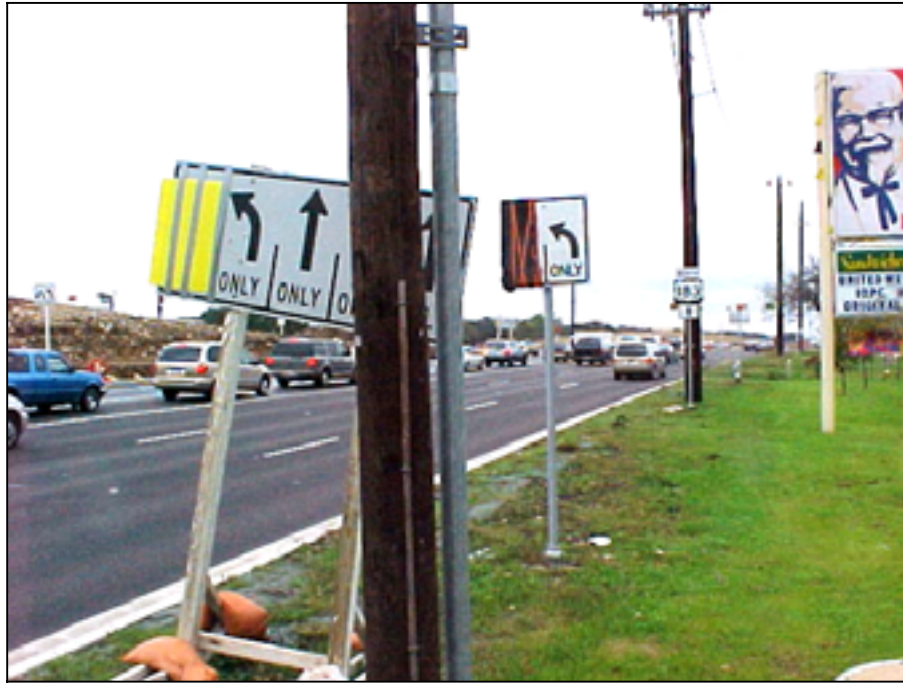
Photo C.15 Second sign hidden by previous. Second sign is unnecessary.
