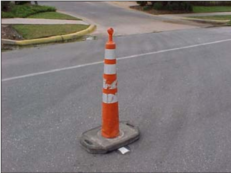
Photo C.2 Damaged edge line channelizer
