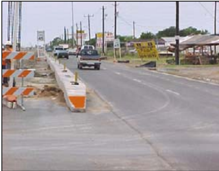
Figure 3.12 Recommended Vertical Markings of Low-Profile Barriers
