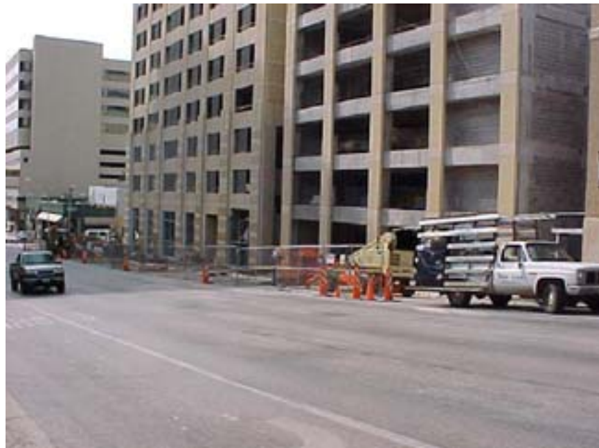
Photo A.4 Austin, Work Zone #2, Lavaca St.: General view
