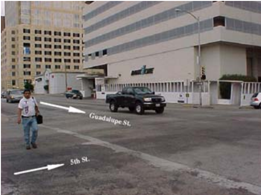
Photo A.5 Austin, Work Zone #3, 400 Guadalupe St.: General view of work zone section on Guadalupe St., block 500
