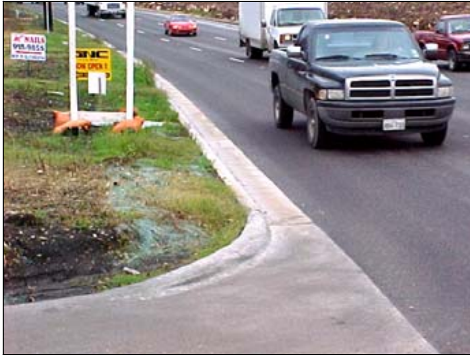
Photo C.13 Small radius curve on the busy local access road
