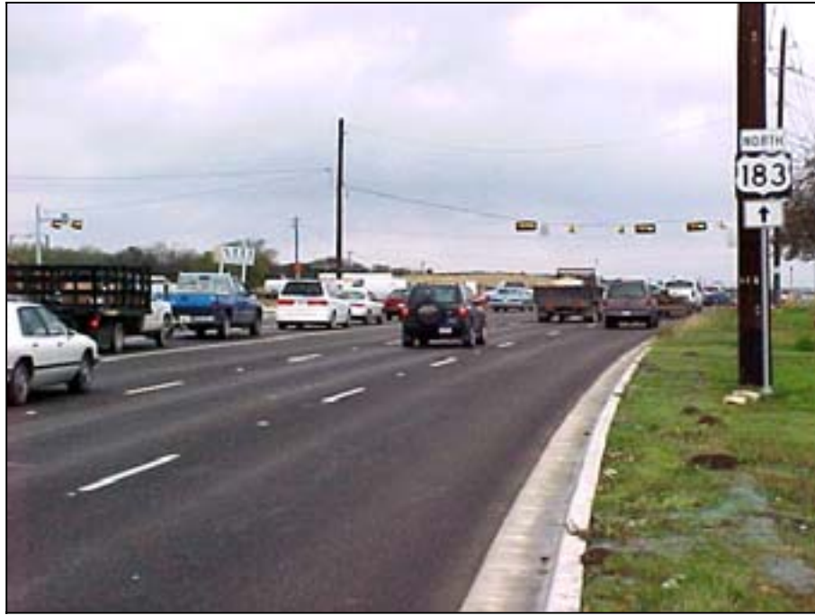
Photo A.25 Austin, Work Zone #9, Research Blvd.: Northbound view of Research Blvd. and Anderson Mill Rd. intersection
