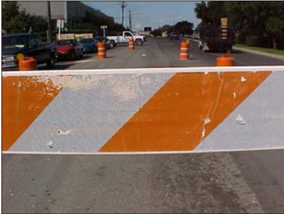
Photo C.11 Typical barricade's reflective sheeting damage
