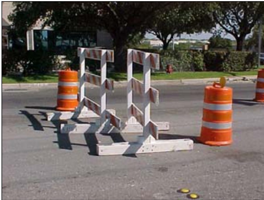
Photo C.10 Overlapping barricades installation
