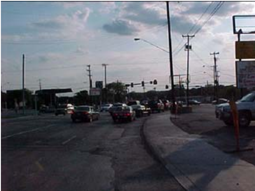
Photo B.13 San Antonio, Work Zone #15, Blanco–Jackson Keller Intersection: Southbound approach (Blanco Rd.), facing south
