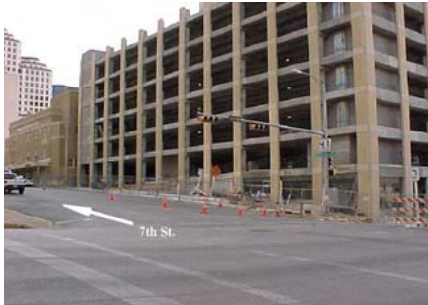
Photo A.3 Austin, Work Zone #1, 600 Guadalupe St.: General view of work zone on 7 th Street
