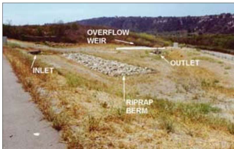
Figure 4-3: Unlined Extended Detention Basin (Caltrans, 2003a)
