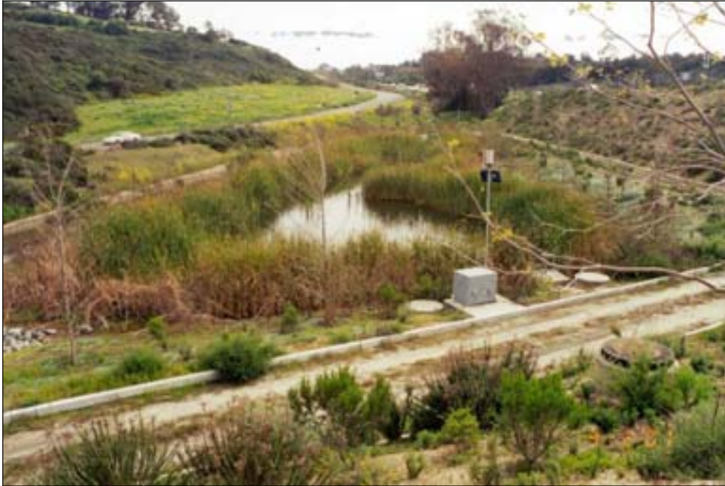
Figure 4-4: An Example of a Wet Basin in California (Caltrans, 2003a)
