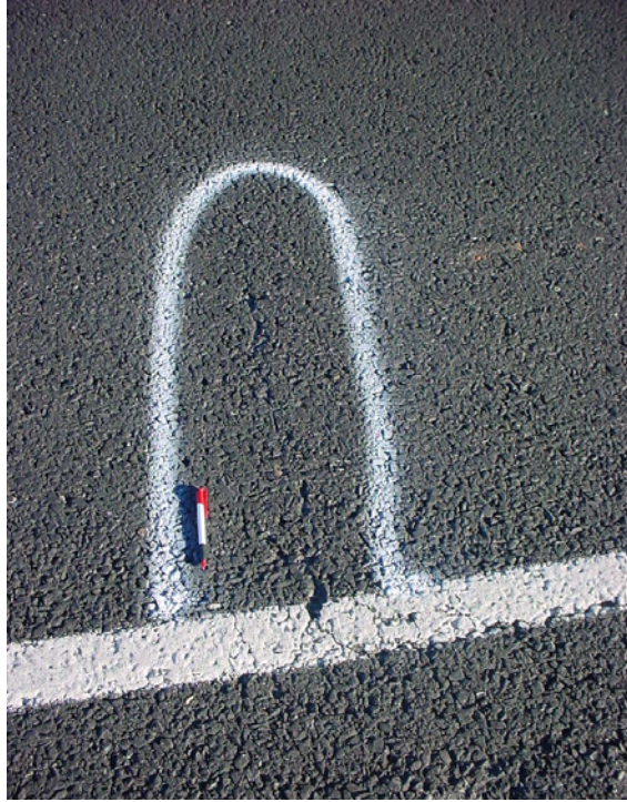
Figure 3.1 Low-level transverse crack
