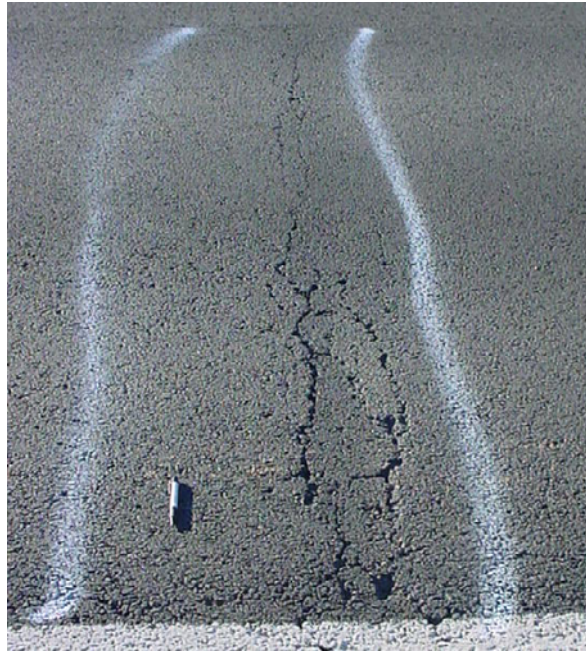
Figure 3.3 High-level transverse crack
