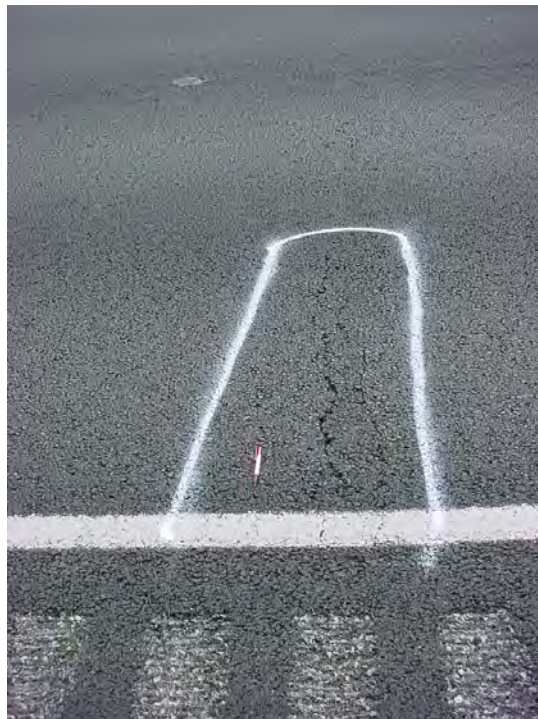
Figure 2.2. Moderate-level transverse crack
