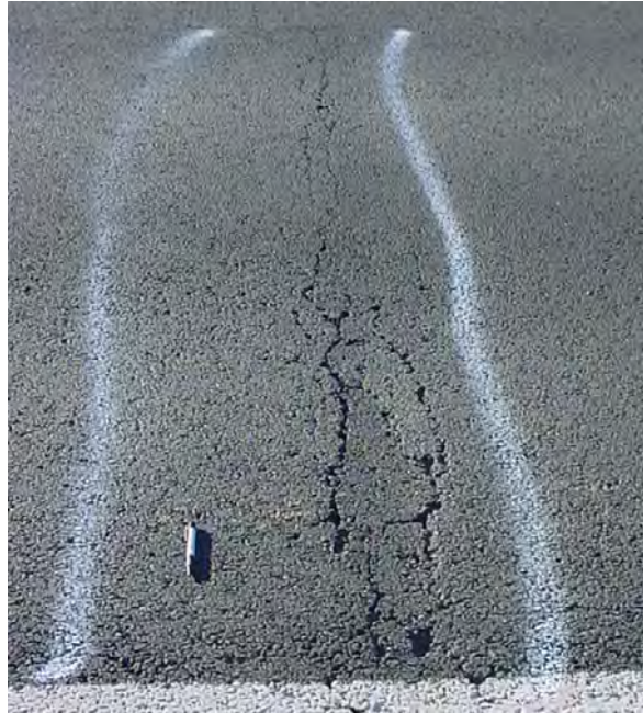
Figure 2.3. High-level transverse crack
