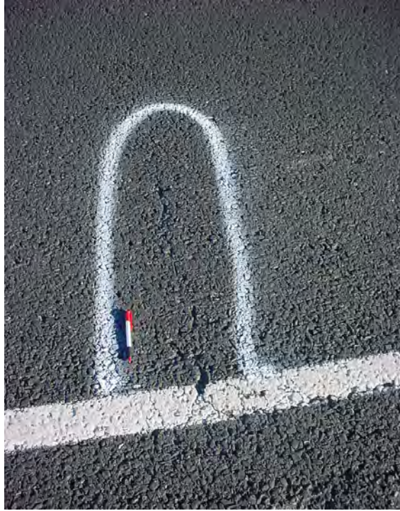
Figure 2.1. Low-level transverse crack
