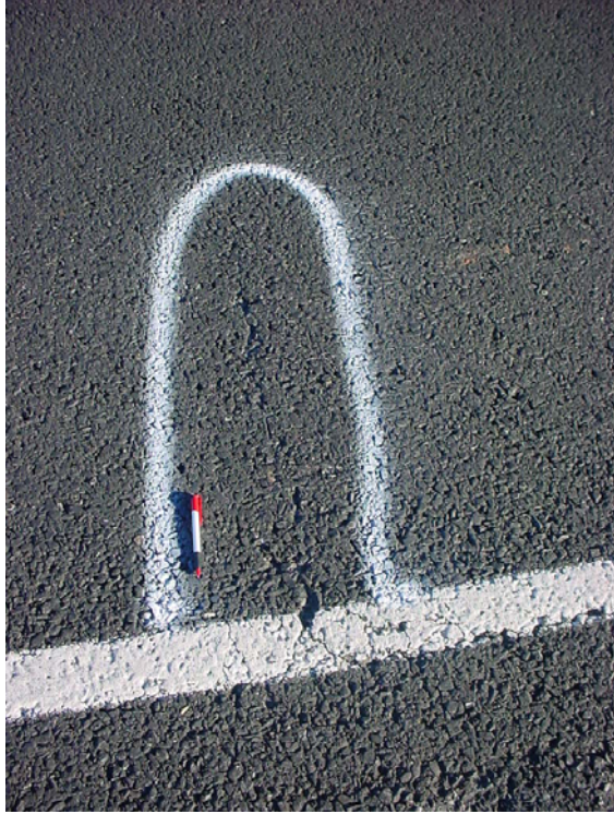
Figure 3.1 Low-level transverse crack
