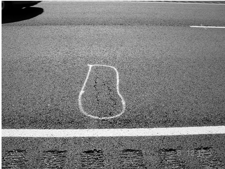
Figure B.12 Low transverse crack between 1195 – 1196
