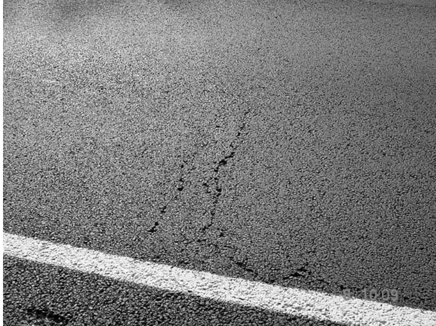
Figure B.3 Low transverse crack between 1296 – 1297
