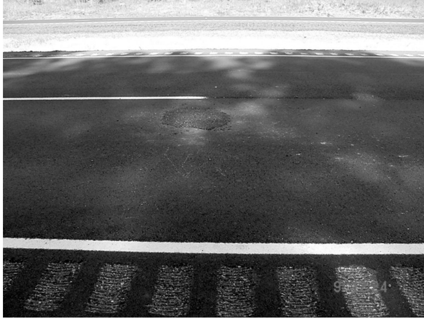
Figure B.15 Low pothole between 1238 – 1239 (Underlying Concrete Failure)
