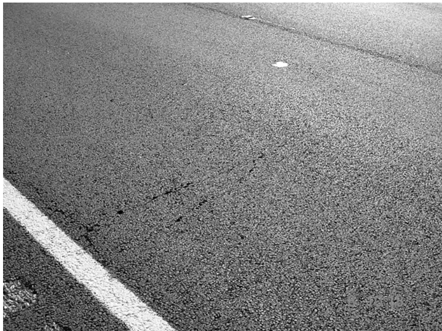
Figure B.4 Low transverse crack between 1292 – 1293
