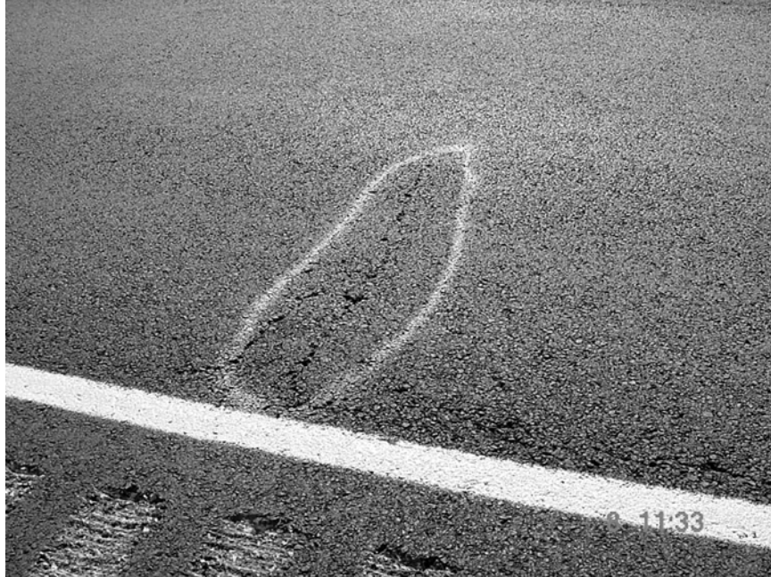
Figure B.7 Moderate transverse crack between 1234 – 1235
