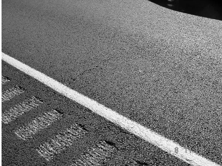
Figure B.5 Low transverse crack between 1250 – 1251
