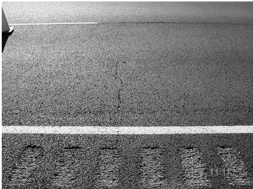
Figure B.6 Low transverse crack between 1245 – 1246
