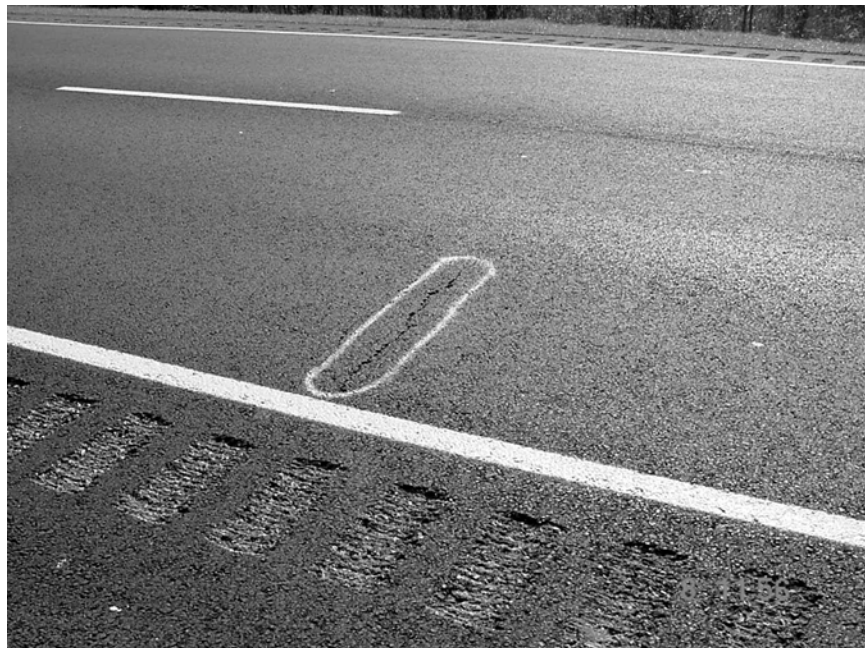
Figure B.10 Low transverse crack between 1210 – 1211
