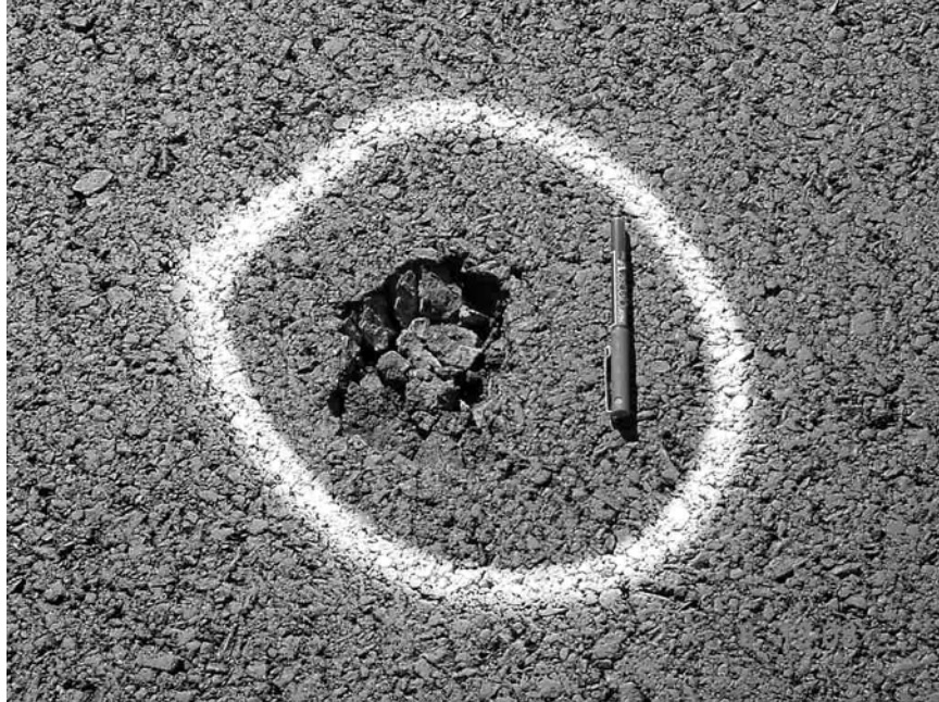
Figure B.13 Low pothole between 1150 – 1151
