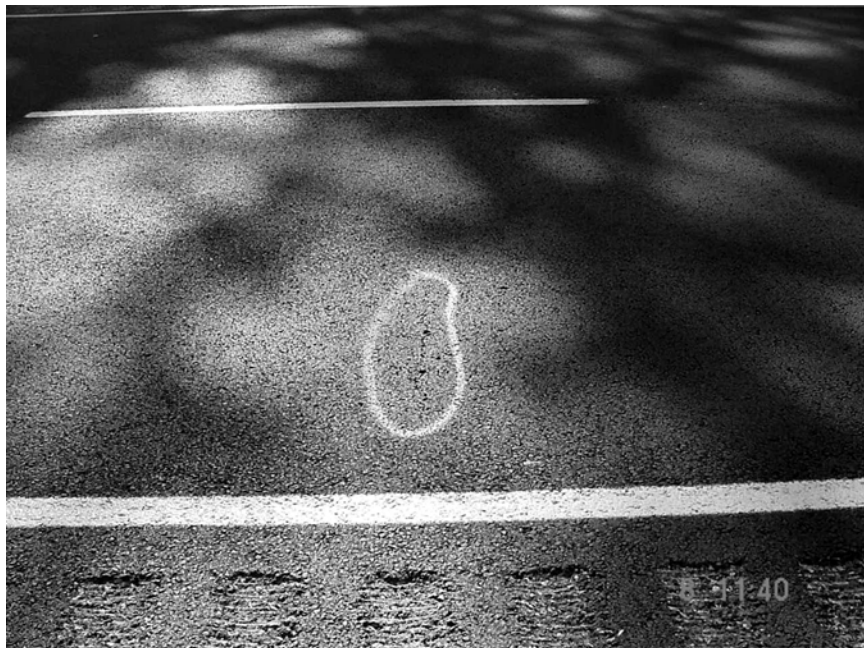
Figure B.8 Low transverse crack between 1228 – 1229
