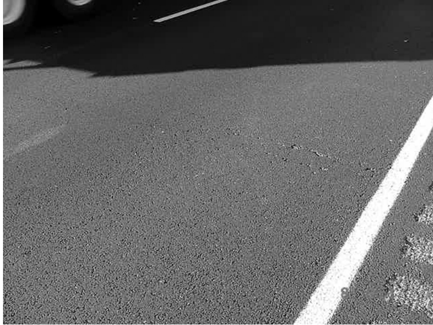
Figure B.1 Moderate transverse crack between 1305 – 1306
