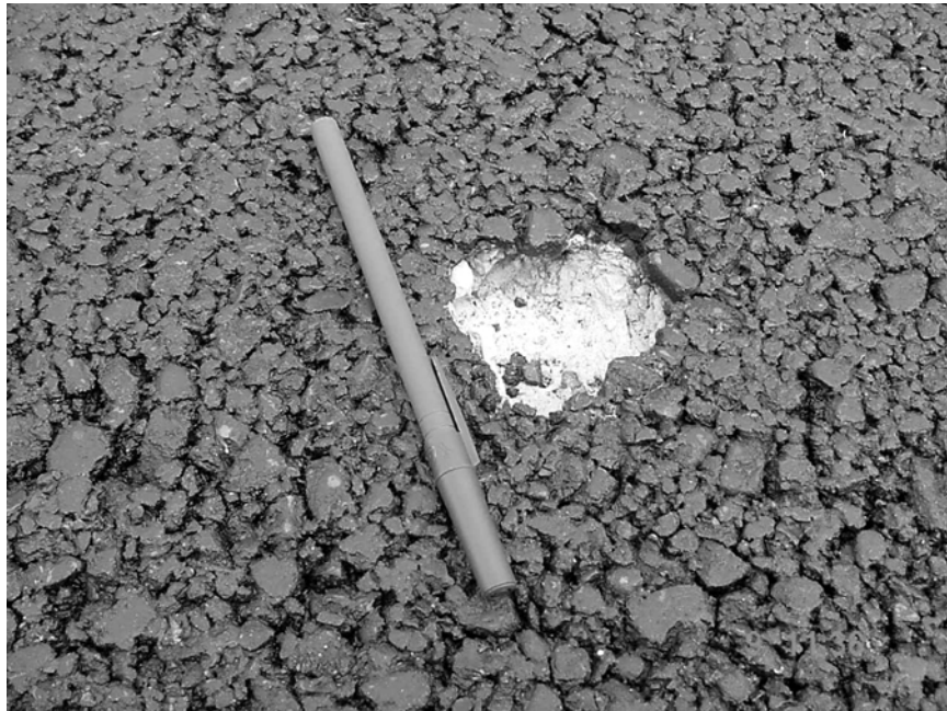
Figure B.16 Low pothole between 1288 – 1289 (Uncoated Limestone Contaminant)
