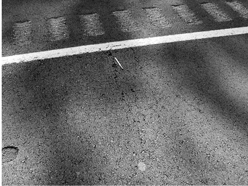
Figure B.17 Low transverse crack between 1292 – 1293
