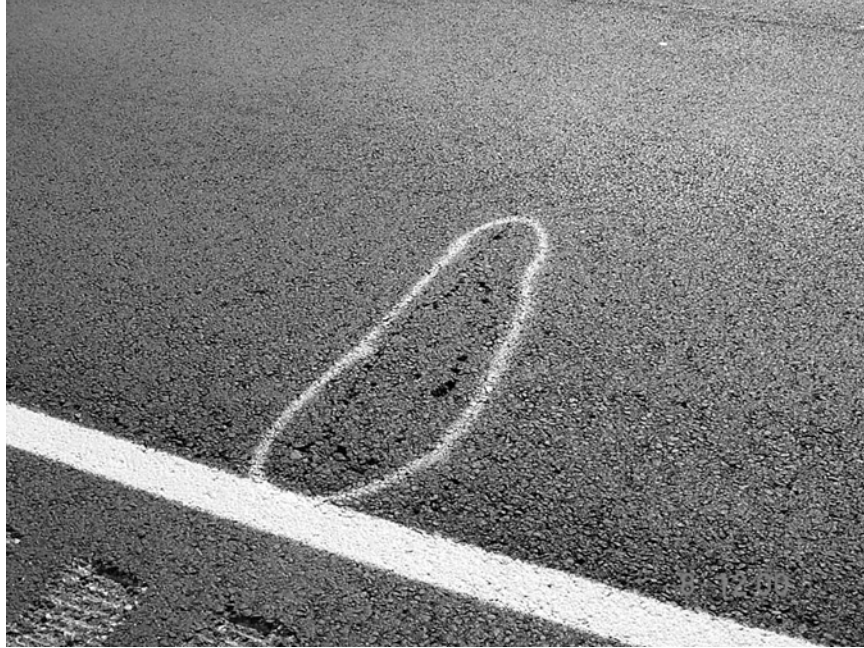
Figure B.11 Low transverse crack between 1215 – 1216
