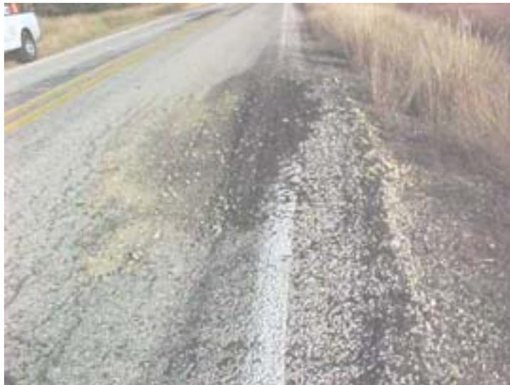
**Figure 3.5 Example of Damage Done by Salt Water Trucks**
