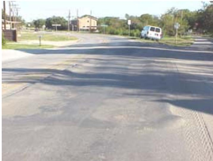
**Figure 3.9 Example of Pavement Rutting**
