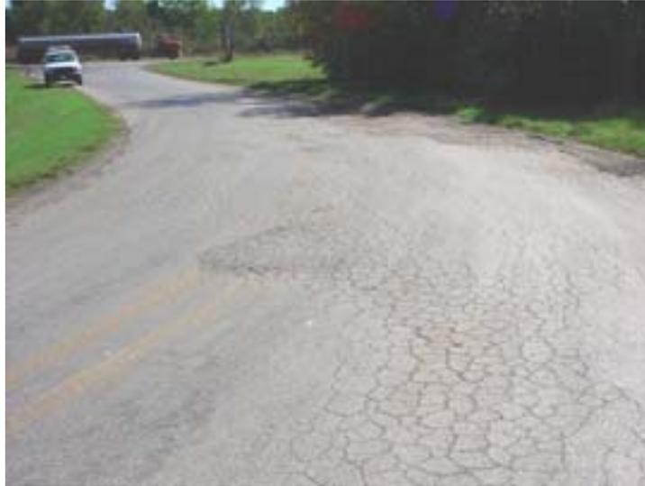
**Figure 3.4 Example of Damage Done by Oil Field Trucks**
