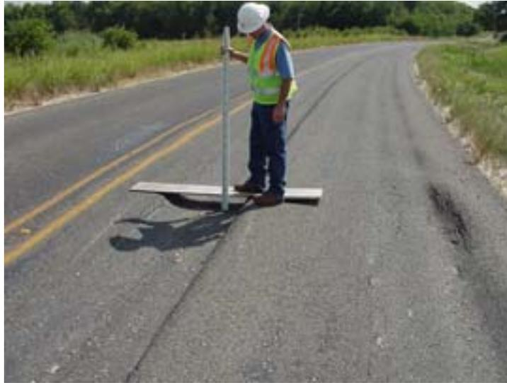
**Figure 3.2 Example of Damage Done by Grain Haulers**
