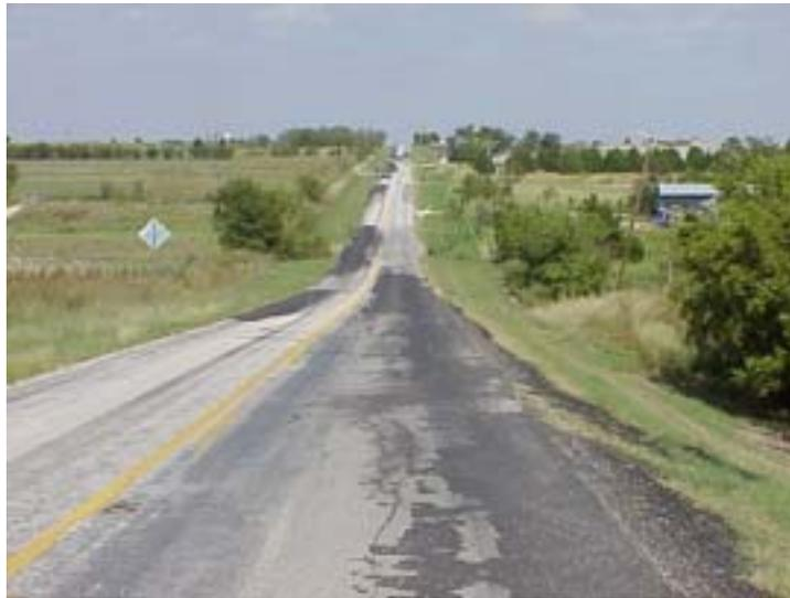
**Figure 3.3 Example of Shoulder Damage**
