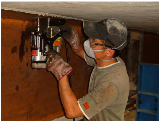
a) Drilling through the steel flange
