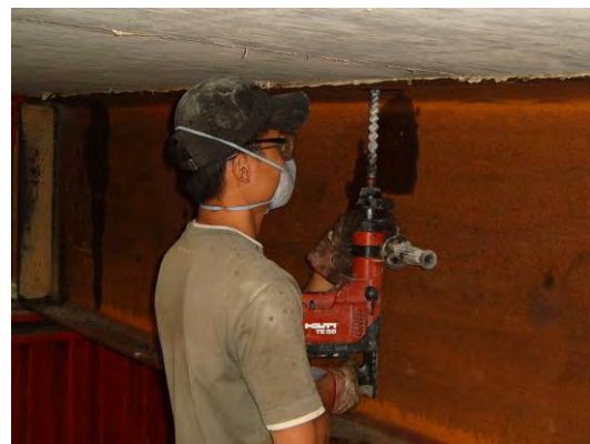
b) Drilling into the concrete
