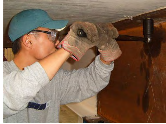
d) Tightening with torque wrench
