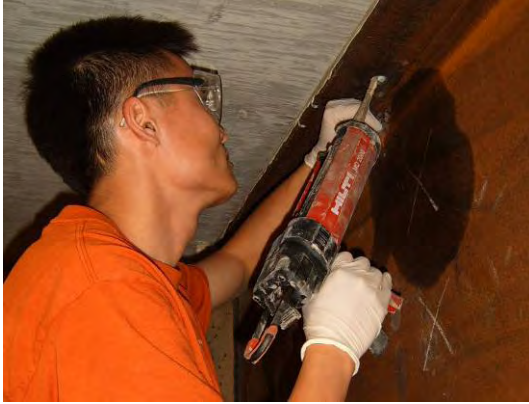
c) Injecting adhesive
