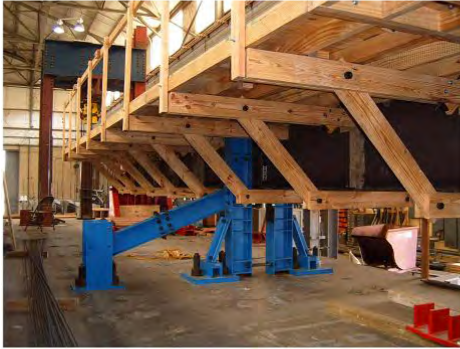
Figure 5.3: Concrete formwork
