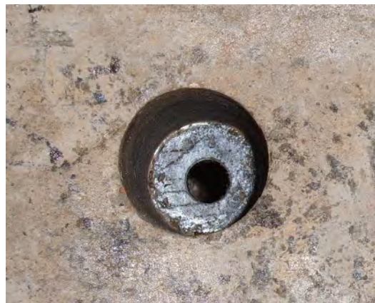
Figure 5.7: Drilled holes for DBLNB installation
