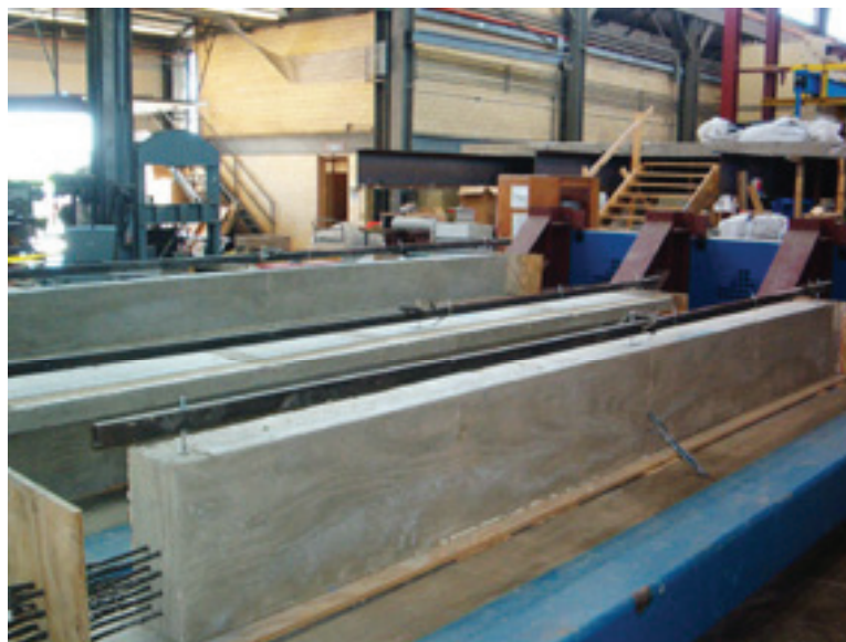
Figure 2: Fabrication of Pretensioned Beams
