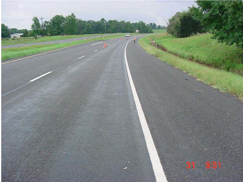
Figure 4.3. Test section crack sealed with C2 in Atlanta District
