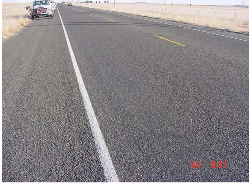
Figure 4.5. Test section crack sealed with C1 in Amarillo District
