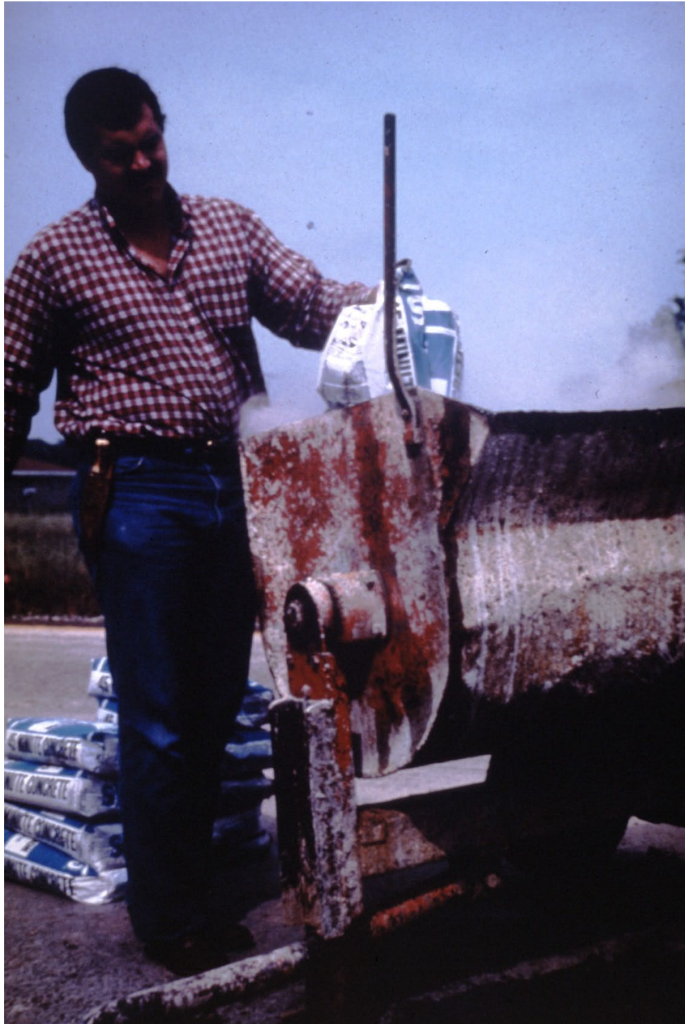
Slide 84. Adding rapid-setting material
