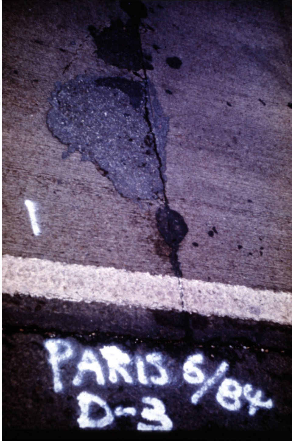
Slide 60. A spall filled with asphalt
