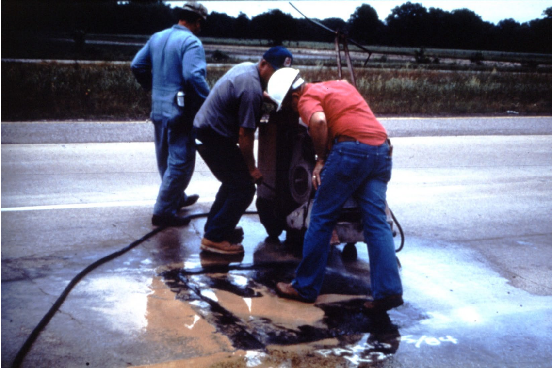
Slide 69. Sawing around repair area
