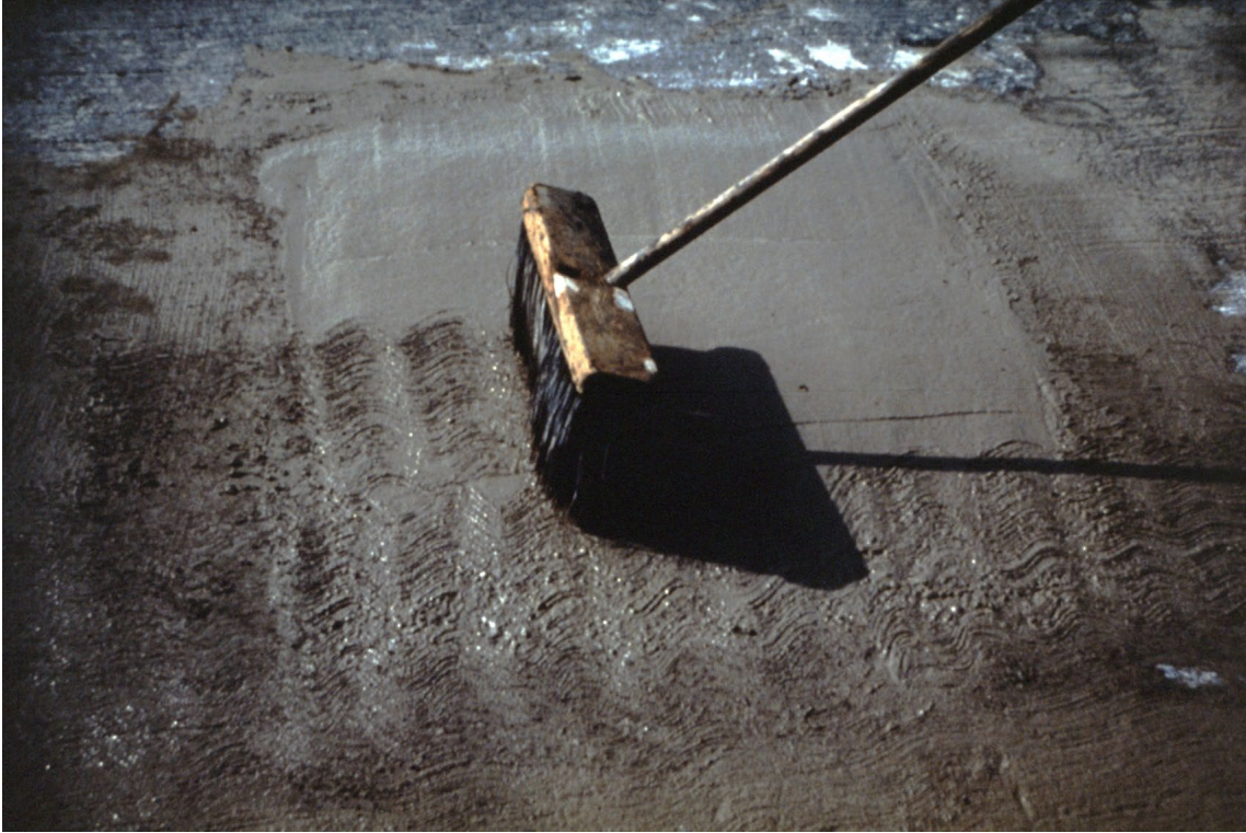
Slide 92. Texturing the surface with a broom
