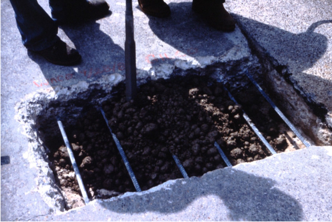
Slide 88. Vibrating the concrete
