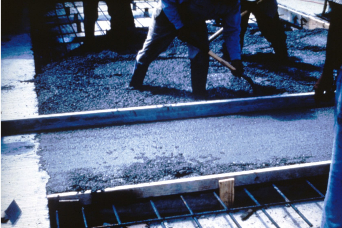
Slide 104. Screeding and finishing
