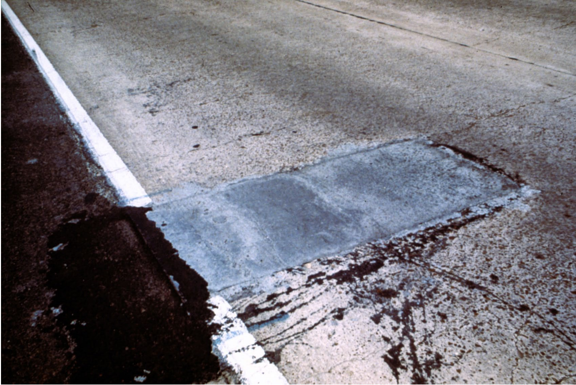
Slide 61. A full-depth repair
