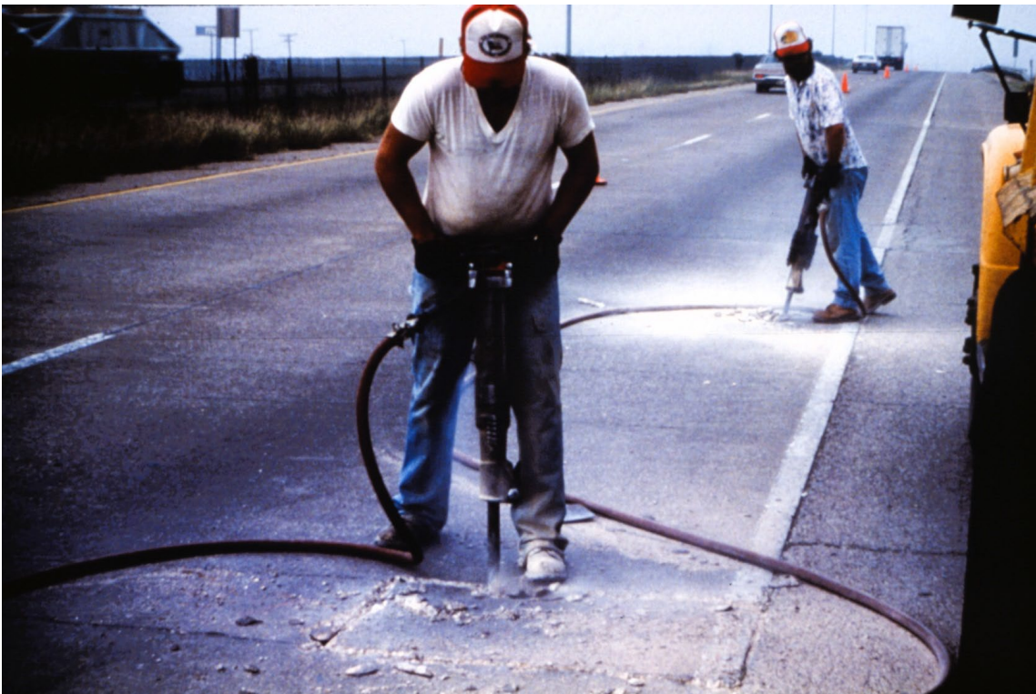
Slide 70. Jack hammer breaking out sawn area
