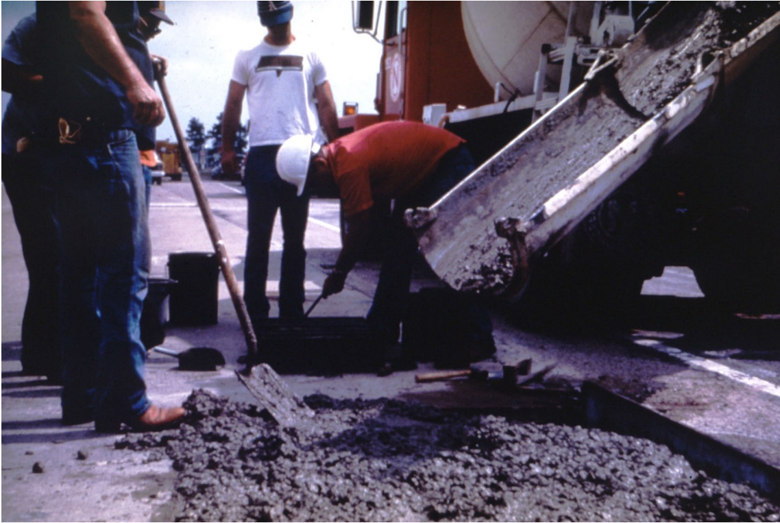
Slide 102. Placing Class "K" concrete
