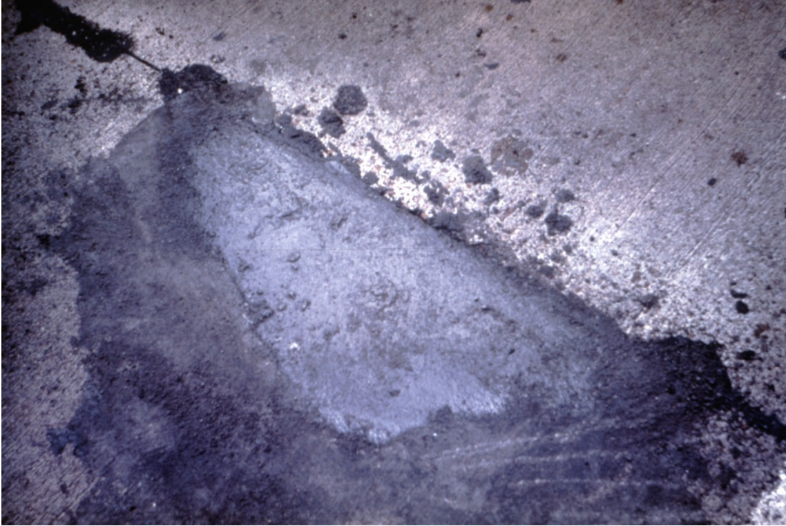
Slide 94. Completed spall repair
