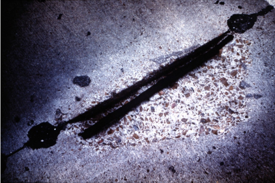
Slide 65. Spall ready for repair
