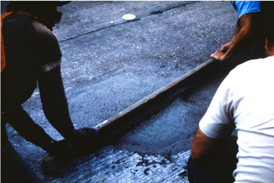
Slide 91. Finishing screeding the surface
