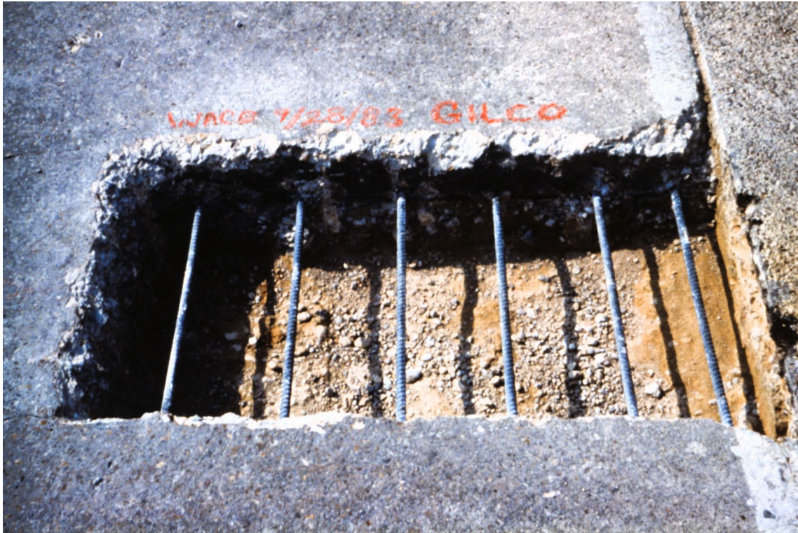
Slide 71. Full-depth repair ready to receive repair materials
