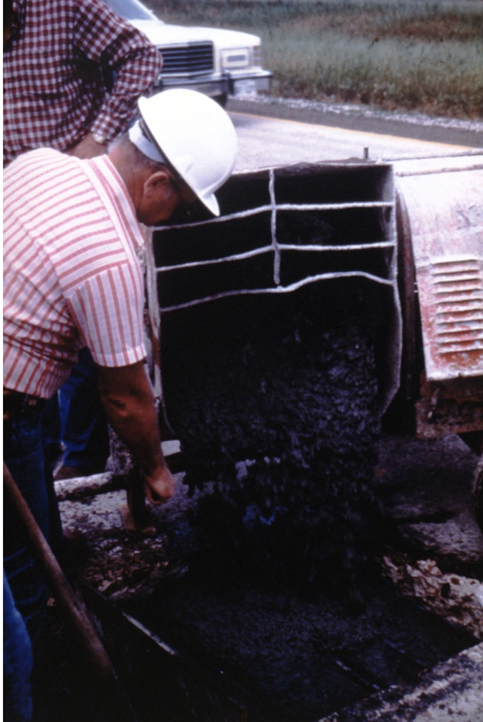
Slide 87. Placing the material into the repair area
