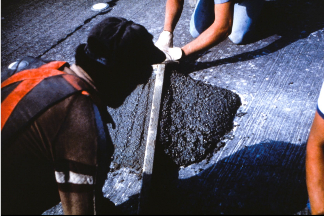
Slide 90. Screeding the surface with a 2x4
