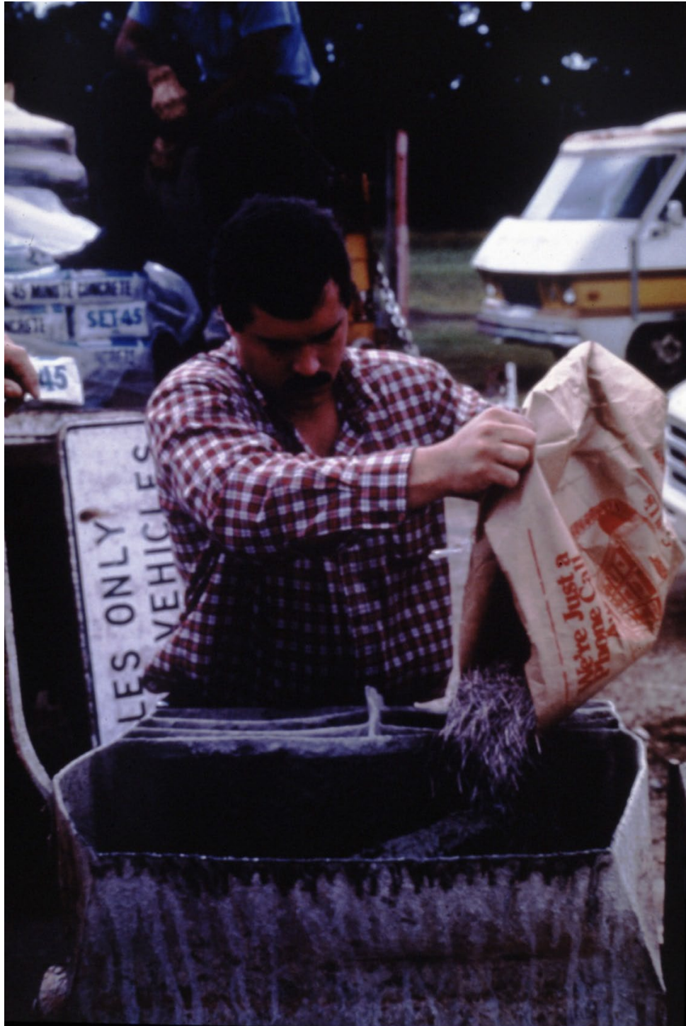
Slide 83. Adding steel fibers to the mix
