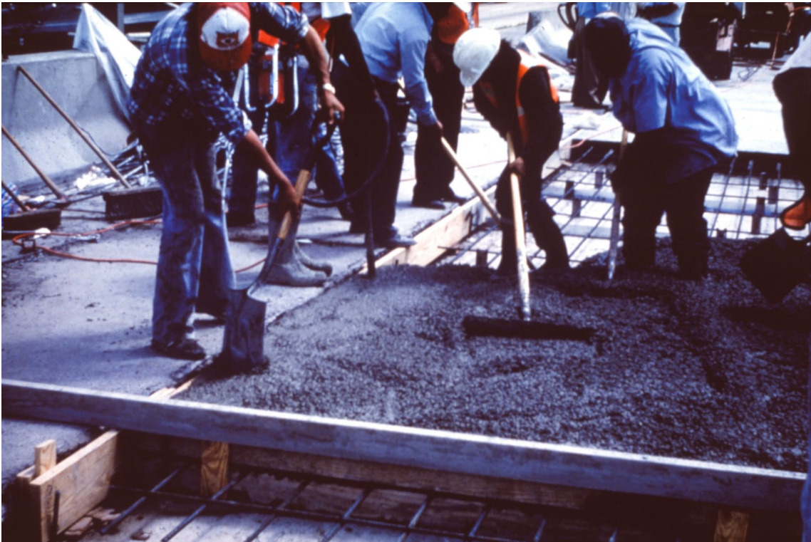
Slide 103. Spreading and consolidating
