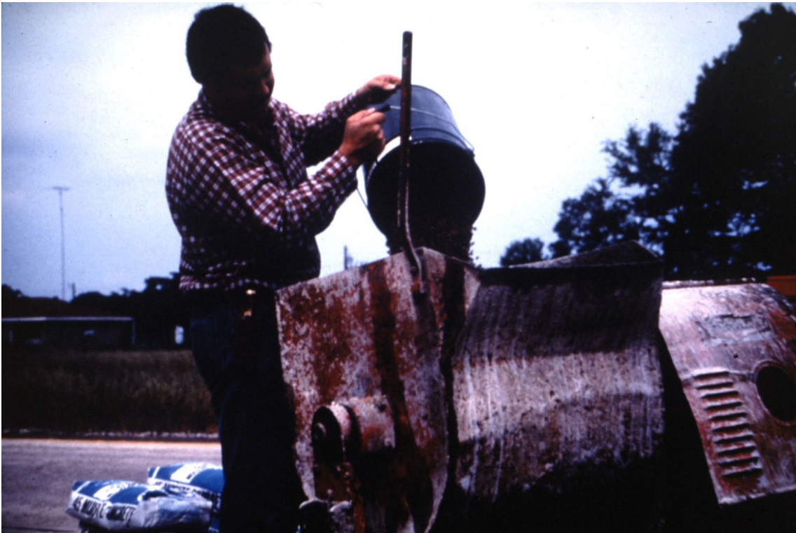
Slide 82. Adding coarse aggregate to the mortar mixture
