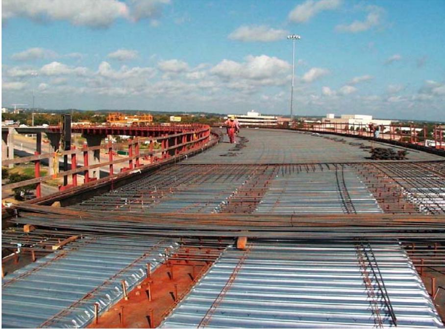
**Figure 4.3 Deck Forms and Reinforcement Installation**
