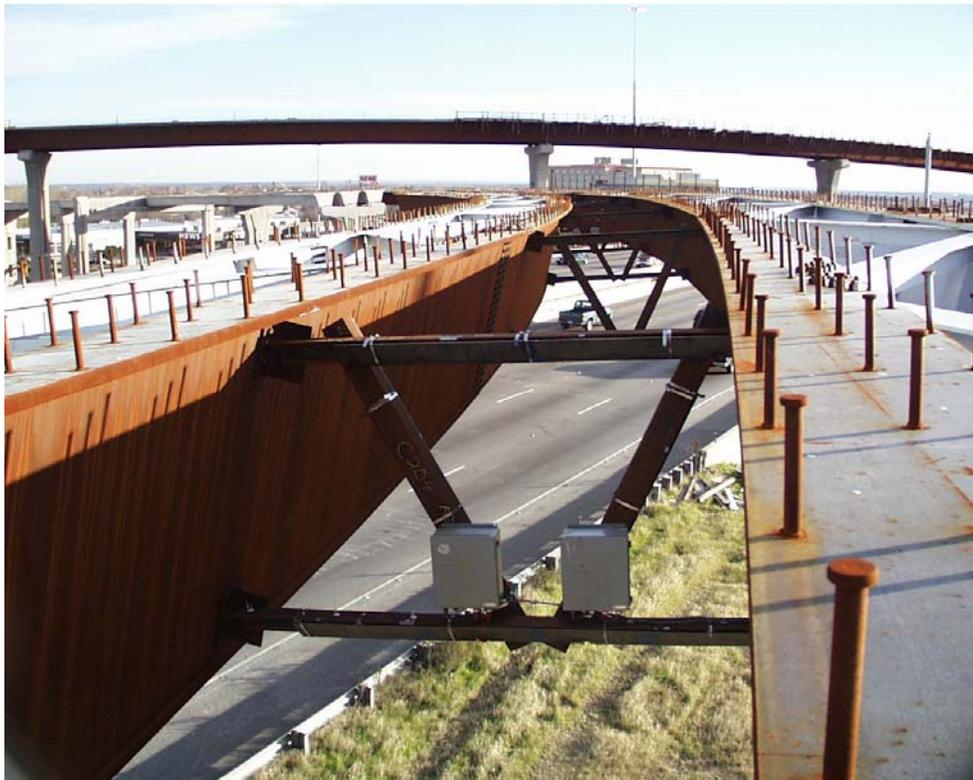
**Figure 2.14 Intermediate External Diaphragm #11 -- Looking South**
