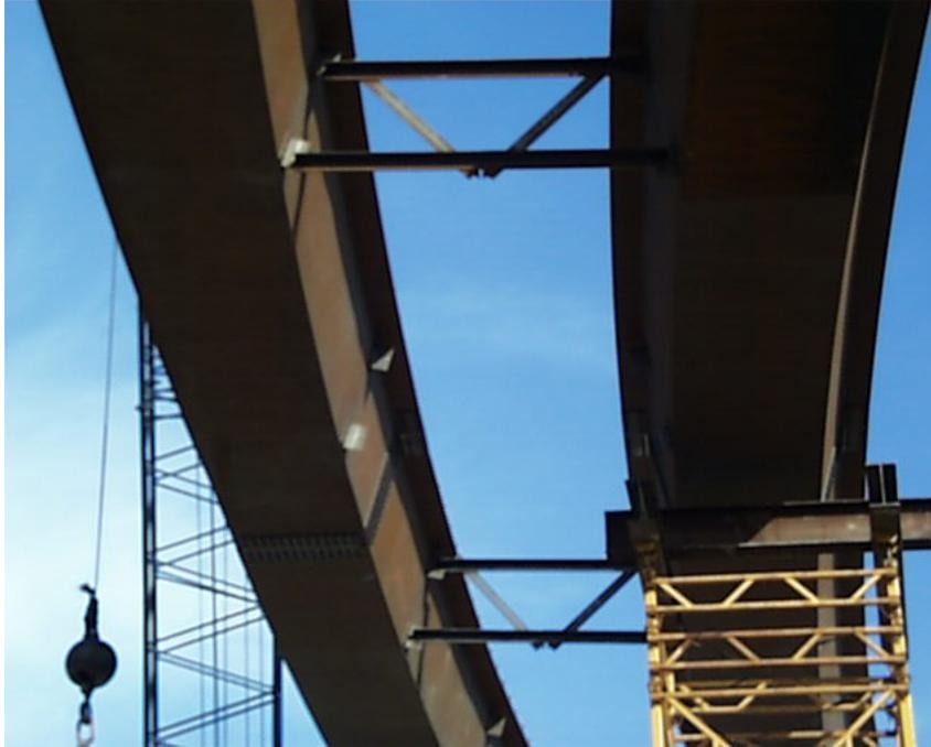
**Figure 2.10 Installed External Diaphragms on Z-Connect**
