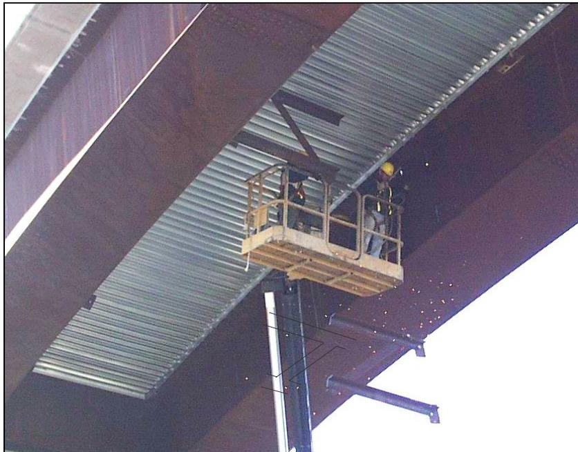
**Figure 2.11 Flame Cut Removal of External Diaphragms**
