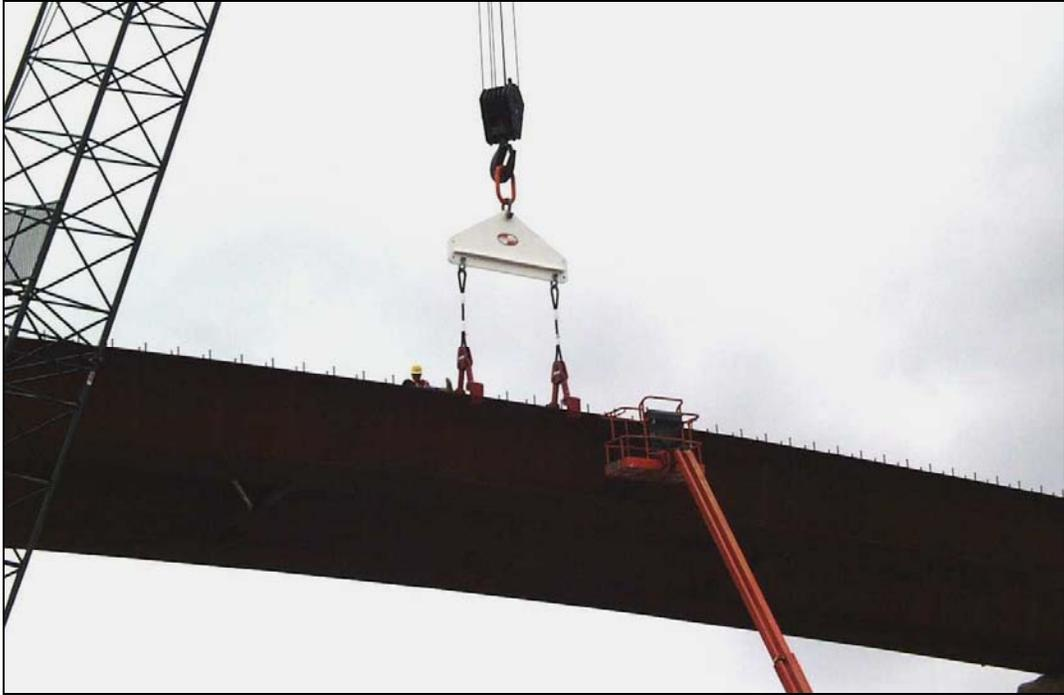
Figure 3.2 Crane Attachment
