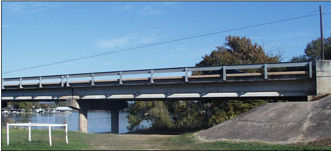
Figure 2.3 Photograph of Lake LBJ Bridge
