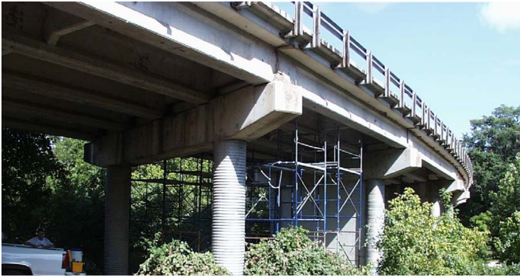
Figure 2.9 Photograph of Wimberley Bridge
