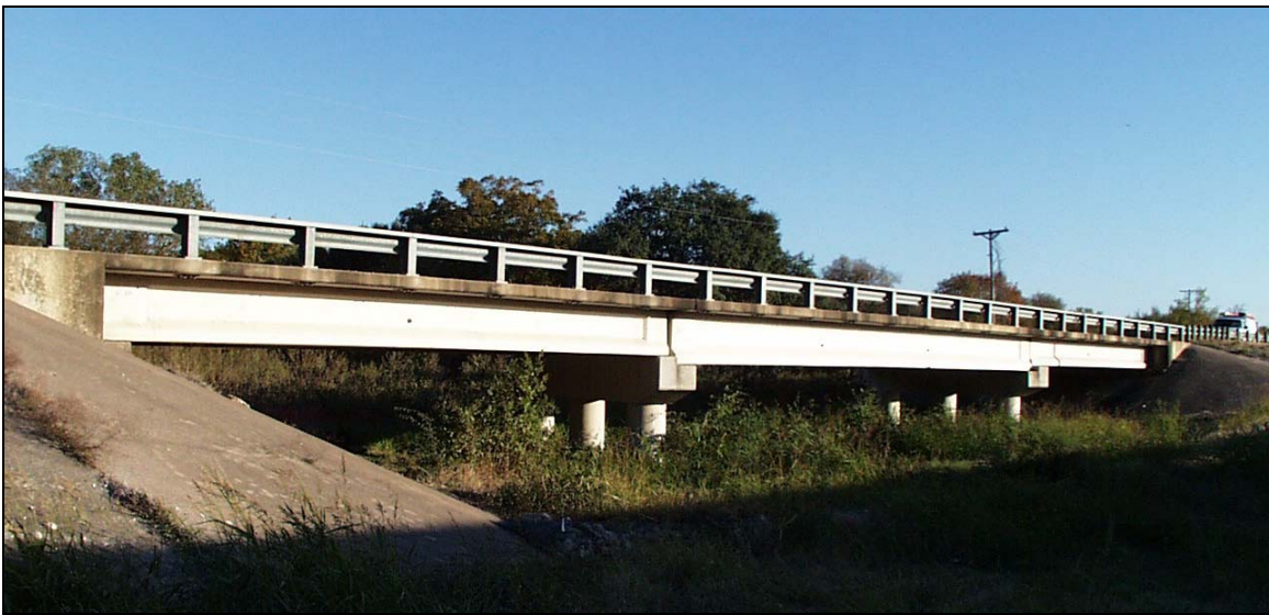
Figure 2.1 Photograph of Chandler Creek Bridge
