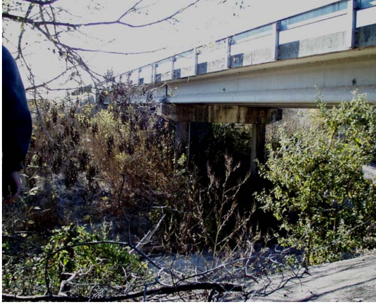
Figure 2.7 Photograph of Willis Creek Bridge
