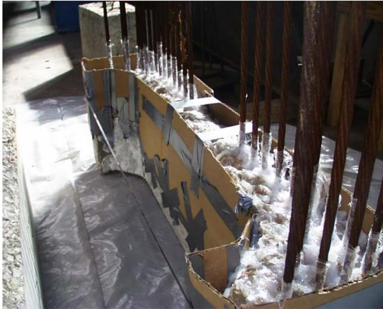
**Figure 3.24: Cardboard formwork used for front face**
