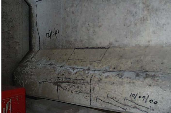
**Figure 6.15: Representative areas used for crack ratios, I-10 structure**
