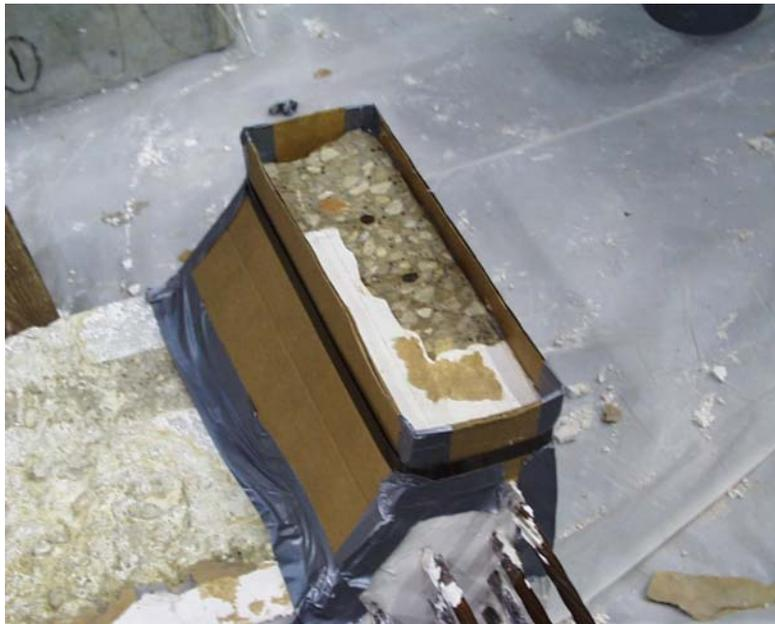
**Figure 3.26: Cardboard formwork for top of web**
