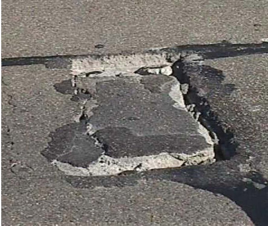
Figure G7: Punchout in AC overlay on CRCP (Photo ID #122)
