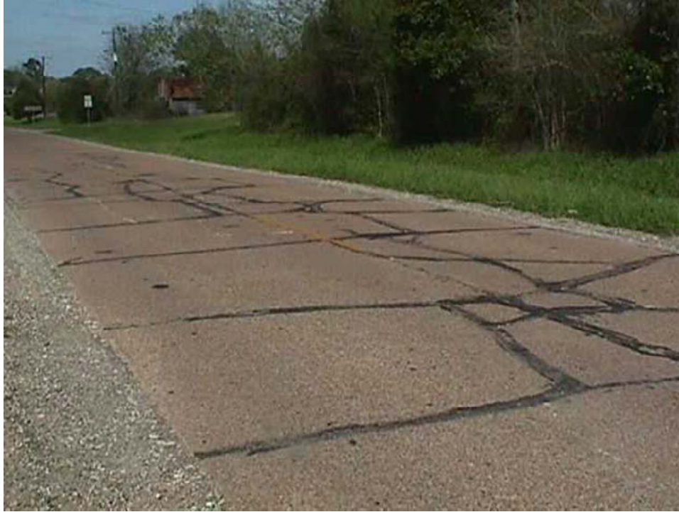
Figure G5: Random cracking in JCP section (CFTR 17602)
