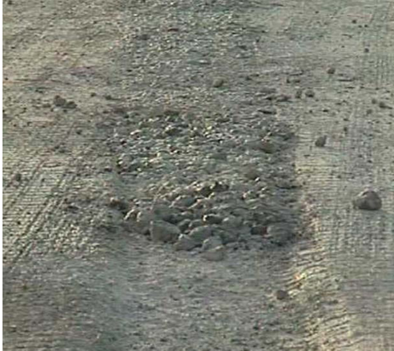
Figure G9: CRCP damaged by early traffic (Photo ID #127)
