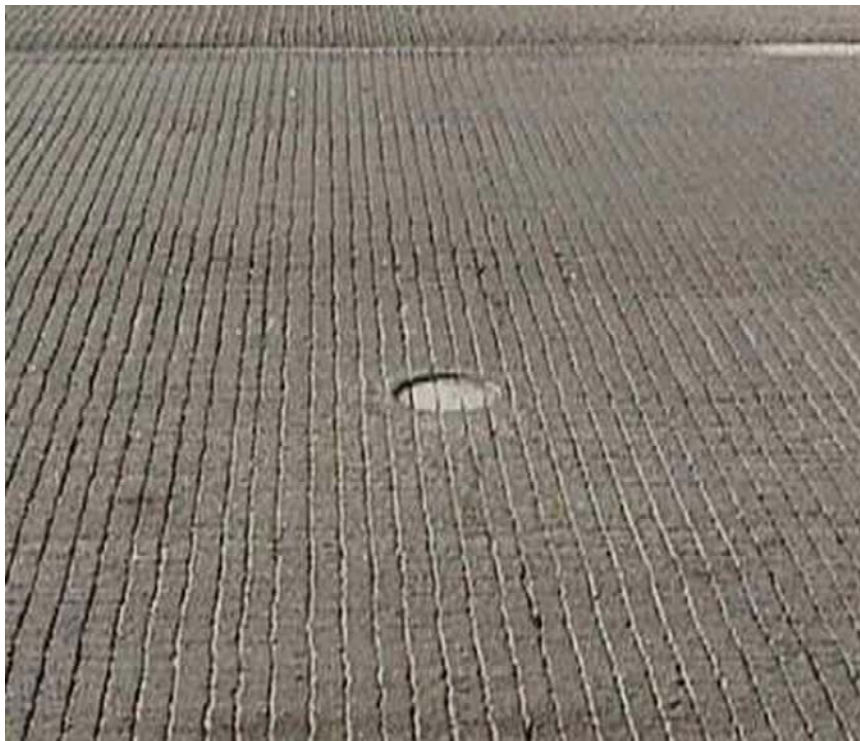
Figure G8: Core hole in newly constructed pavement
