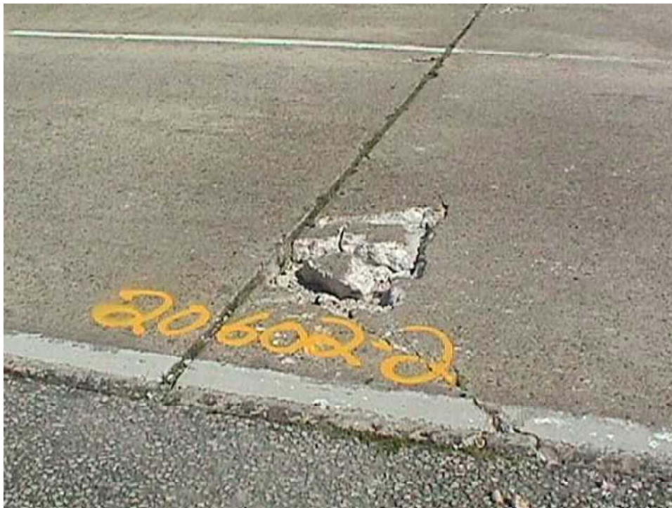
Figure G12. Possible corner break in JCP (CFTR# 20602)
