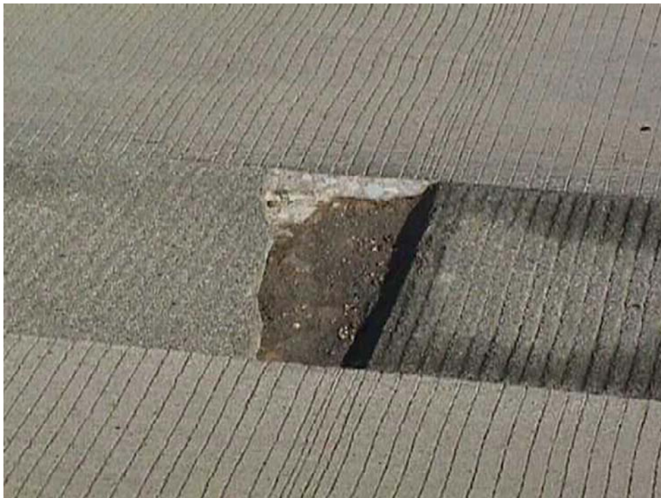
Figure G6: Punch-out from a Patch in CRCP (Photo ID #116)
