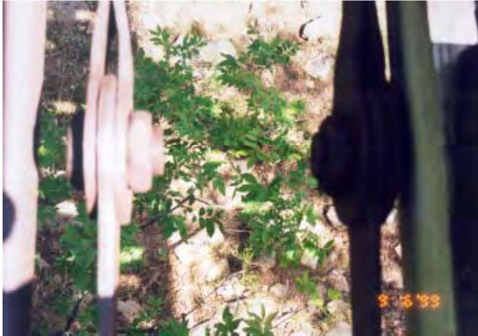
Figure A.11: Bottom chord joint L1
