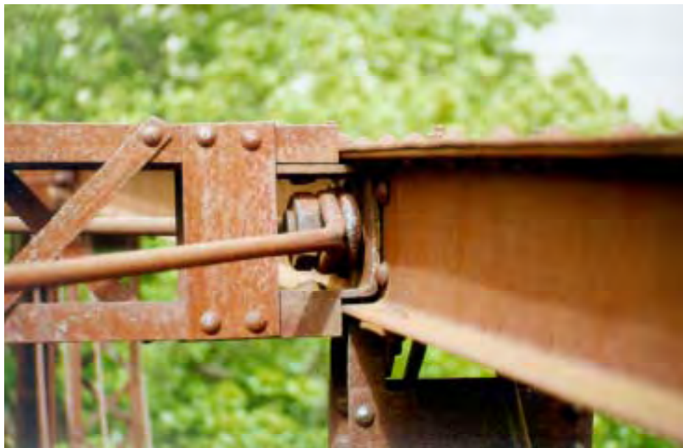
Figure A.16: Top bracing connection
