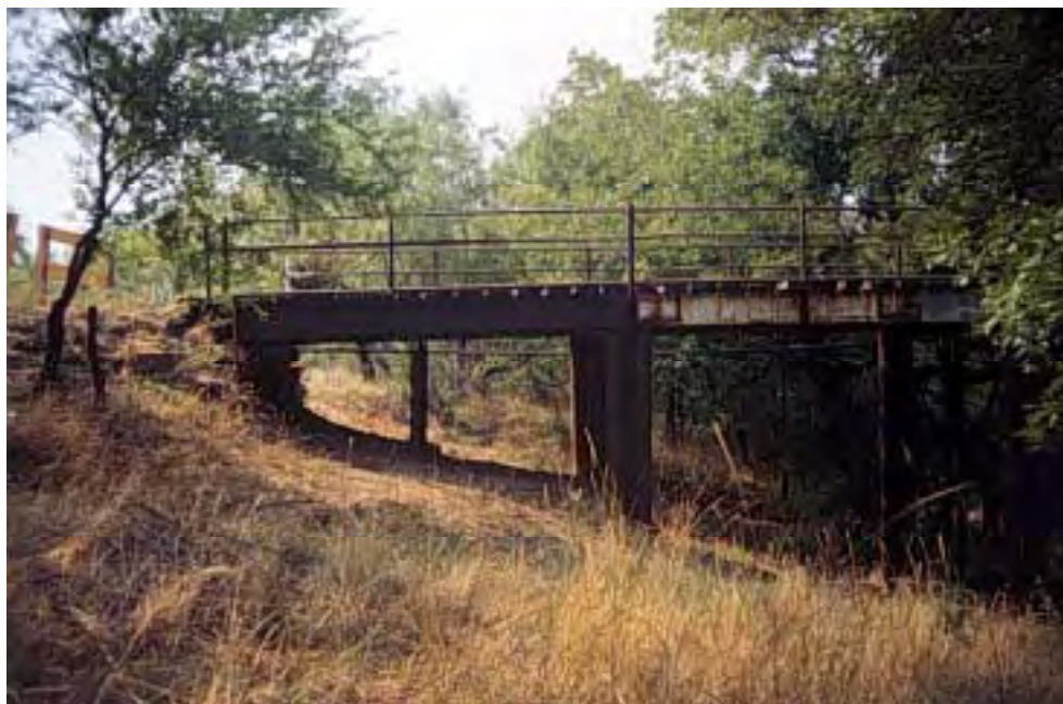
Figure A.2: South approach span
