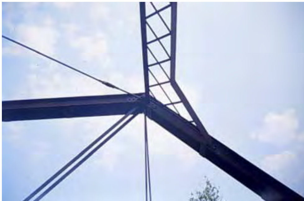
Figure A.14: Upper chord joint U1
