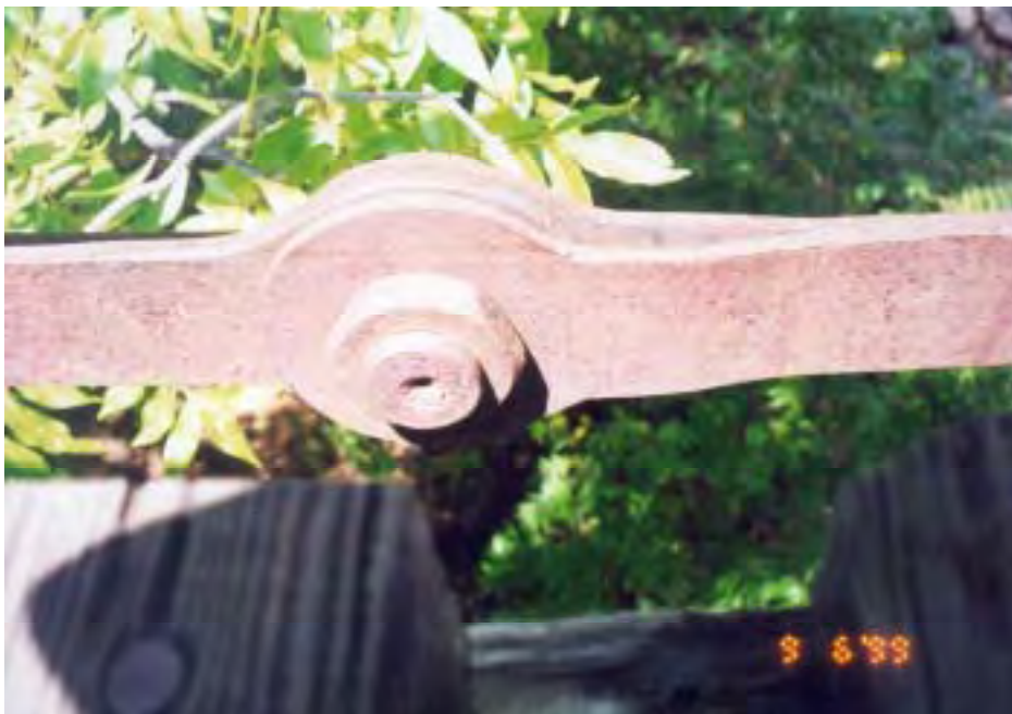
Figure A.12: Bottom chord joint L1
