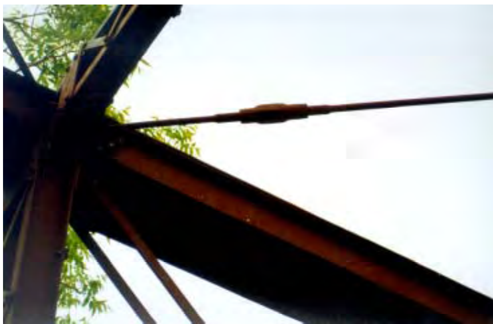
Figure A.22: Turnbuckle at a top bracing tension rod
