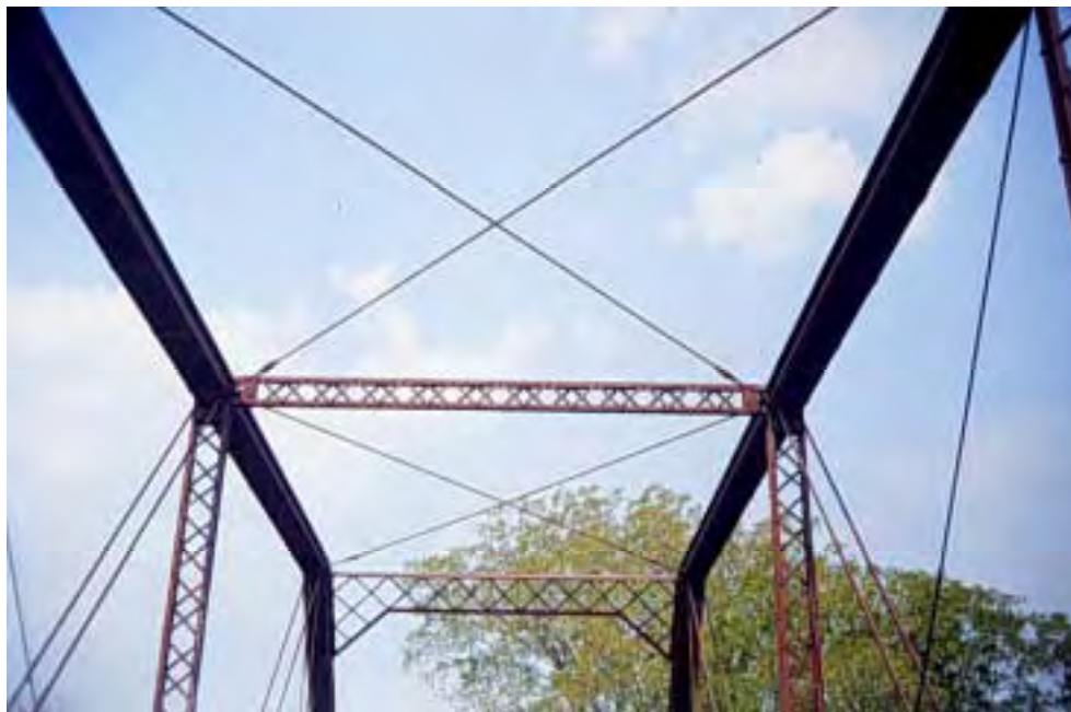
Figure A.21: Top lateral bracing system
