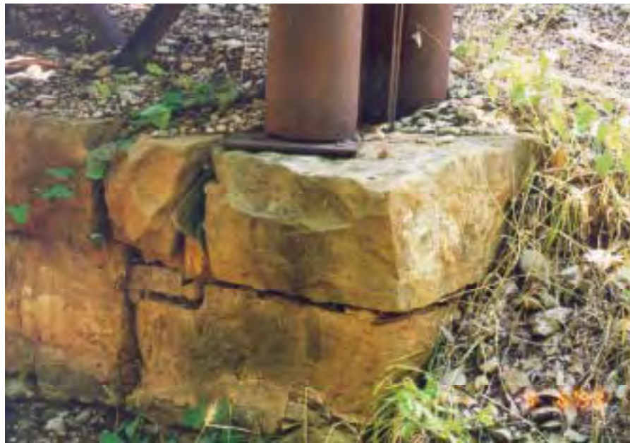
Figure A.33: Base of pipe column of metal bent for north approach span
