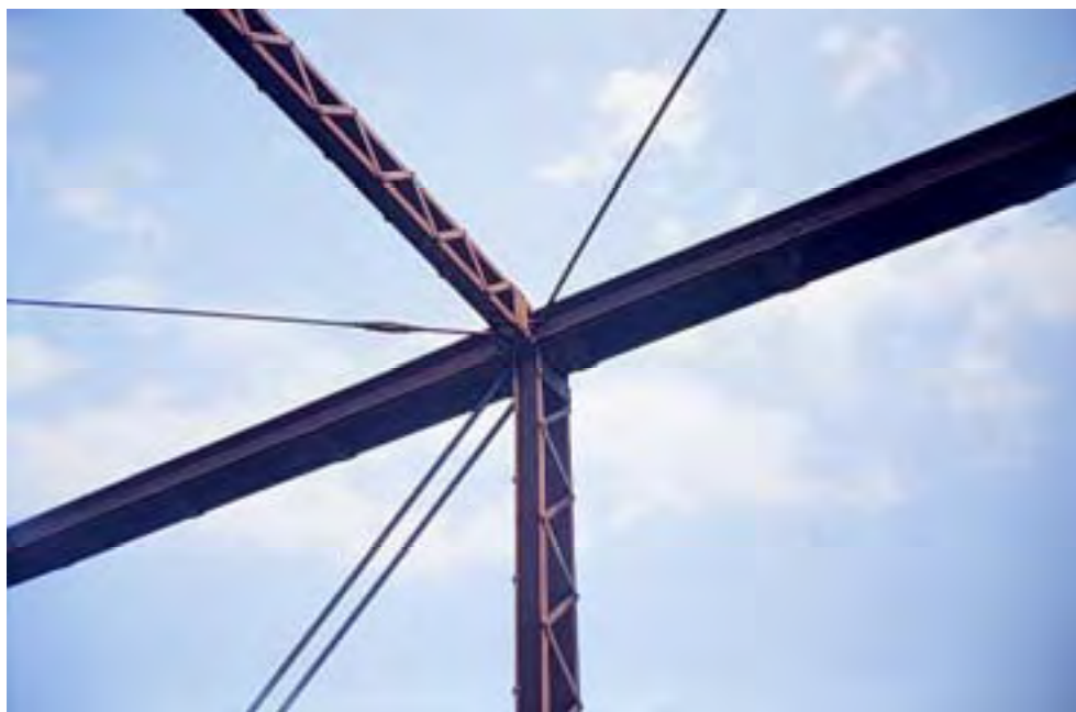
Figure A.15: Upper chord joint U2
