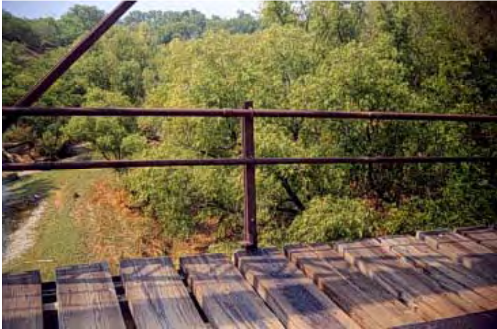
Figure A.23: Metal railing
