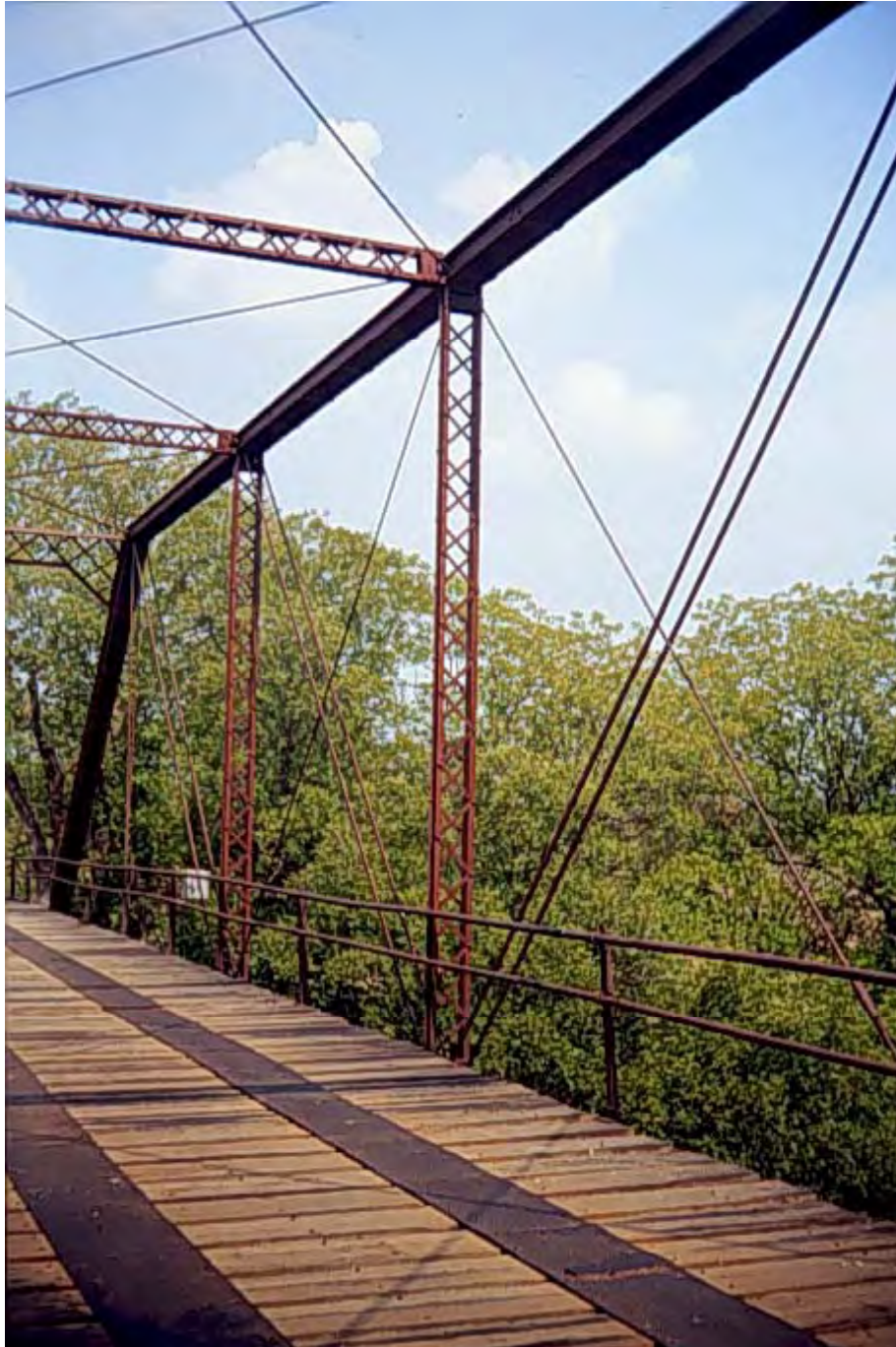
Figure A.6: Downstream truss
