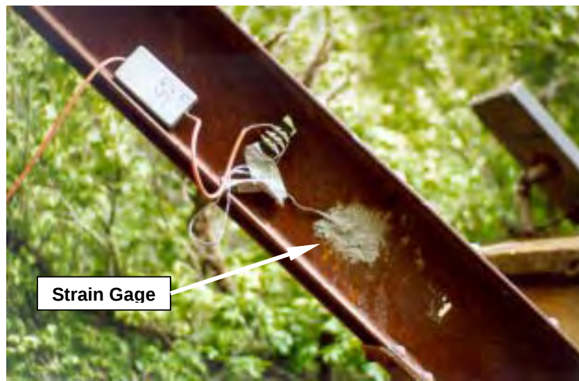
Figure 5.1: Typical strain gage installed on bridge member
