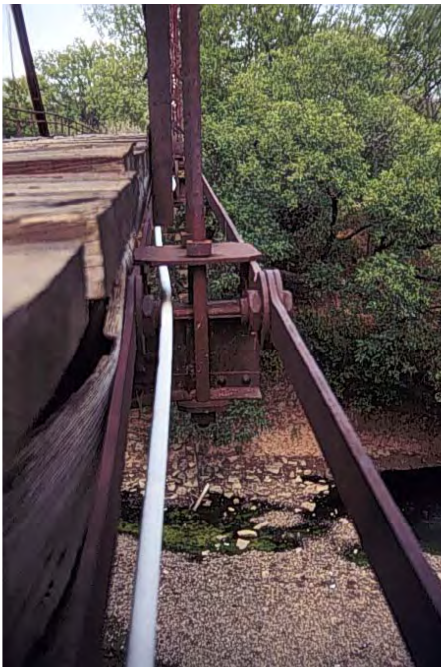
Figure A.9: Bottom chord joint L1
