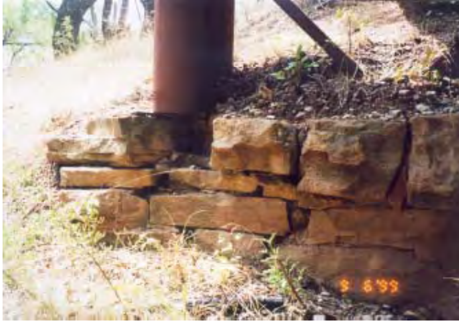
Figure A.32: Base of pipe column of metal bent for north approach span
