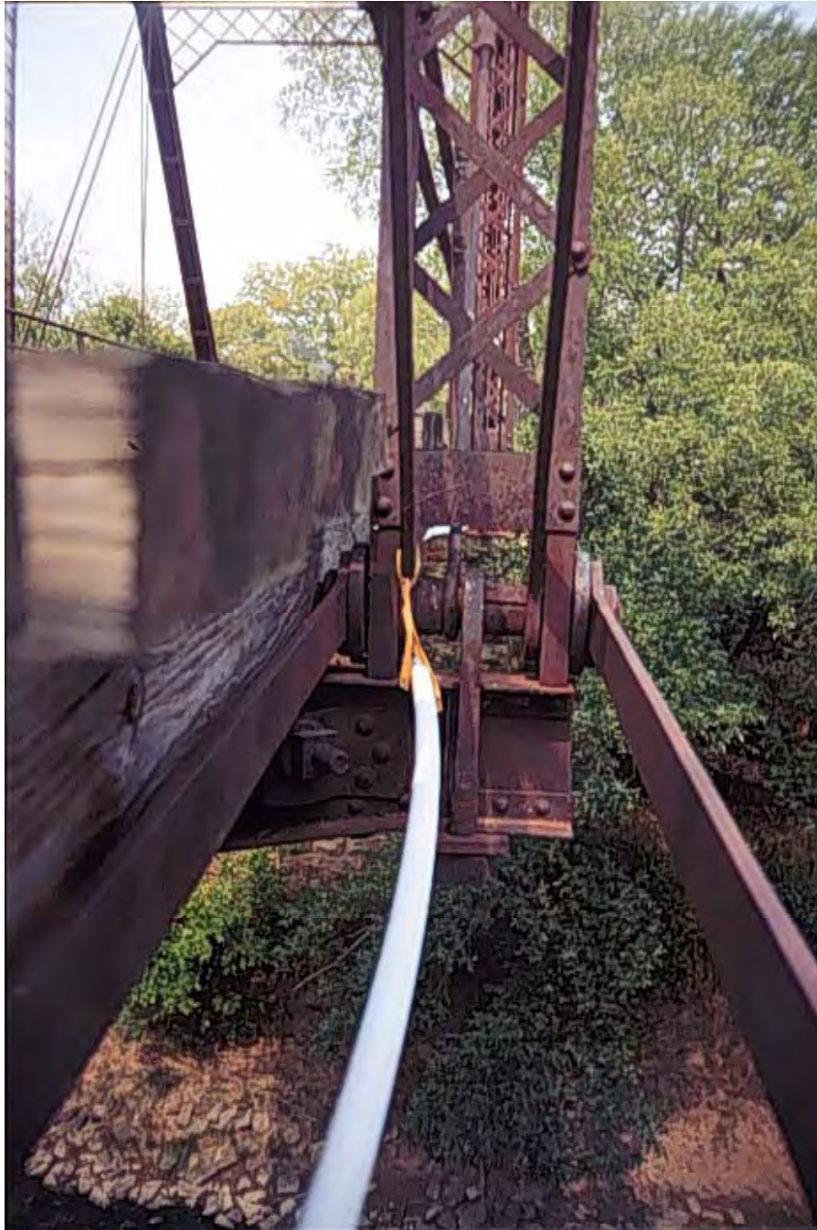
Figure A.10: Bottom chord joint L2
