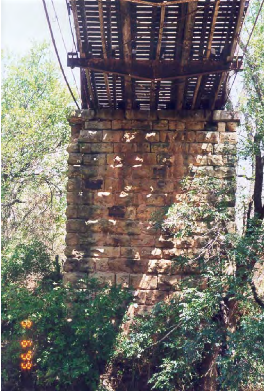
Figure A.19: North stone masonry pier
