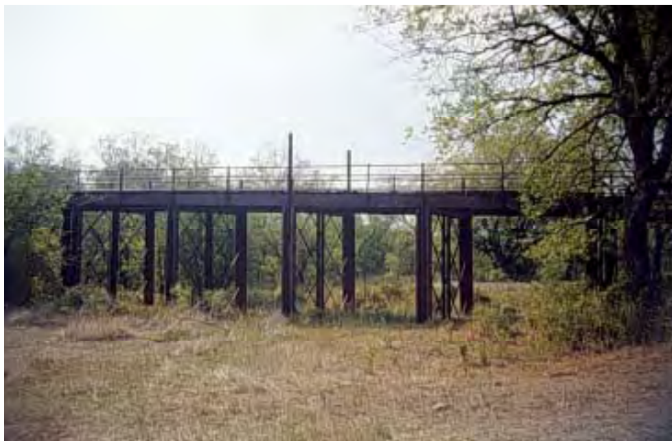
Figure A.4: North approach span
