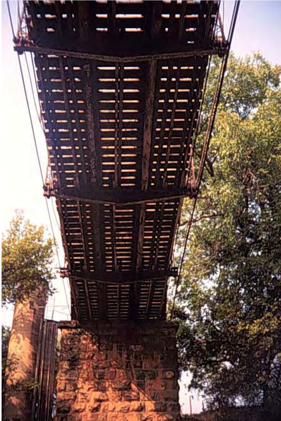
Figure A.20: South stone masonry pier
