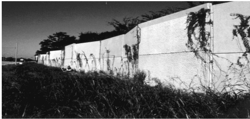
Figure 6.7 Example of fan-wall system (Austin District)
