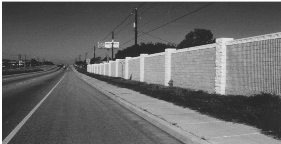
Figure 6.6 Constructed-in-place post-and-panel system (Austin District)
