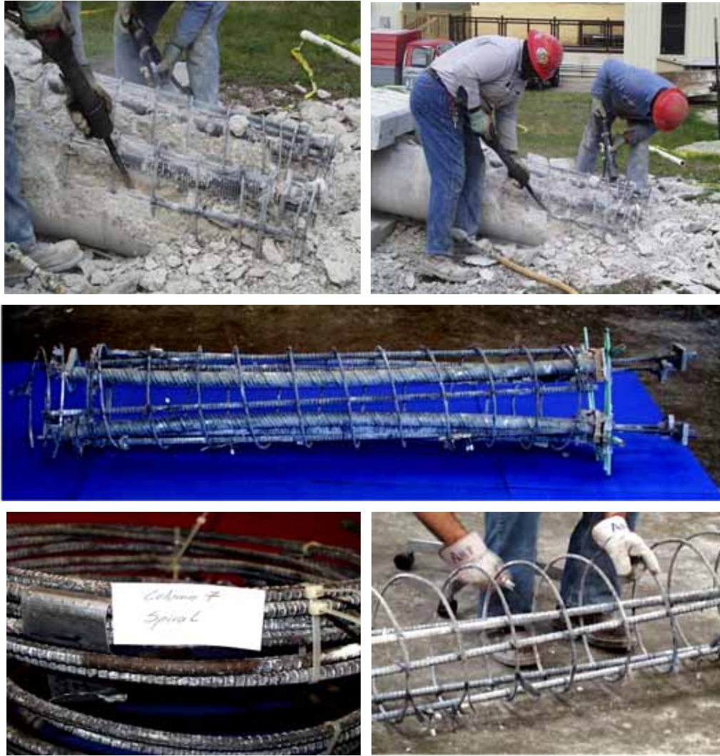
Figure 4.2 Concrete Removal and Reinforcement Dismantling 1
