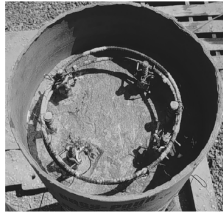
Gasket Around Post-Tensioning Bar Top of Column Prior to Capping
