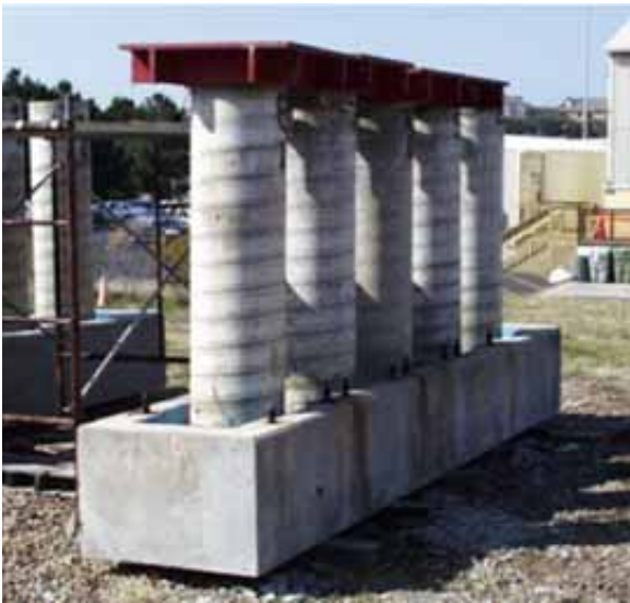
Figure 4.6 Specimen Condition at the End of Testing 1
