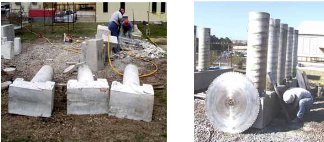
Figure 4.1 Saw Cutting of Column Foundation 1
