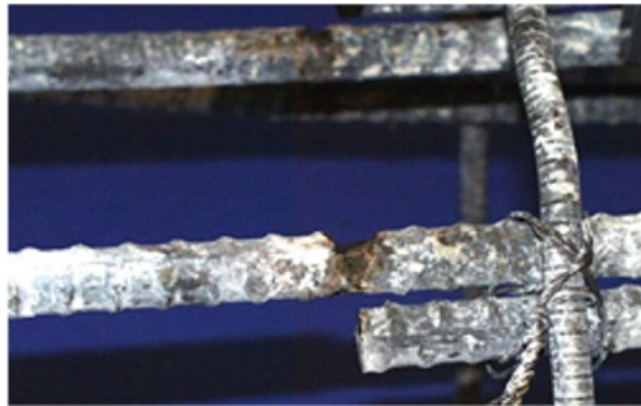
Figure 5.1 Typical Corrosion and Section Loss Found on Dowels at the Column-Foundation Interface 1
