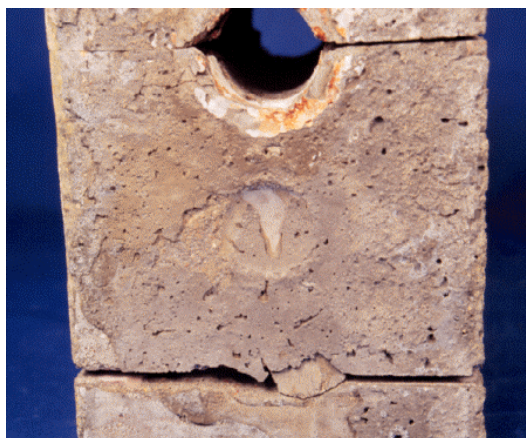
Figure 4.15 – Grout Infiltration Into Joint: Specimen DJ-S-L-CI-1
