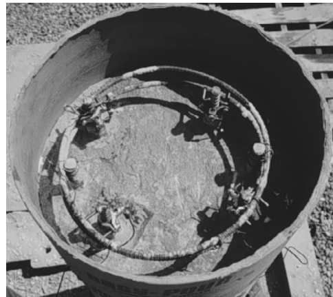
Top of Column Prior to Capping
