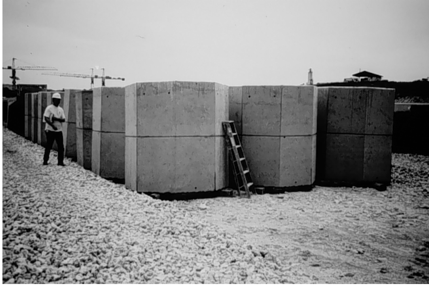
Figure 1.6 - Precast Bridge Pier Segments
