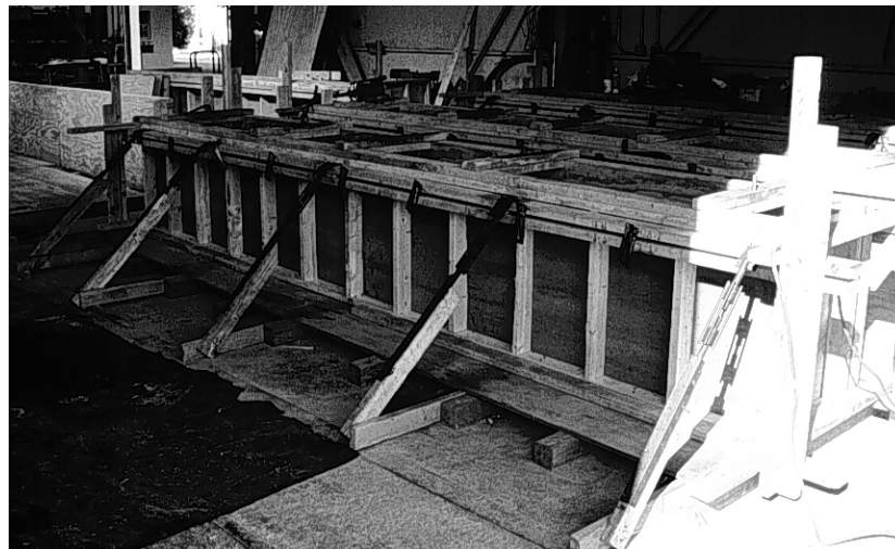
Figure 2.32 - Beam Formwork
