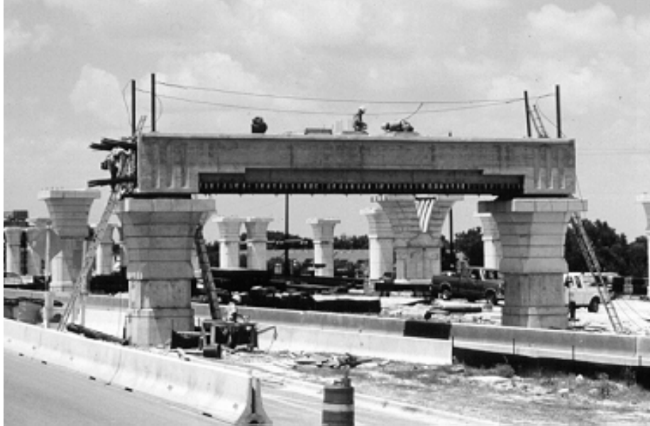
Figure 1.7 - Post-Tensioned Straddle Bent
