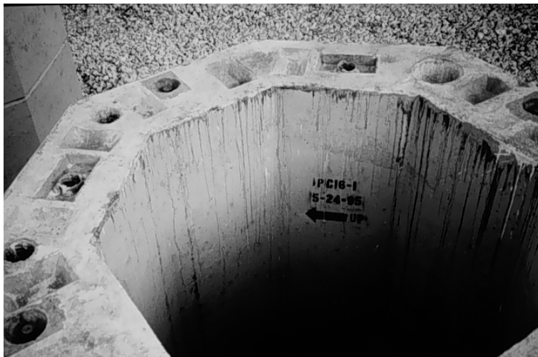
Figure 1.5 - Precast Bridge Pier Segment Close Up
