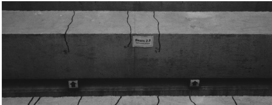
Figure A.42 - Crack Pattern for Specimen 2.8
