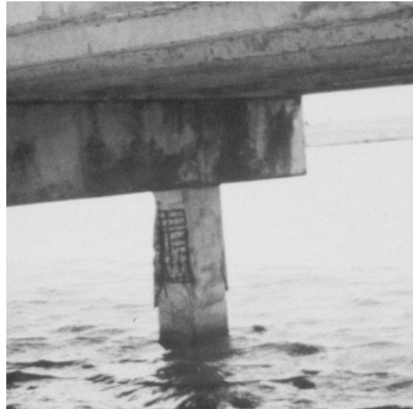
(b) Coastal Saltwater Exposure “Attack from Below”
