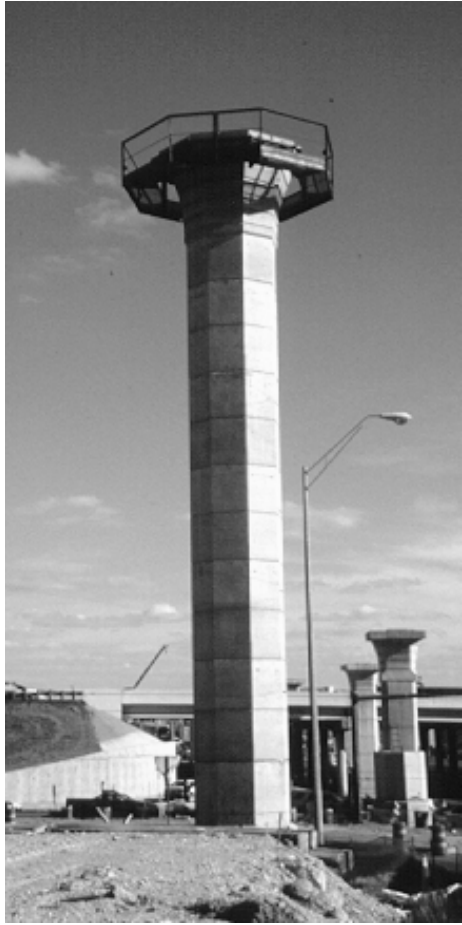
Figure 1.4 - Post-Tensioned Precast Segmental Bridge Pier
