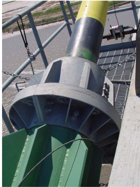
Figure 1.8 Freyssinet Damper
