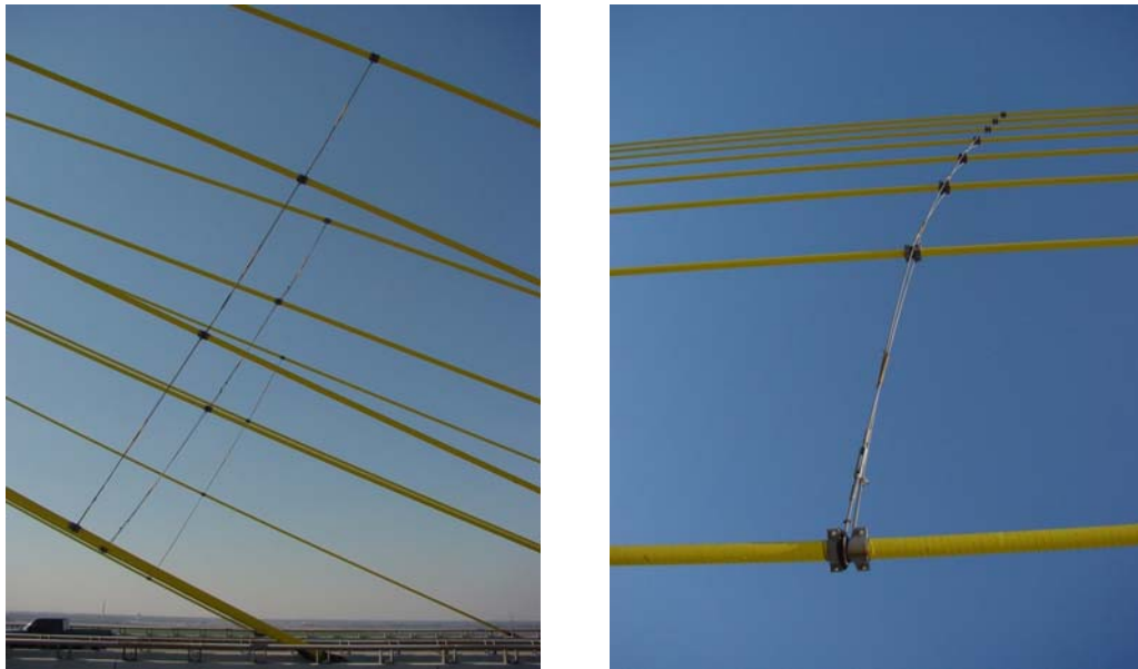
Figure 1.6 Cable Restrainers
