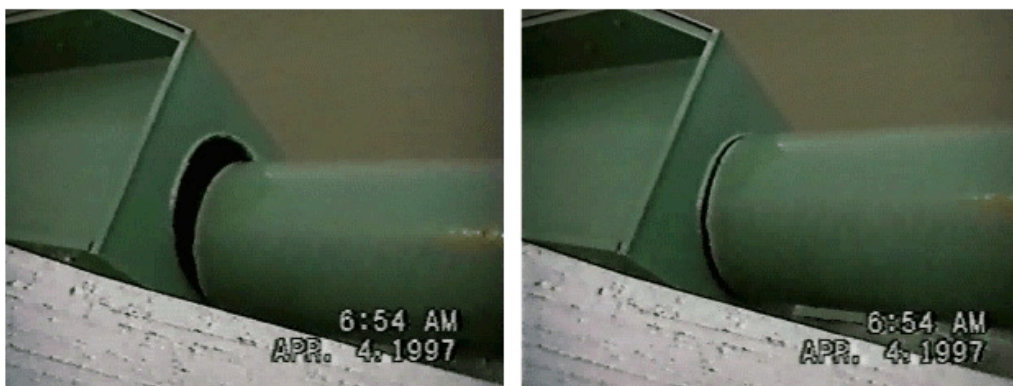
Figure 1.5 Broken Guide Pipe – Fred Hartman Bridge
