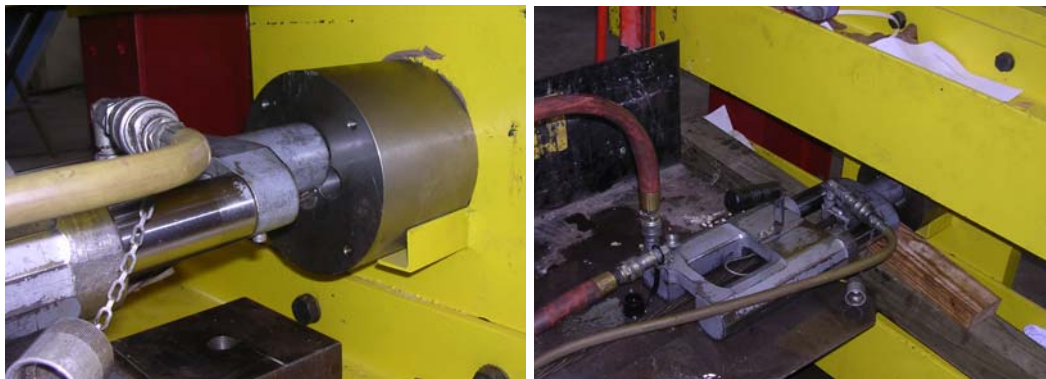
Figure C.11 Stressing of Strands Individually with Hydraulic Ram
