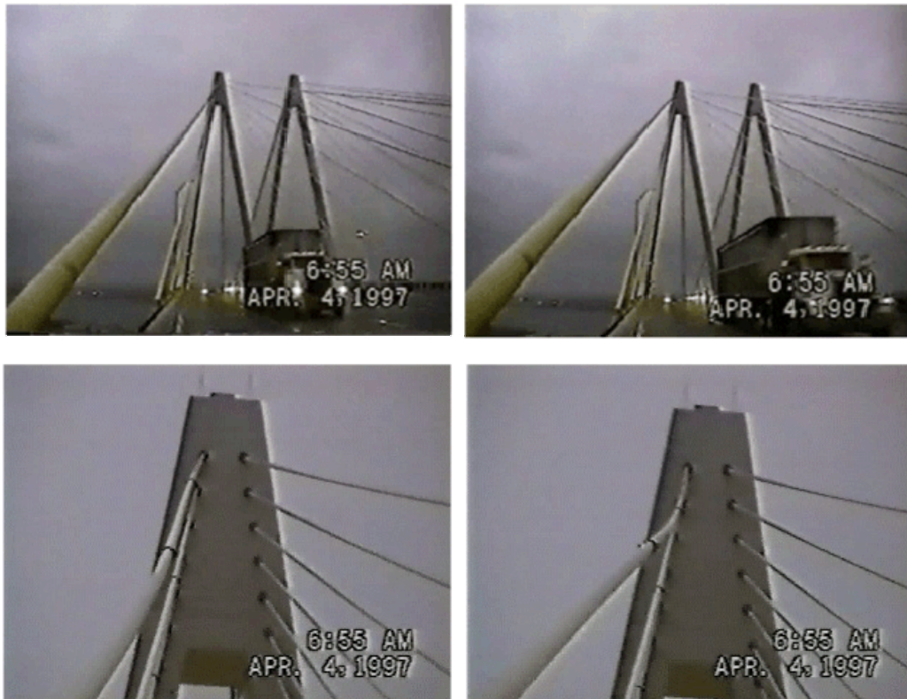
Figure 1.4 Stay Cable Vibrations – Fred Hartman Bridge
