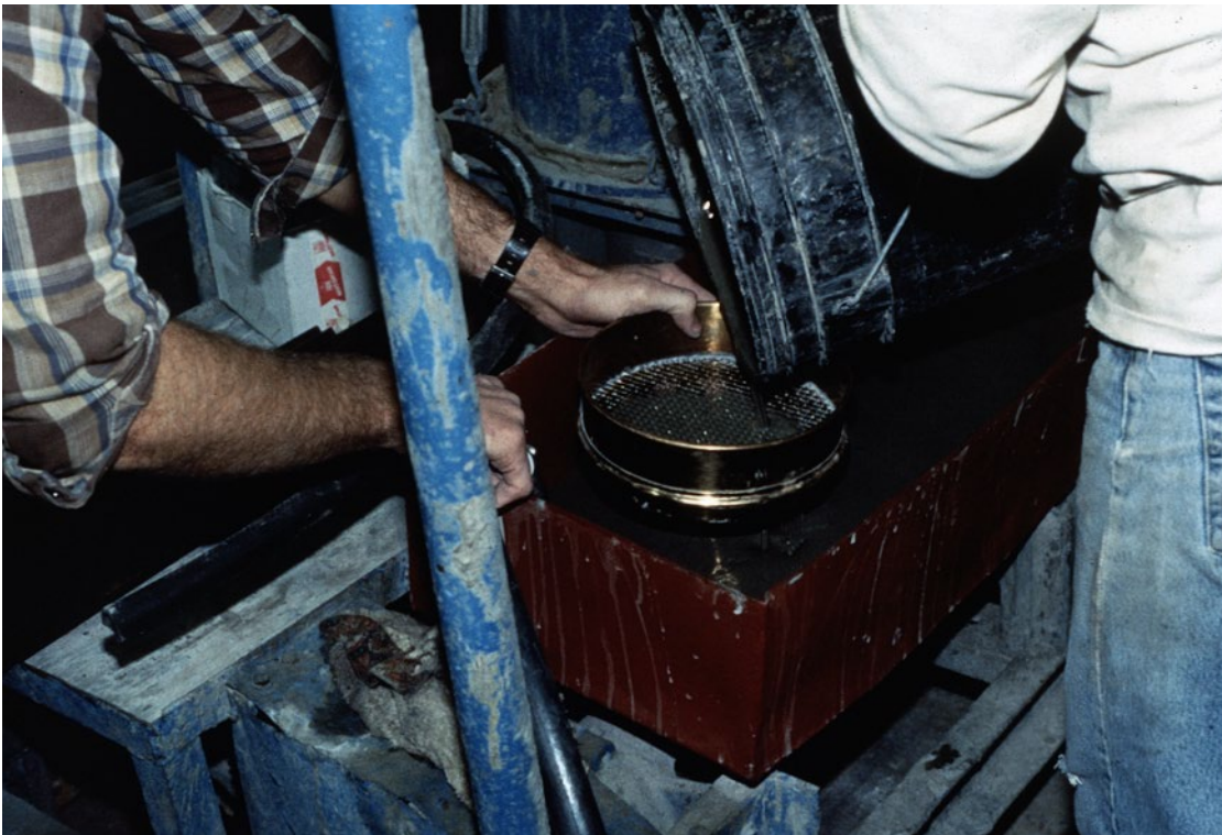
Slide 88. Straining grout.
