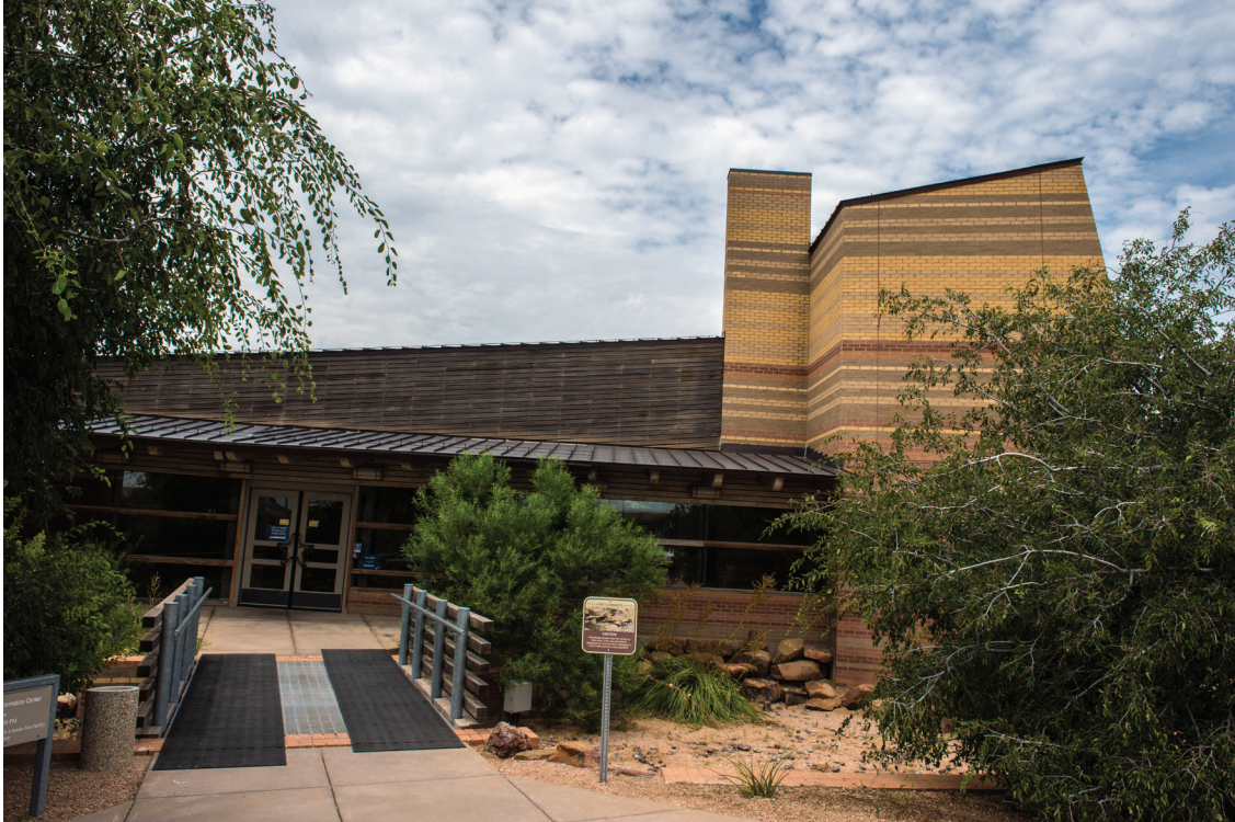
Figure 3-9. Main Entrance to the Amarillo Travel Information Center.
