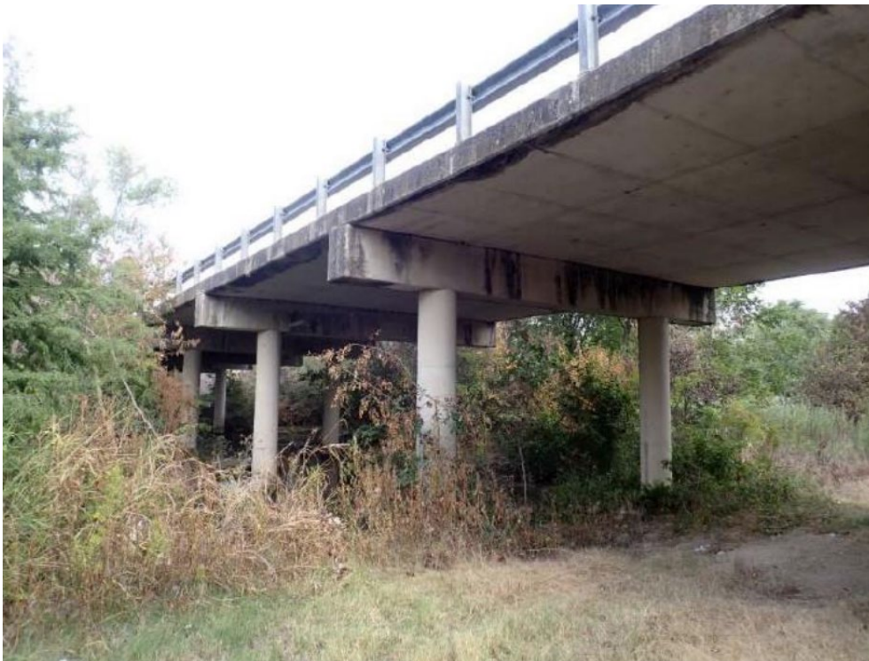
Figure 3-1: Photograph of flat slab concrete bridge
