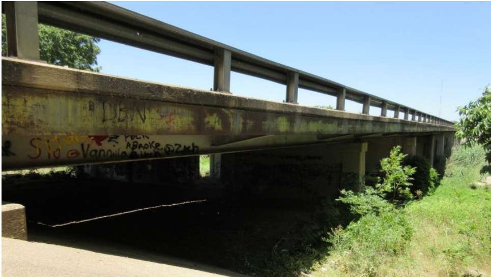
Figure 3-11: image of bridge
