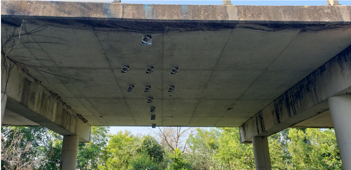
Figure 3-2: Attachment of HCPTs at midspan on the bridge slab soffit.
