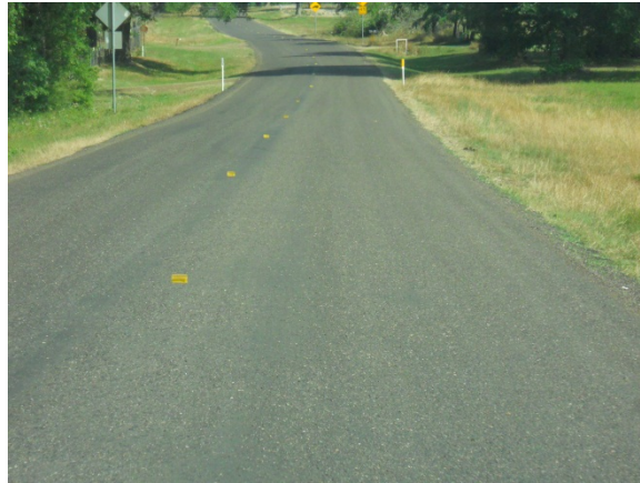
Figure 15. Temporary marking placed at the road centerline
