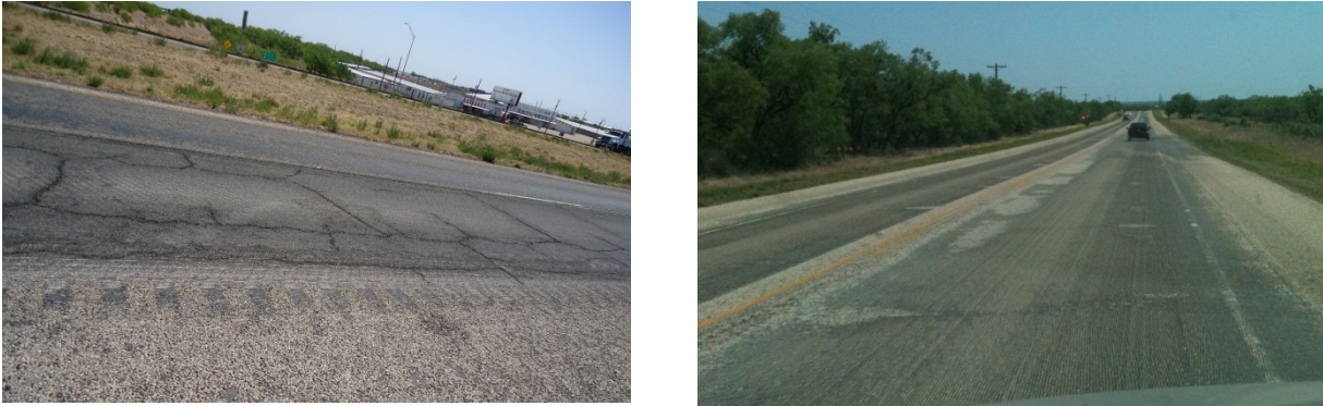
Figure 3. Full-lane width milling to remove the deteriorated surface layer
