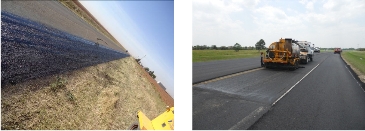
Figure 6. Tack coating over full-lane width with regulated Asphalt Distributor
