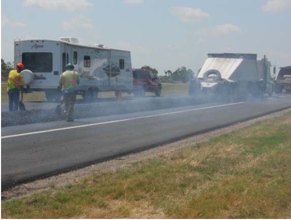
Figure 7. Placing the mix on the surface with belly dump and end-dump truck.
