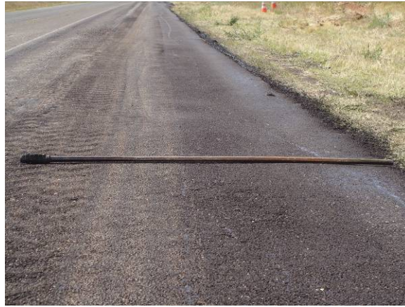
Figure 14. A visual check with a rod or straight edge to check on the cross slope
