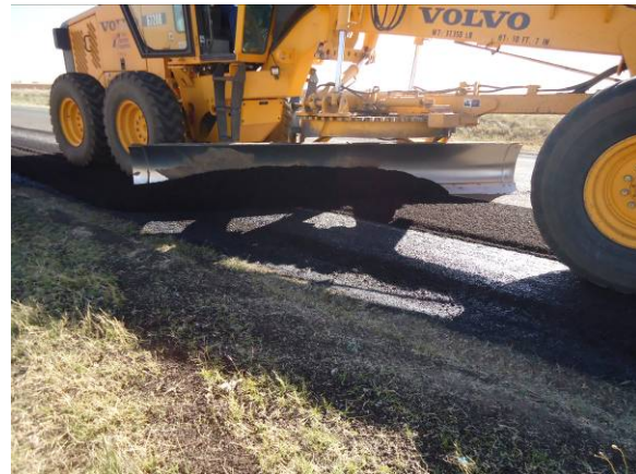
Figure 10. Leveling up the mix with blade
