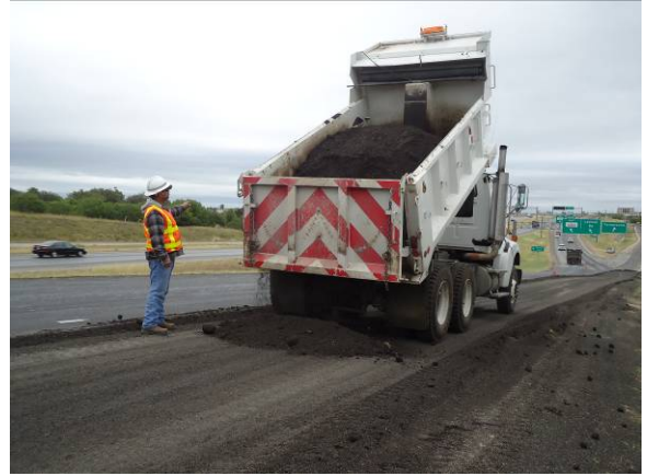
Figure 7. Placing the mix on the surface with belly dump and end-dump truck.
