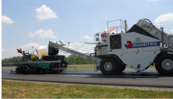
Figure 9. MTV used for hot mix patching operation
