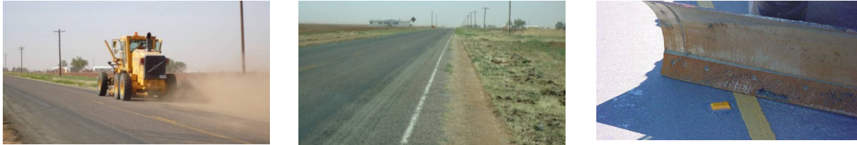
Figure 4. Vegetation, soil and marker removal along the side of the worked lane
