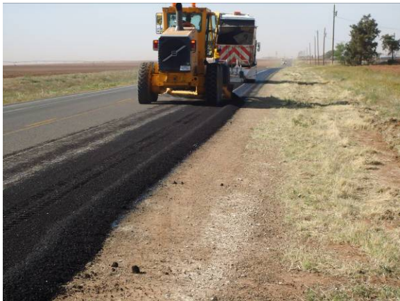
Figure 10. Leveling up the mix with blade
