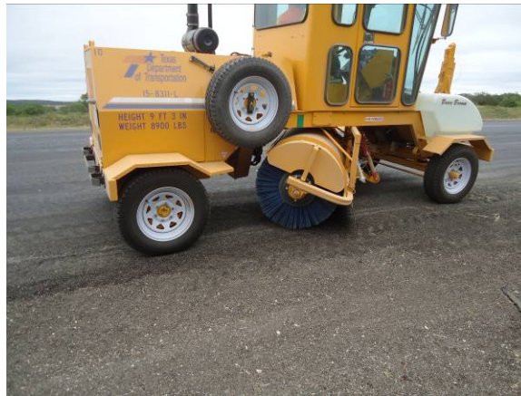
Figure 5. Surface dry cleaning prior to patching using a broom machine
