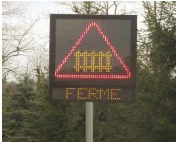
Figure 2-9 VMS in Protected Crossing (Ref. 2-6)
