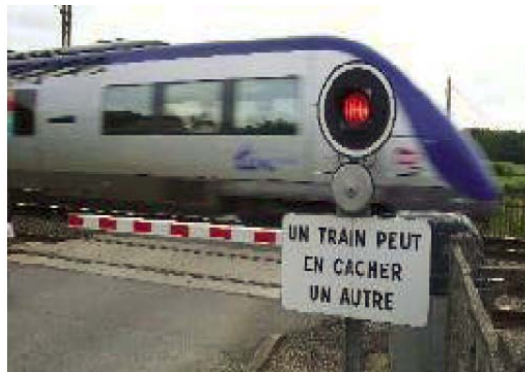
Figure 2-7 Example of Active Protection in France
