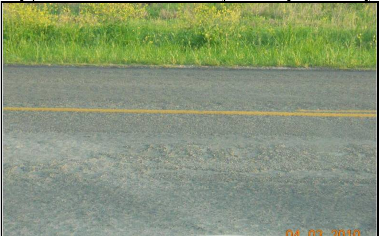
Category 5: FM 758 from 2.7 miles East of SH 46 to SH 123 (base repair and poor ride)
