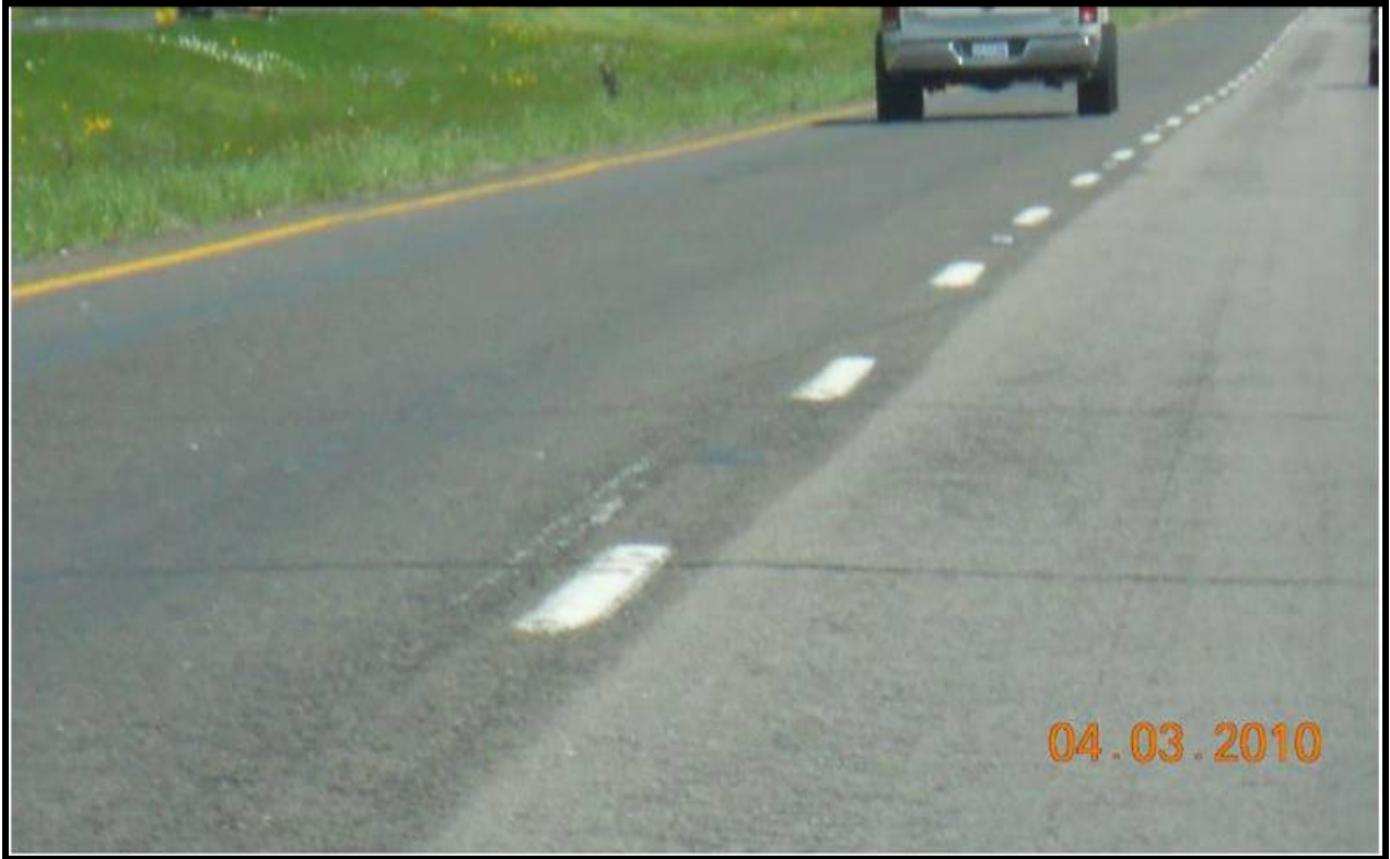
Category 1: Northbound US 59 from San Jacinto county line to FM 3460
