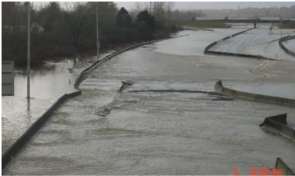
Figure 1.2. Sliding and Overturning of TCTBs during a Flood Event.
