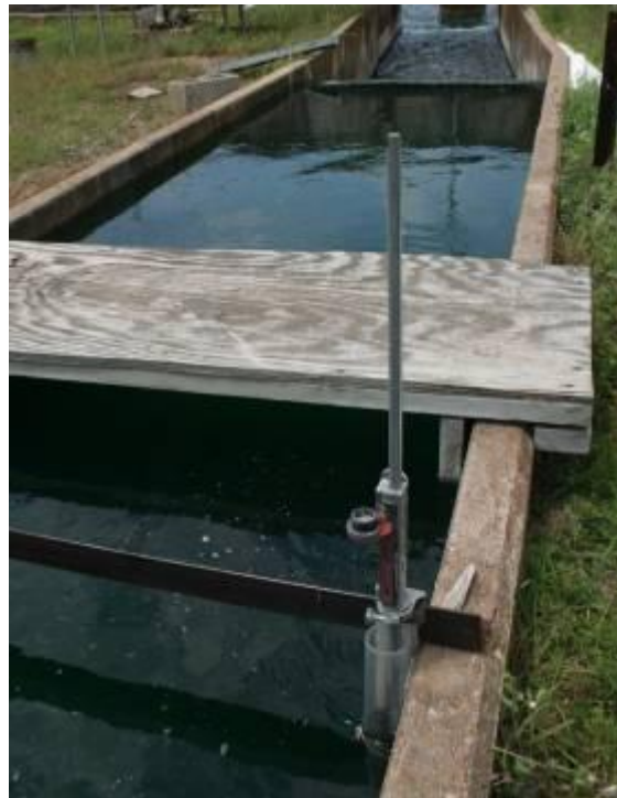
Figure 3.13. Weir Point Gage.
