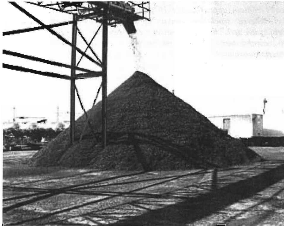
FIGURE 2 Crumb Rubber Produced Using Ambient Grinding
