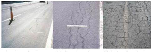
Low Severity: Few connecting cracks with no spalling; cracks are not sealed.
