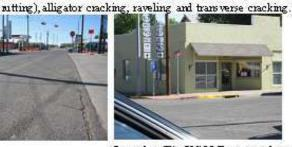
Location (B and C): SH 188 Severe rutting and raveling. Also, alligator and longitudinal cracking.
