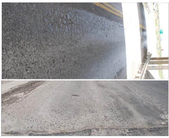
Figure 7.14 – Alligator cracking and Surface Rutting along US 83 Underpass.
