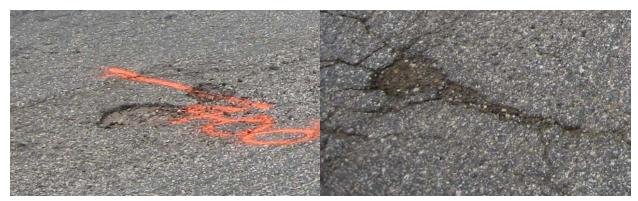
Figure 5.6 - Cracking Resulting in Potholes on SH 49.
