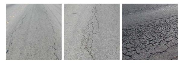
Figure 2.7 - Fatigue or Alligator Cracking on Asphalt Pavements.
