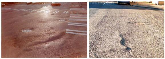
Figure 2.6 - Shoving on Asphalt Pavements.
