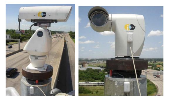
(a) Mechanical device installed on the pole in Fort Worth
