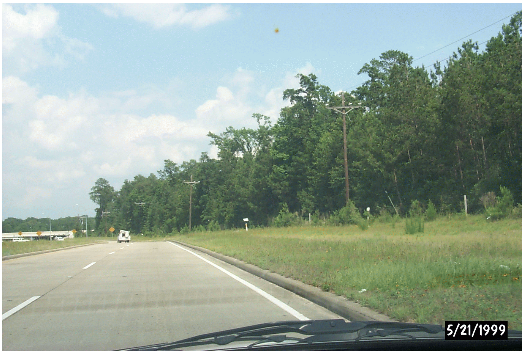
Figure A4. Photo of Curb Showing Absence of Shoulders Along K6 Lane Near the IH45 Junction.
