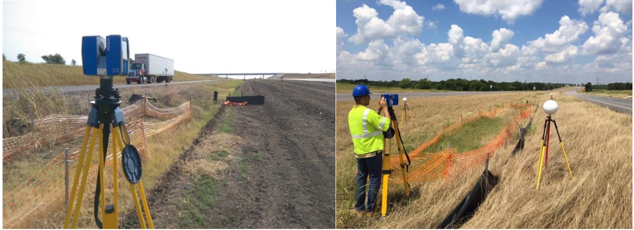
Figure 27: LiDAR investigations at Test section 3
