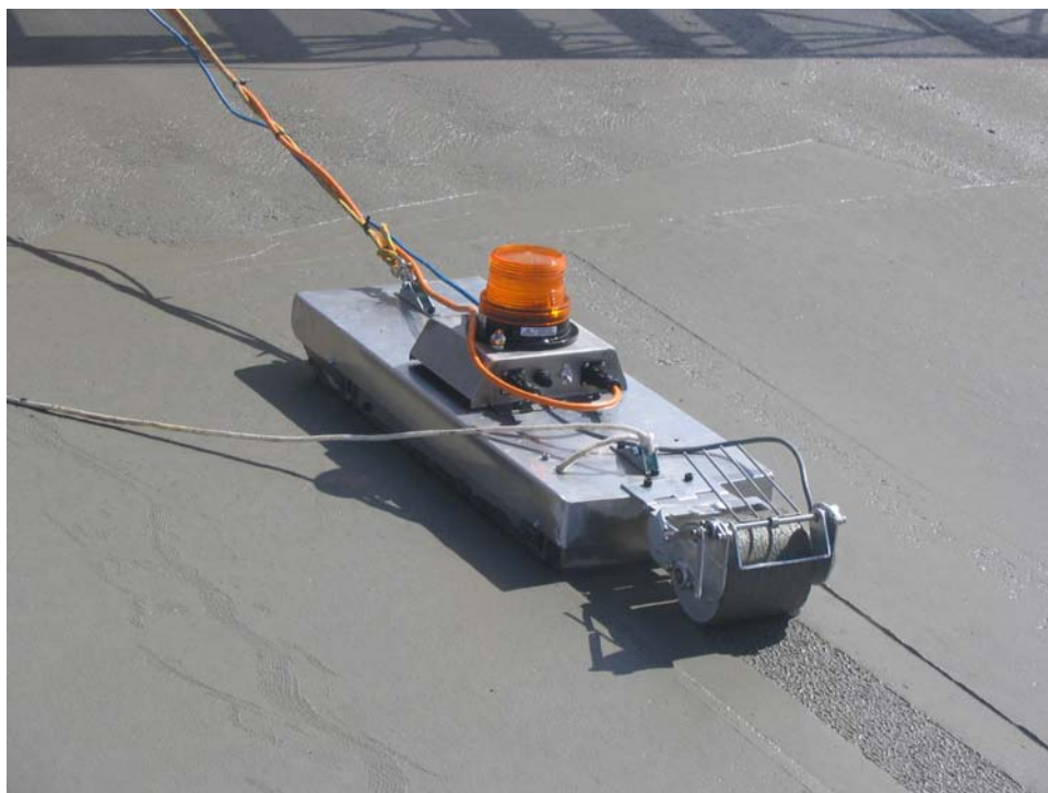
Figure 2 Sliding Profiler on El Paso Tests after Hwy 360 Adjustments
