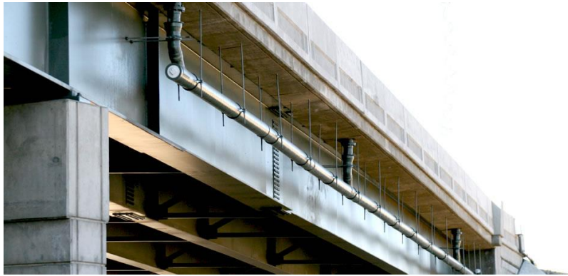
Figure 5.7 Pipes Sloped Along Bridge Profile Grade (Hennegan, 2021)
