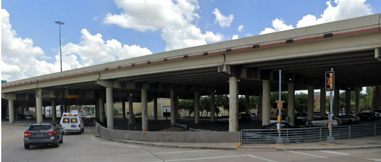
Figure 5.2 Free-fall Discontinues Over a Roadway in Houston
