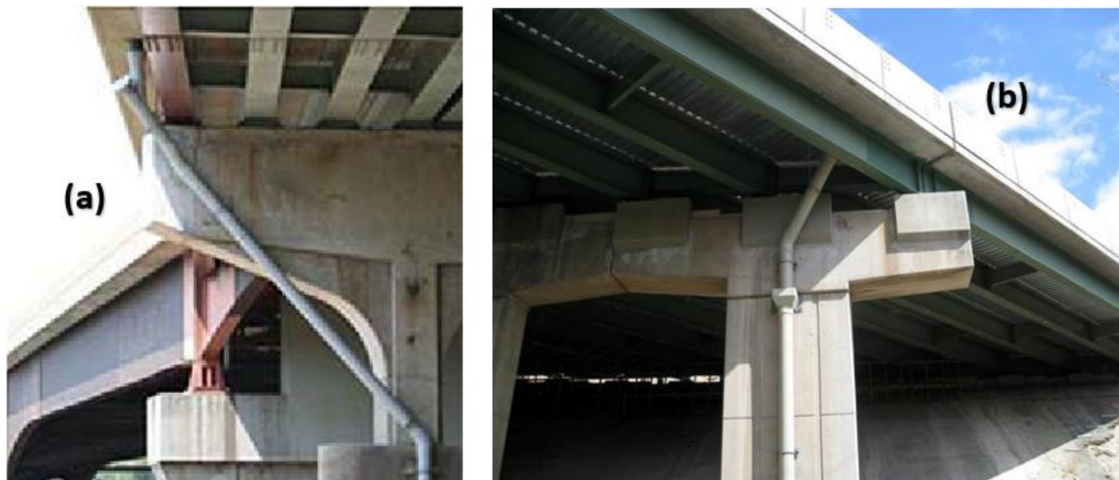
Figure 5.1 Hung system Aesthetics: (a) Aesthetically Displeasing System (b) Aesthetically Pleasing System (Yildiz Dak, 2010; NJDOT, 2011)
