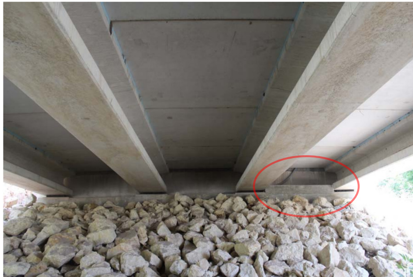
Figure 6.1 Shear key on bridge bent cap
