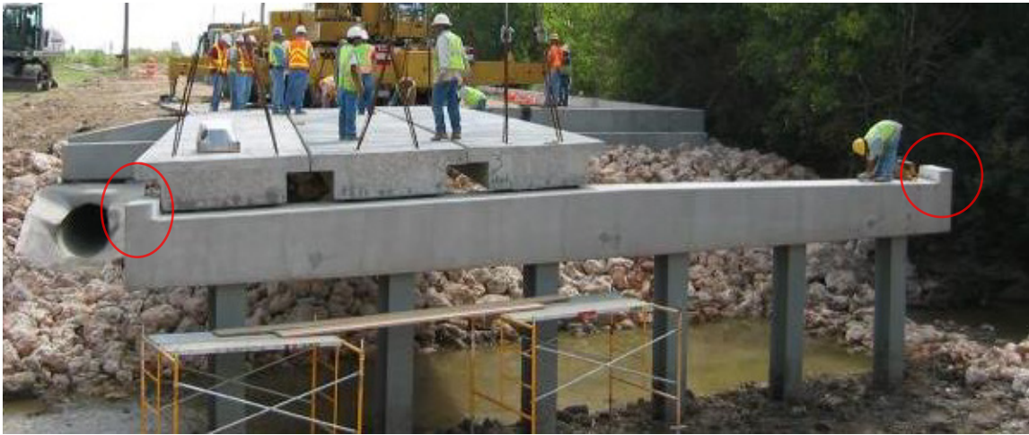
Figure 6.4 Earwall on bridge
