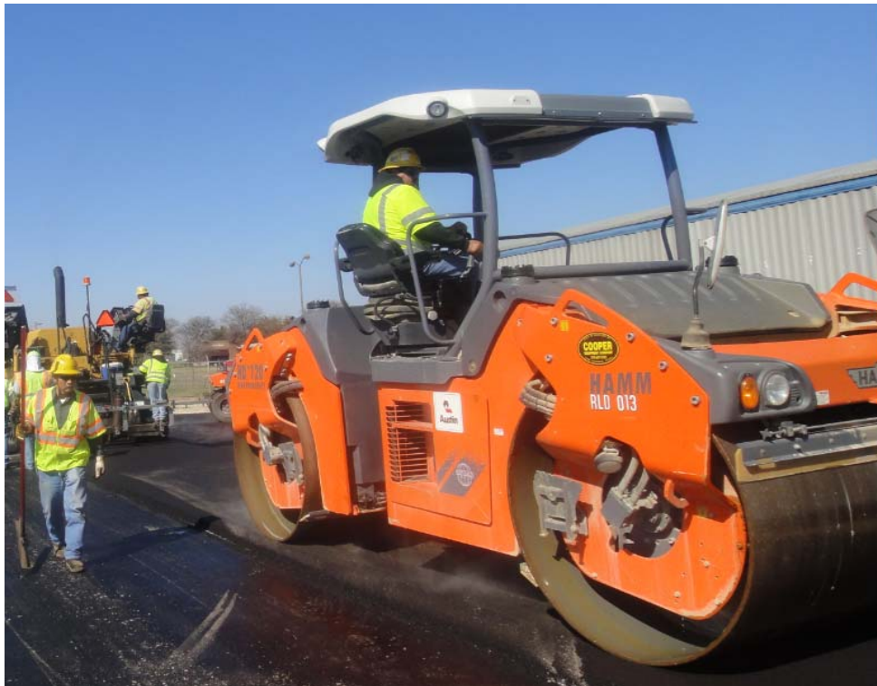
Figure 5.5. Breakdown Roller (a Combination of Vibratory and Static Passes Were Used).
