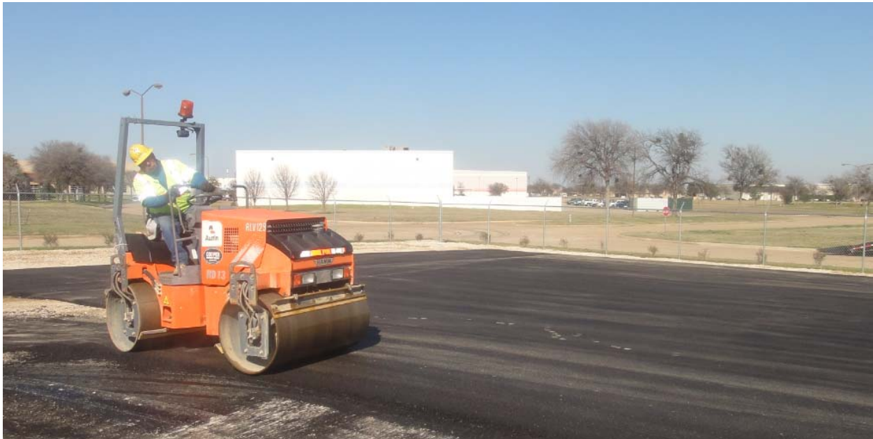
Figure 5.7. Finishing Roller for Edges and to Give a Smooth Finish.
