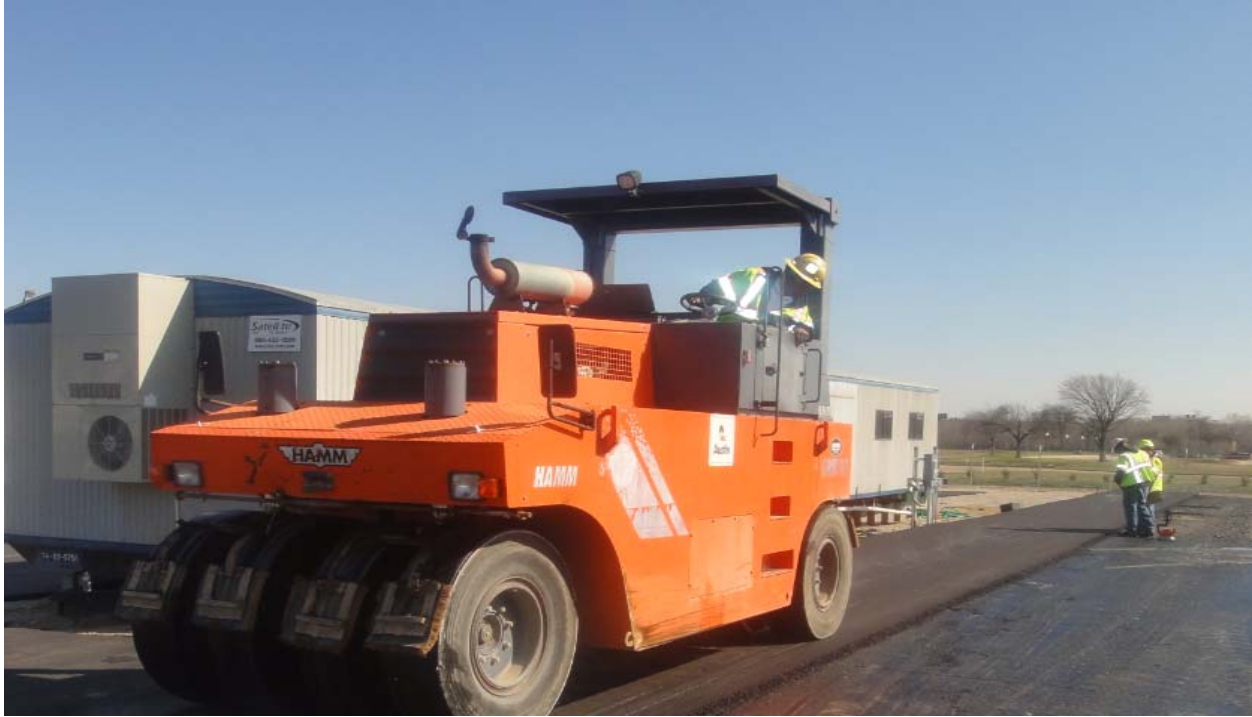
Figure 5.6. Multiple Passes of the Pneumatic Roller.
