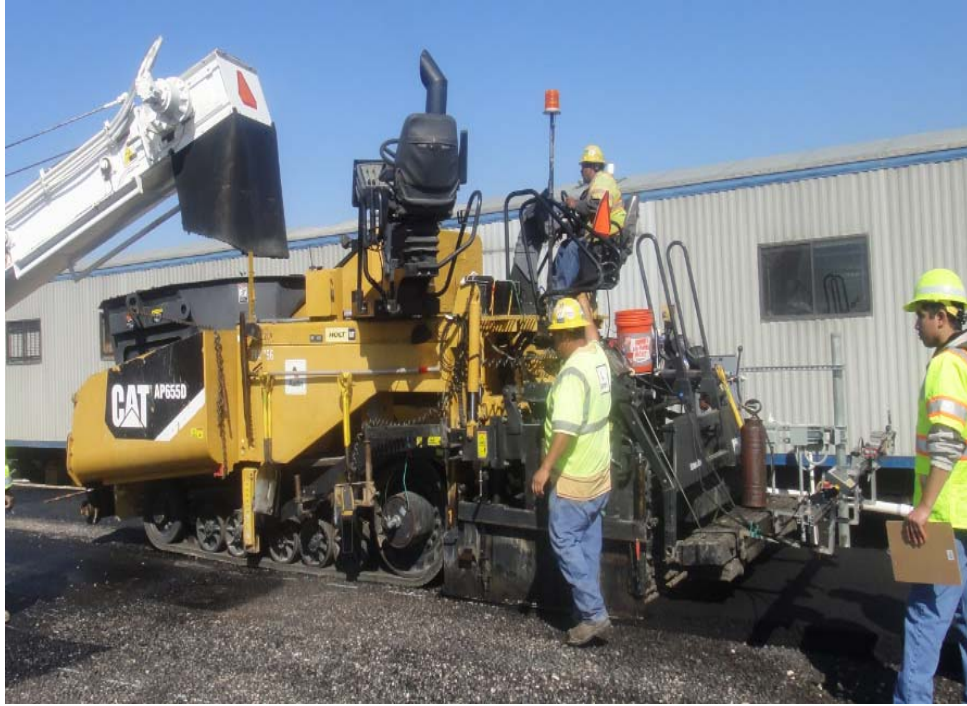
Figure 5.4. Paver with the Pave-IR Bar Attached.
