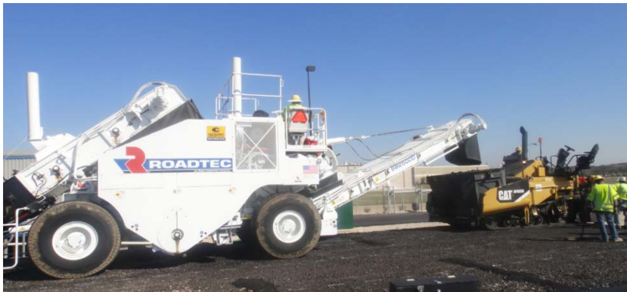
Figure 5.3. Shuttle Buggy Used on All HMA Placement to Ensure Thermal Uniformity.
