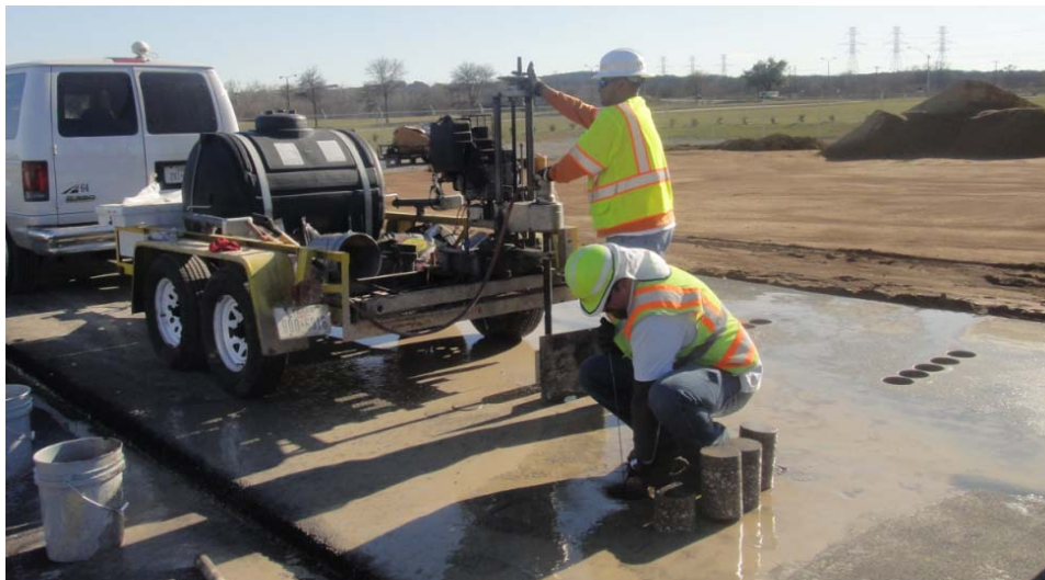
Figure 5.13. Section Coring Close to the Transition Zone between Sections.
