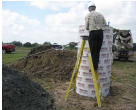
(b) Check of Angle for Dywidag Bars
