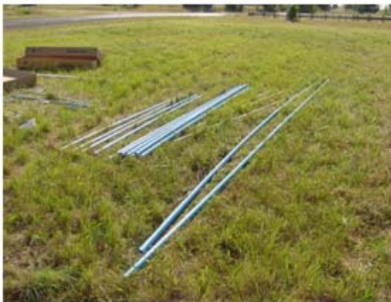
(a) Inclinometer Casings (Blue)
