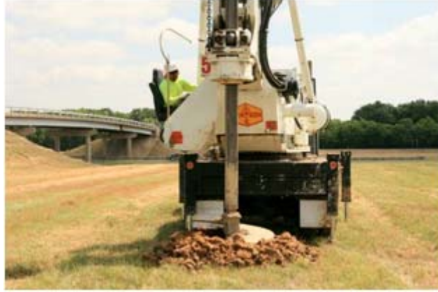
Figure 4.8. Drilling of Reaction Shaft Holes.
