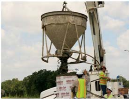
(a) Pouring Concrete in Sonotubes
