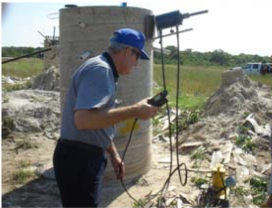
(a) Applying Tensioning Loads
