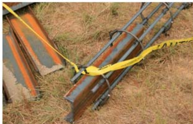
Figure 4.9. Channel Steel Tied to Steel Rebar Cage.
