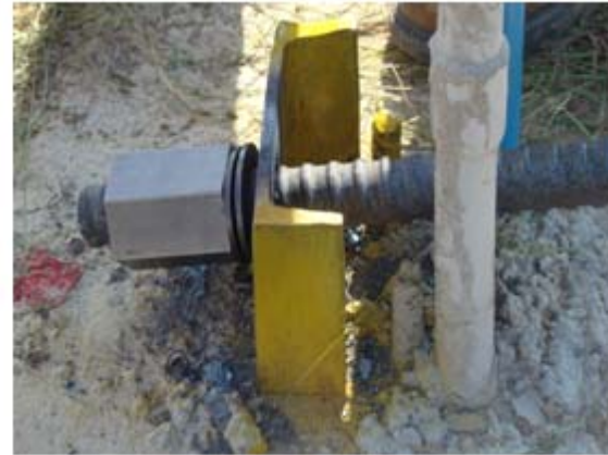
(b) Retaining Nut Attached to Test Shaft Steel Channel
