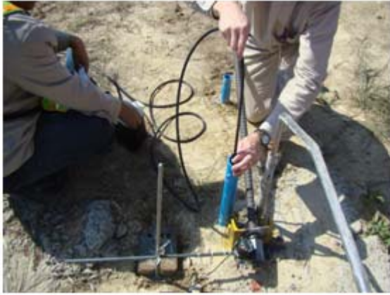
(a) Test Shaft
