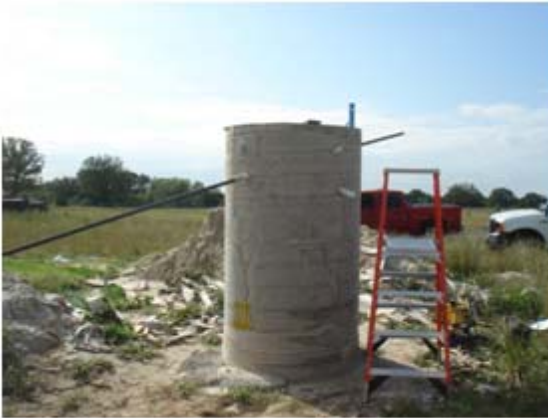
(a) Dywidag Bar in Place for Testing
