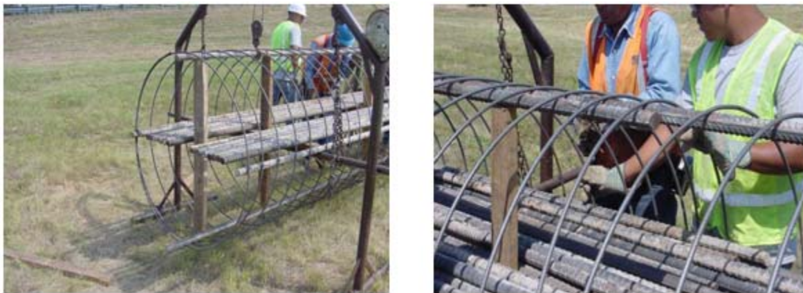
Figure 4.5. Construction of the First Reaction Shaft Rebar Cage.
