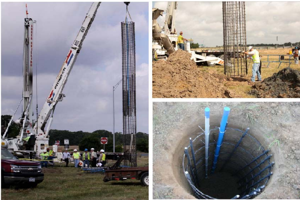
Figure 4.10. Setting the Steel Rebar Cages.
