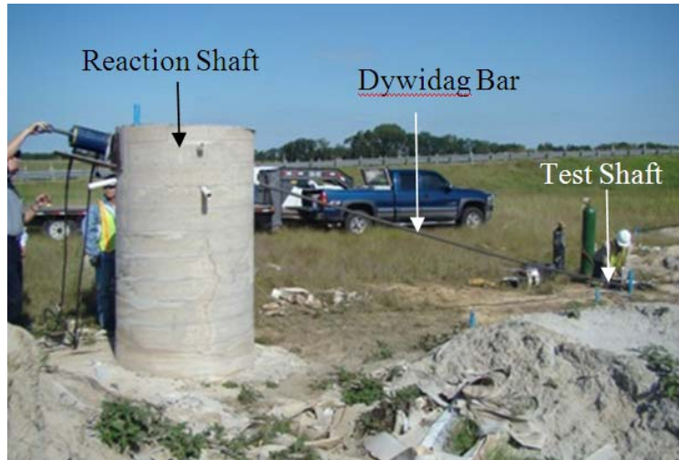
Figure A.2. View of a Reaction Shaft with Inclined Dywidag Bar.
