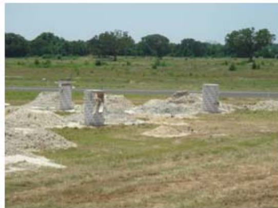
(b) Final View of Test Setup Area
