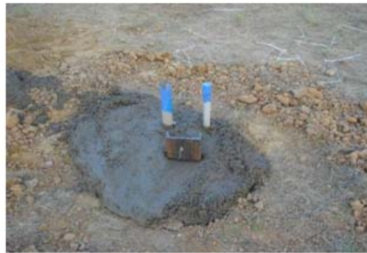
Figure 4.11. Pouring Concrete and Final Shaft.
