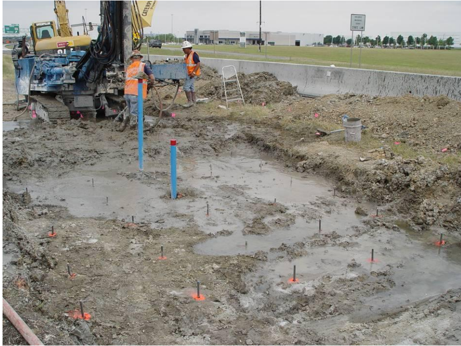
Figure 5.26 Field schematic of placing inclinometer into DSM column
