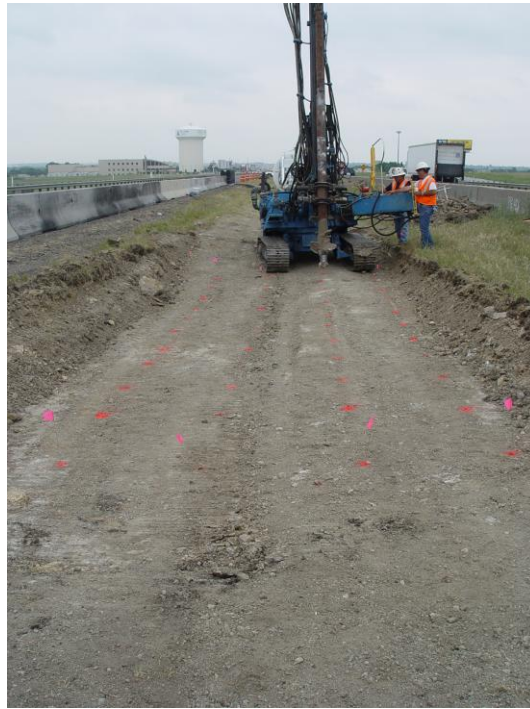
Figure 5.13 Test section at Site 1 prepared for DSM column installation
