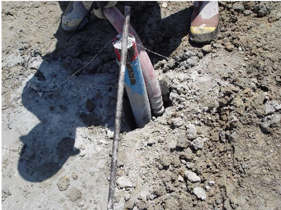
Figure 5.27 Field schematic of inclinometer anchoring and grouting
