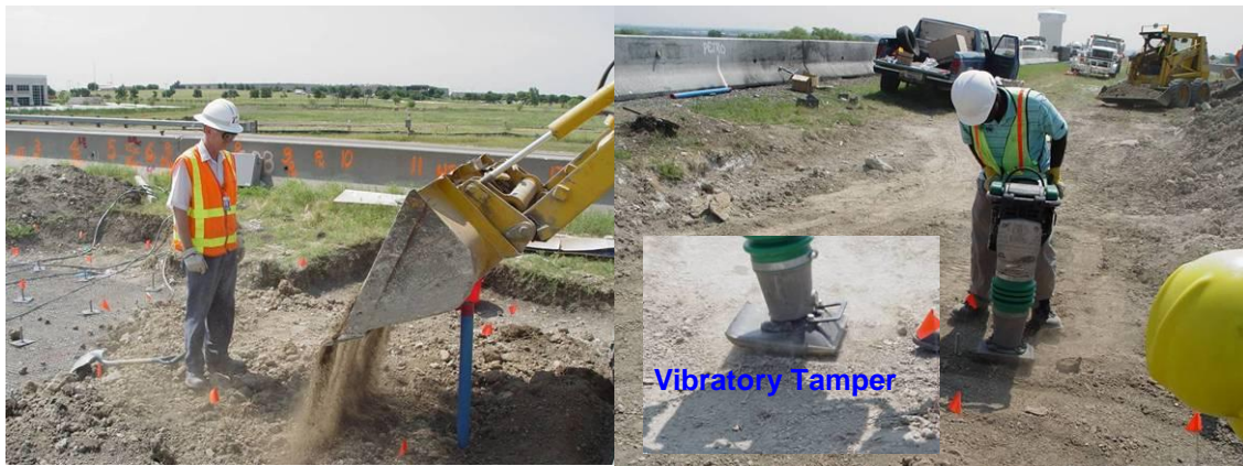
Figure 5.20 Fill placement and compaction using a vibratory tamper
