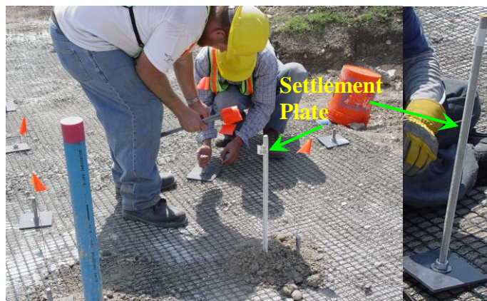
Figure 5.34 Settlement plate and its placement
