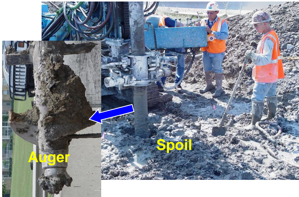
Figure 5.15 Field schematic of soil-binder mixing process and mixing auger
