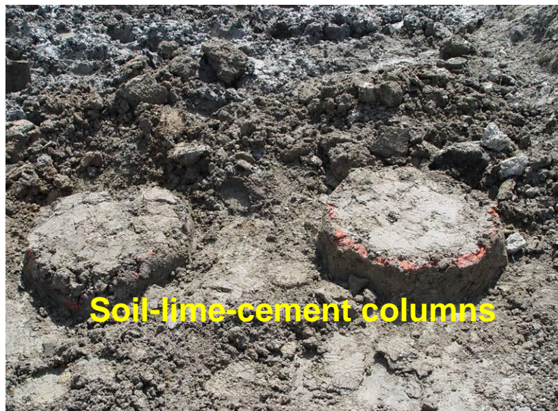
Figure 5.16 Soil-binder columns formed at the end of in-situ mixing
