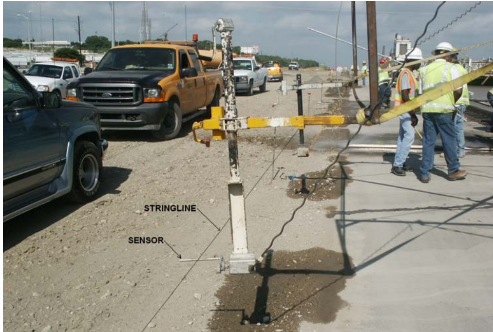
Figure 2-4. Stringline Set-Up on a Concrete Paving Project.
