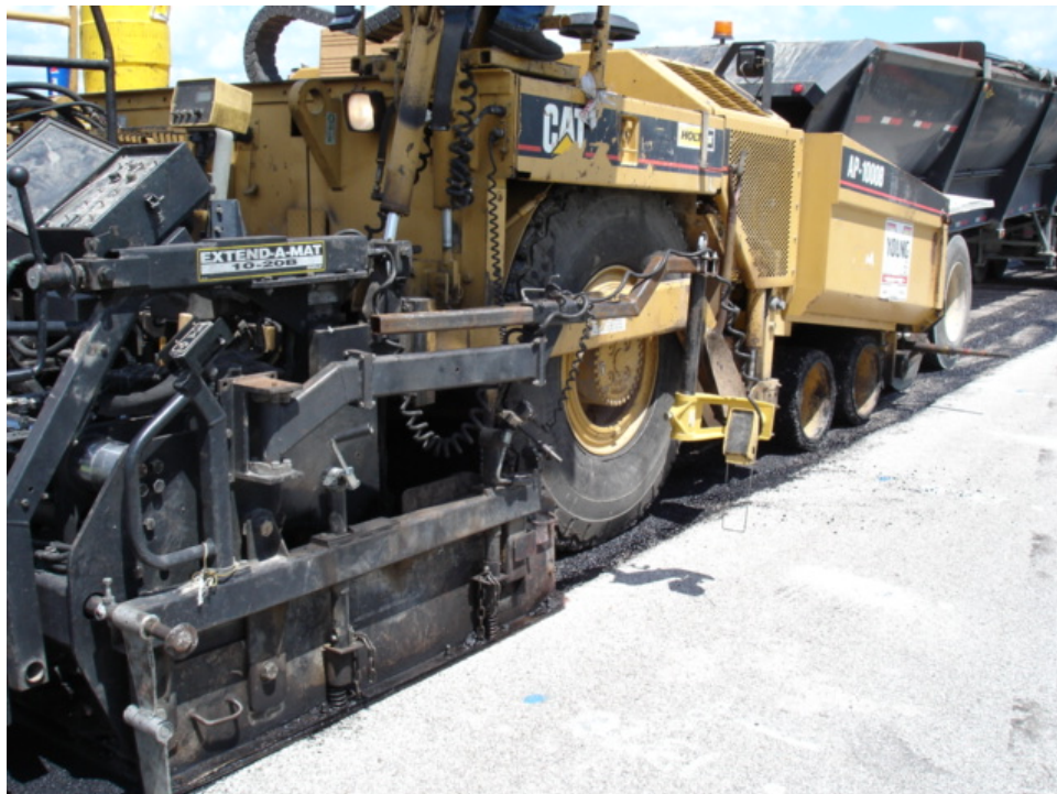
Figure 2-5. Picture of Paver Used to Overlay Test Section.
