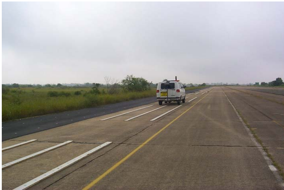
Figure 1-2. Rut Calibration Section.
