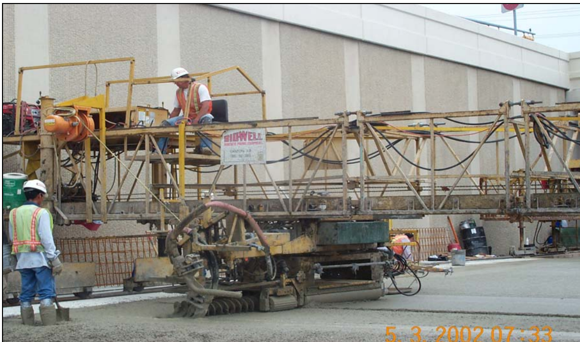
Figure 10. Bidwell Paving Machine Used in San Antonio Project.
