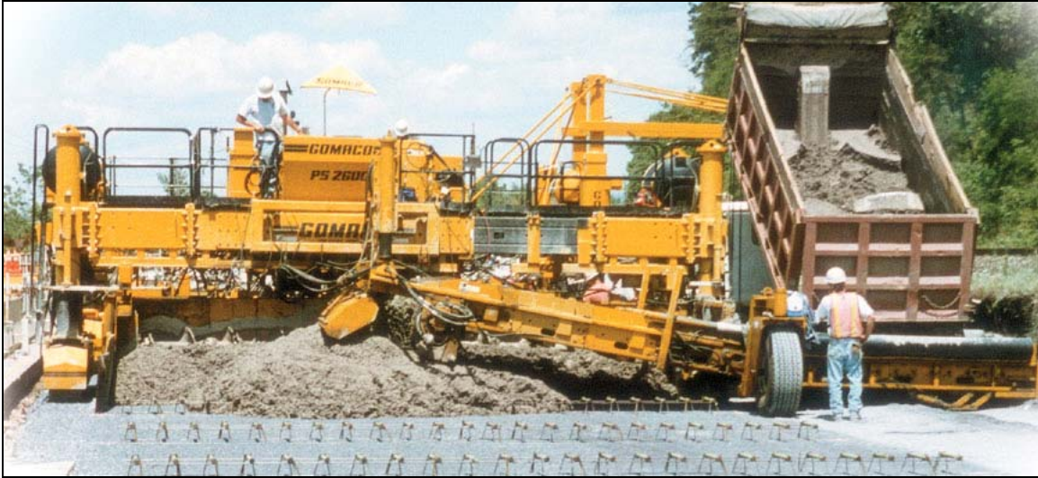
Figure 1. Placer Spreader.
