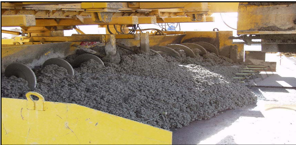
Figure 2. Close-up View of Spreader Showing Auger.
