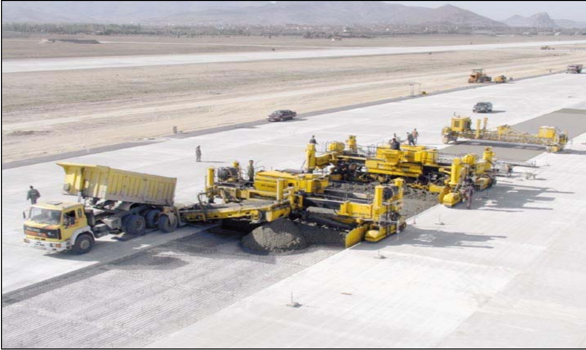
Figure 6. Illustration of Paving Train.
