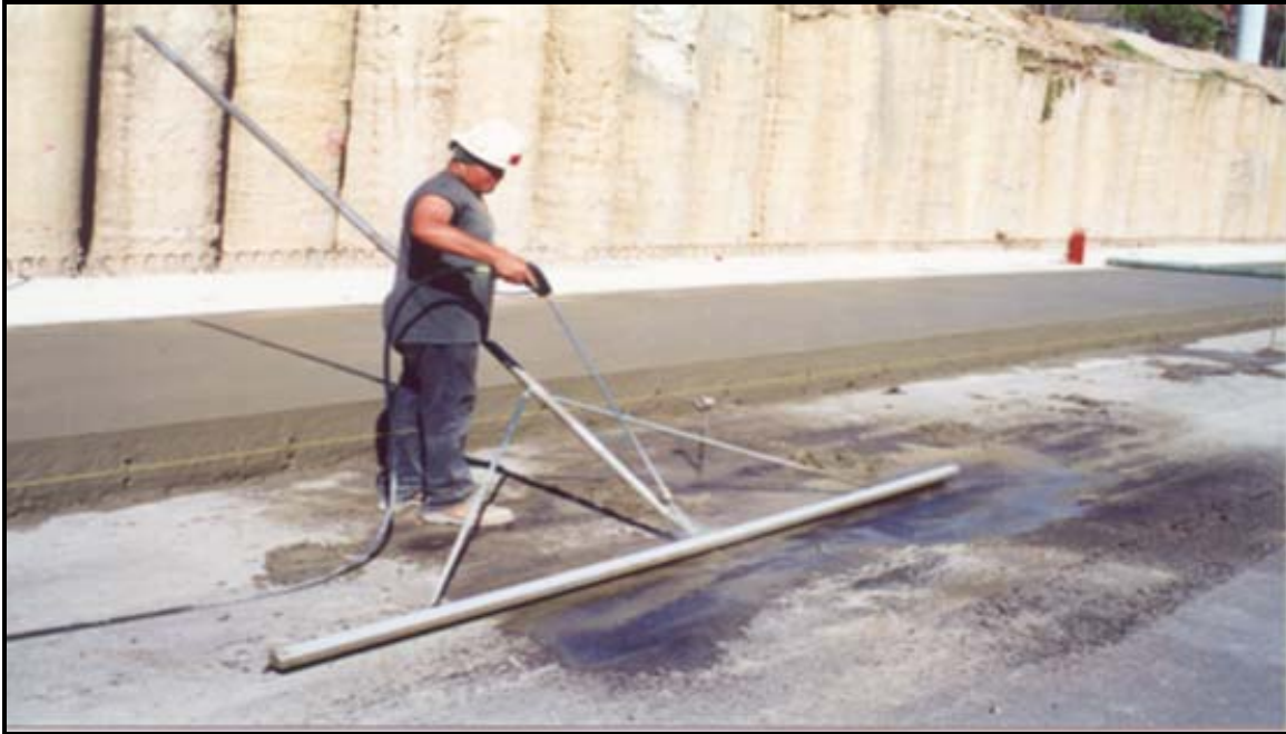
Figure 5. Straightedge Used for Hand Finishing.
