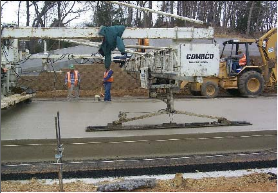
Figure 3.1. Autofloat Attached to Paver.
