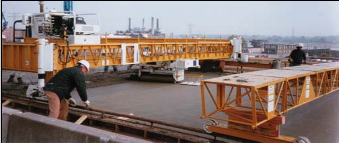
Figure 9. Mechanical Finisher for Bridge Decks.
