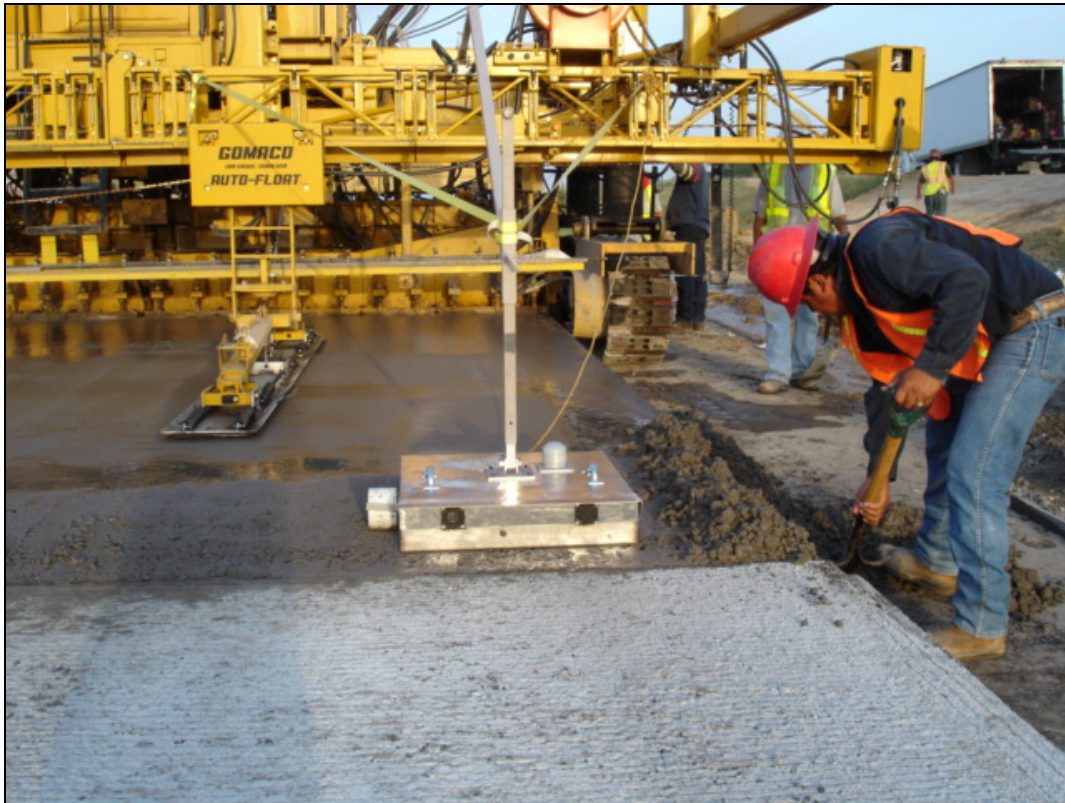
Figure 3.11. Photo of Sliding Profiler Taken Just after Crossing the Header Joint.
