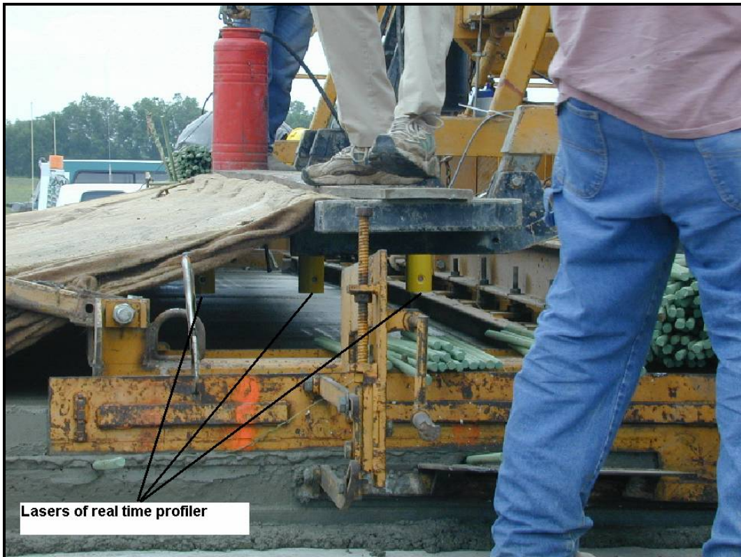
Figure 12. Real Time Profiler Developed by Ames Engineering.
