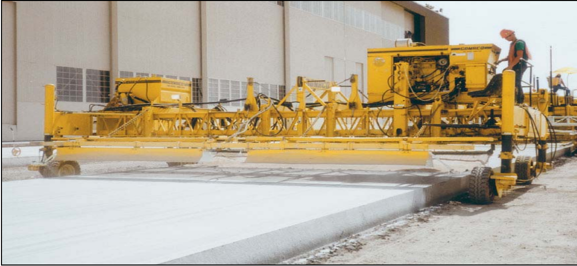
Figure 11. Texture and Curing Equipment.
