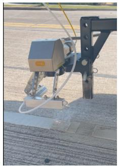
Figure 1. Laser system in operation: white thermo stripe removal from a concrete surface. Firstly, a literature review and a national survey were conducted to understand the current stateof-the-art and industry standards regarding the removal of road stripes. The survey was prepared and disseminated to various DOT districts from different states.
