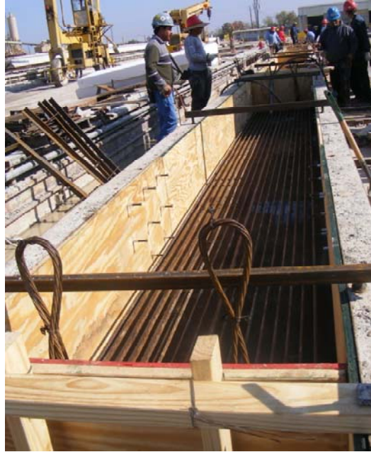
Fig. 8.2 Details of PSFC Box-Beam Before Casting.
