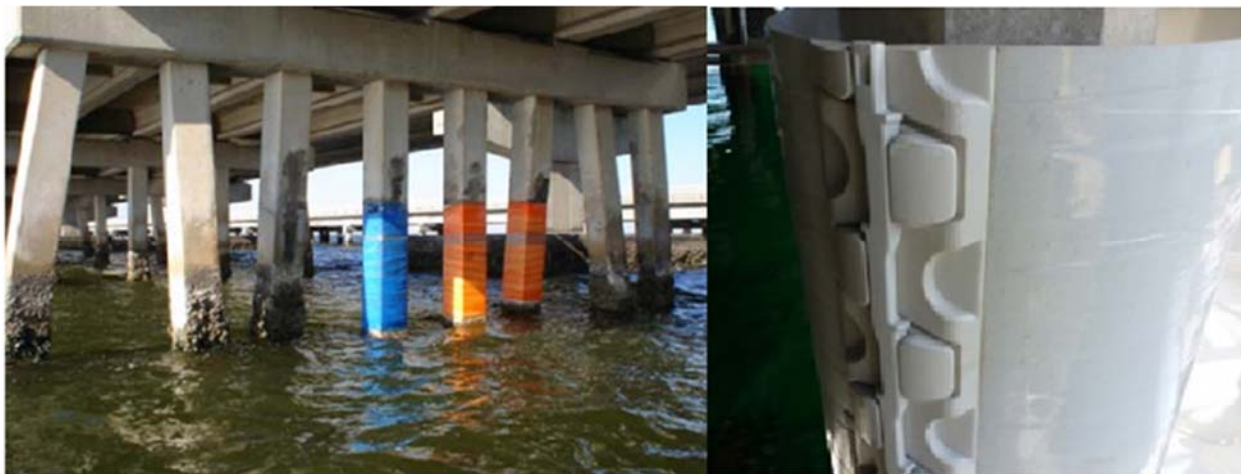
Figure 5. FRP Wrapping Retrofit (left), Plastic Pile Jacket (right).
