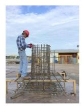
(a) Drilled shaft and base rebar cage
