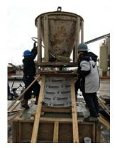
(c) Drilled shaft and base casting
