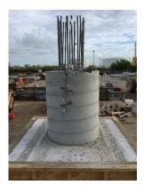
(e) Drilled shaft and base- after casting
